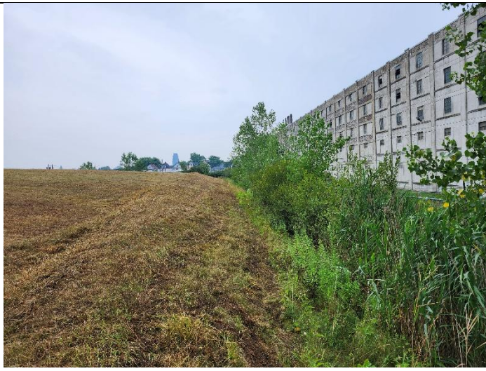
View of east portion of Site and drainage swale
