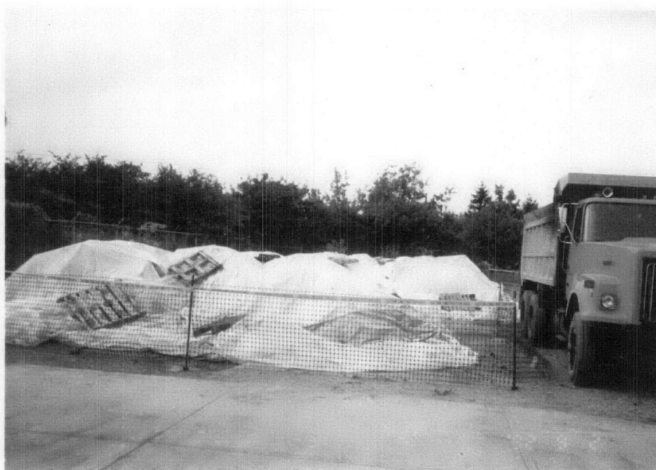
SOIL STOCKPILE AREA COVERED AND PROTECTED
