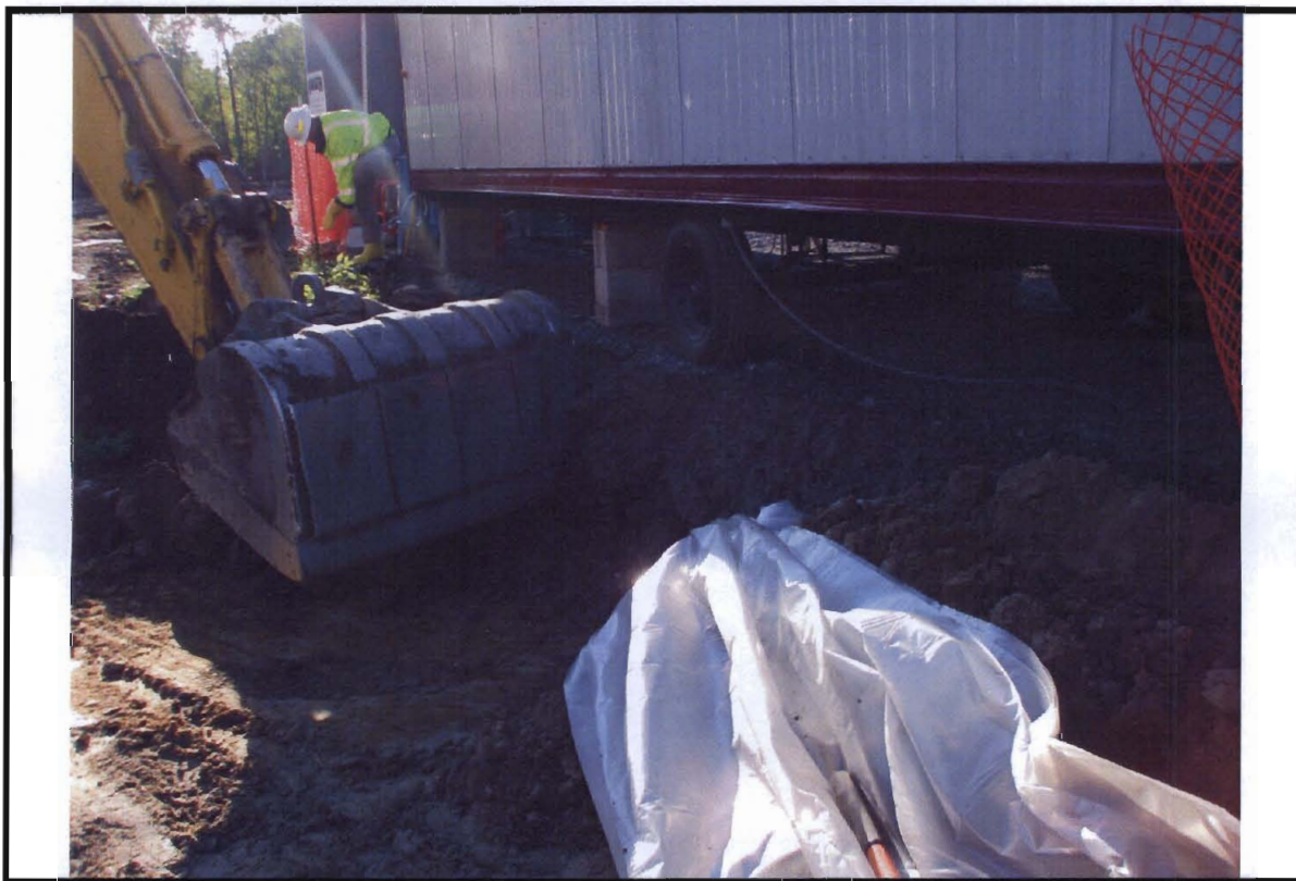
Photograph 20. Excavation of the contaminated waste layer north of access road and site construction trailer.
