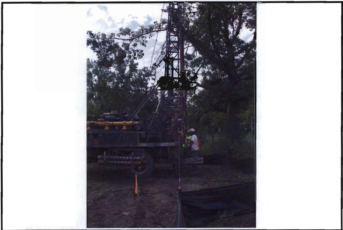
Photograph 18. Monitoring well installation in the southwestern portion of the property (MW5A-07).
