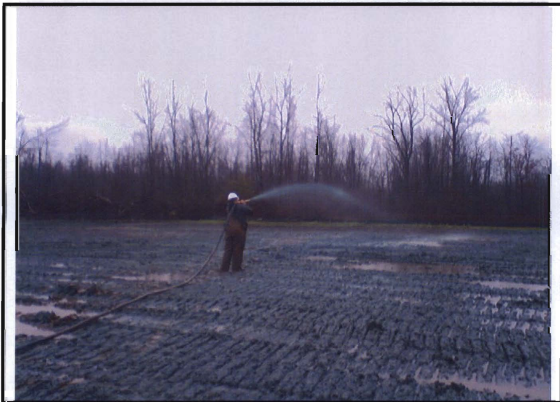
Photograph 30. Hydro-seeding of the property after final grading.
