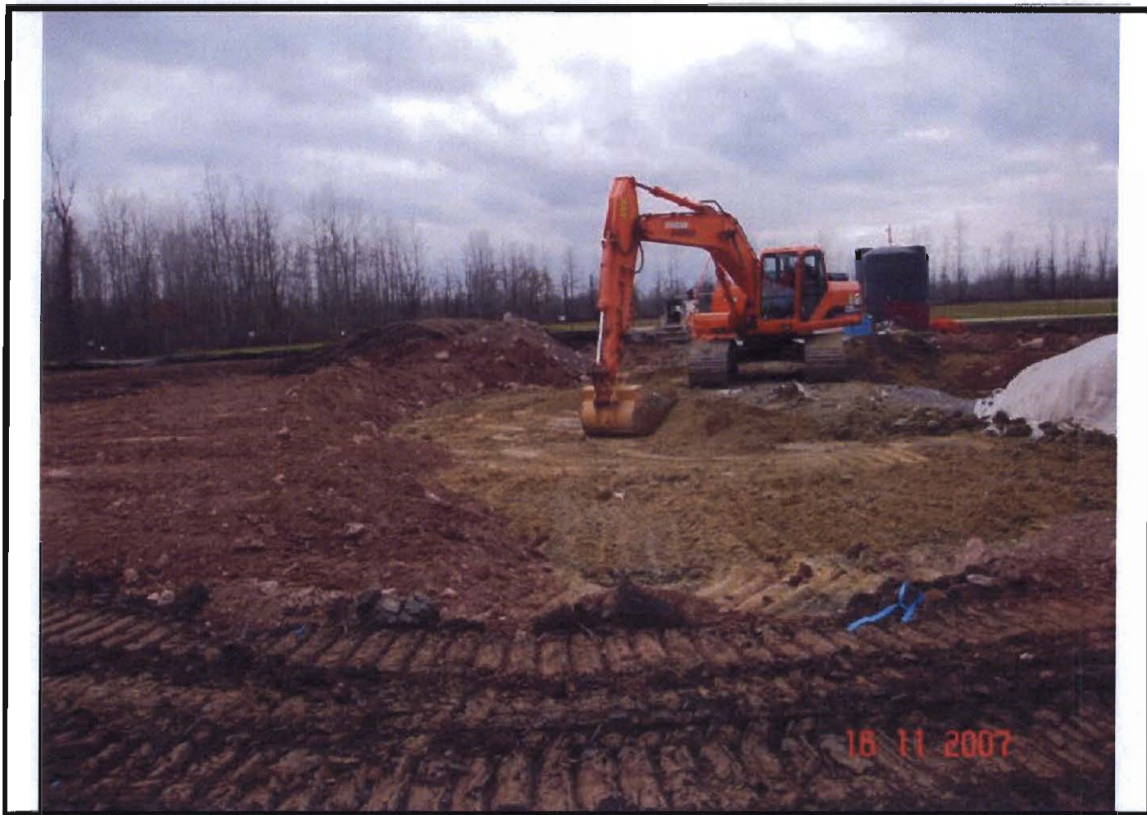
Photograph 27. Final grading of top soil before hydro-seeding can begin.
