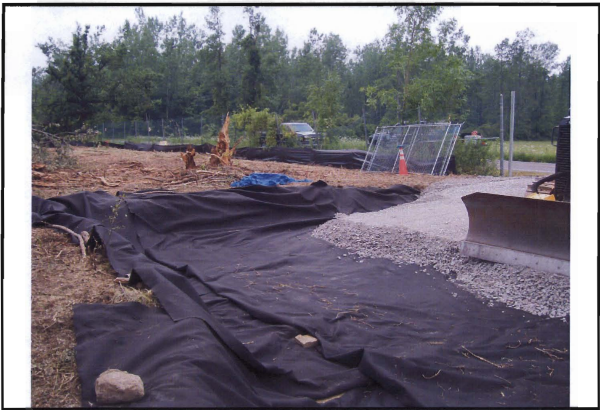
Photograph 3. Construction of the access road and decontamination pad.
