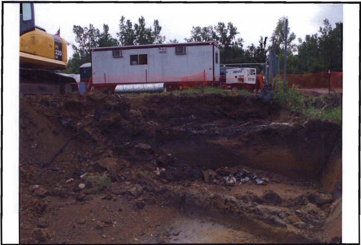
Photograph 17. Excavation of the contaminated waste layer, near Fletcher Road. Paint waste and debris are visible.
