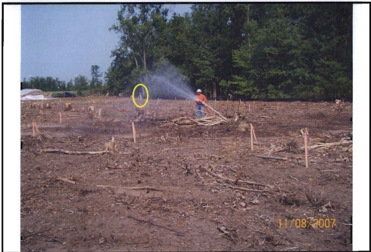
Photograph 5. Dust control conducted during excavation activities with air monitor in the background.
