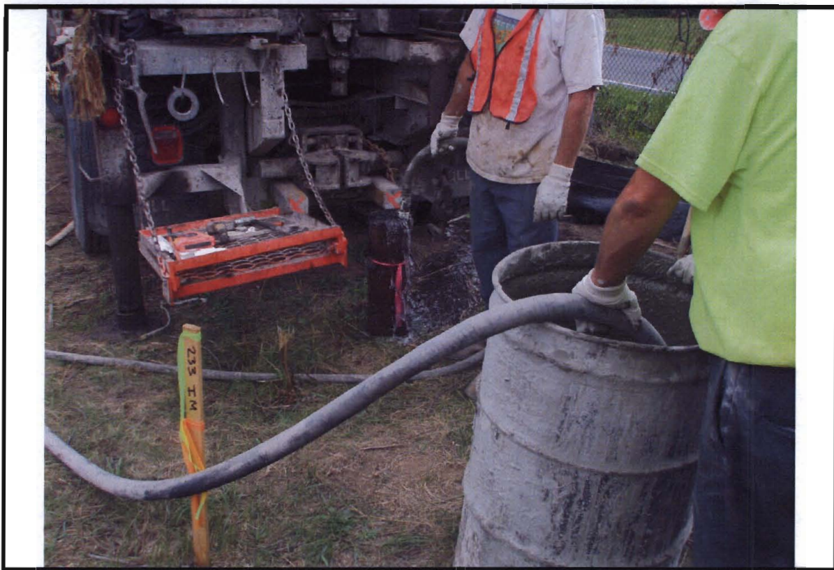
Photograph 19. Well decommissioning of the on-site water supply wells.
