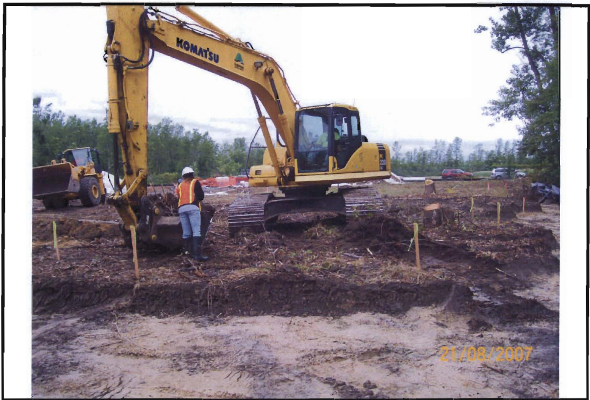
Photograph 9. PID readings taken from the excavator bucket during soil removal.
