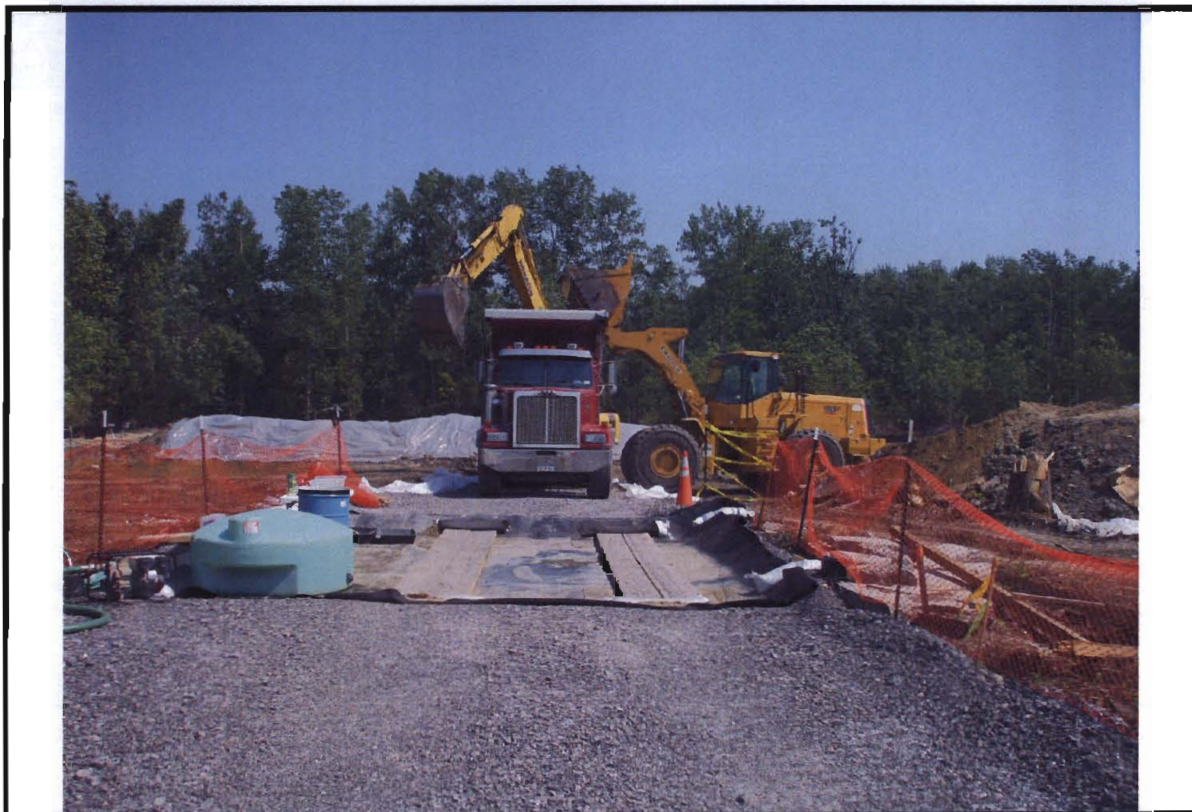
Photograph 15. Off loading of the staged soil. Decon pad and access road in foreground.
