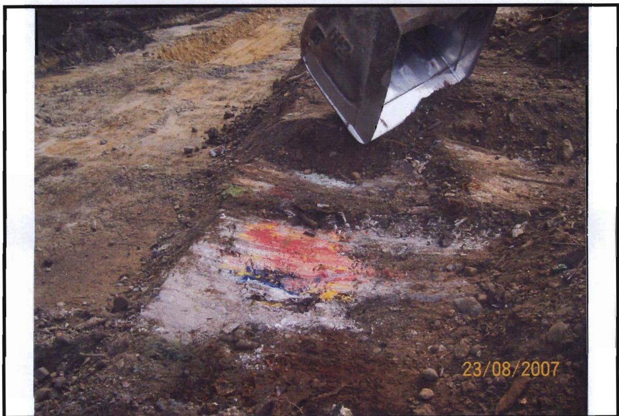
Photograph 14. Visible paint waste in the northwest corner of the contaminated waste layer.
