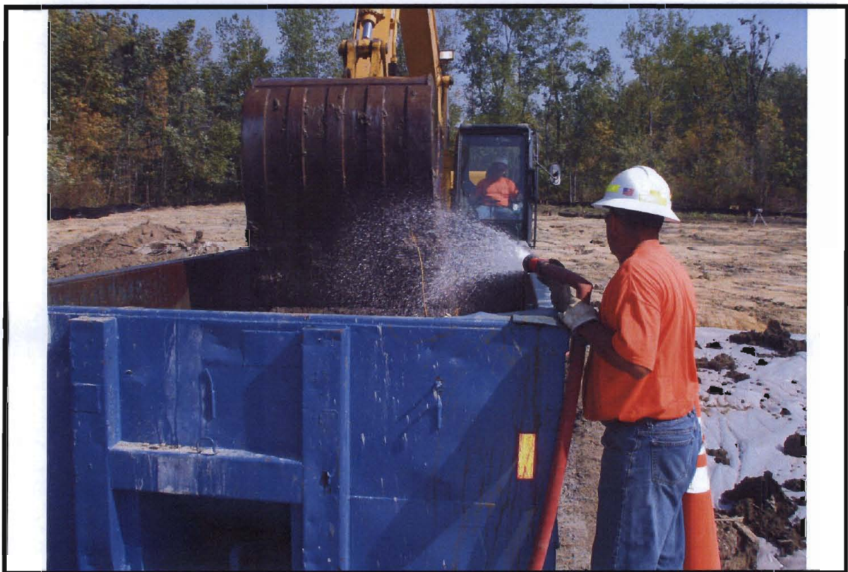
Photograph 24. Stabilization of the hazardous soil excavated from the northern wall face.
