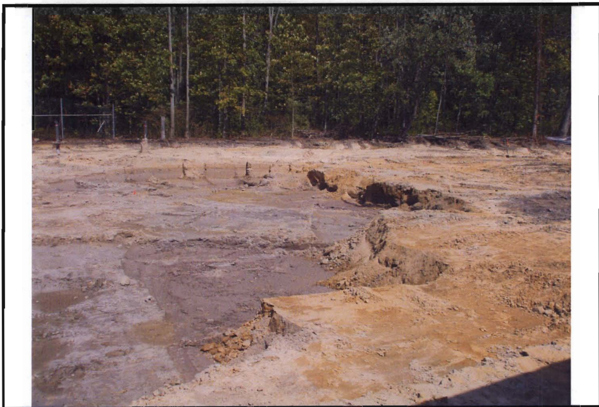
Photograph 21. Finished excavation of the contaminated waste layer.
