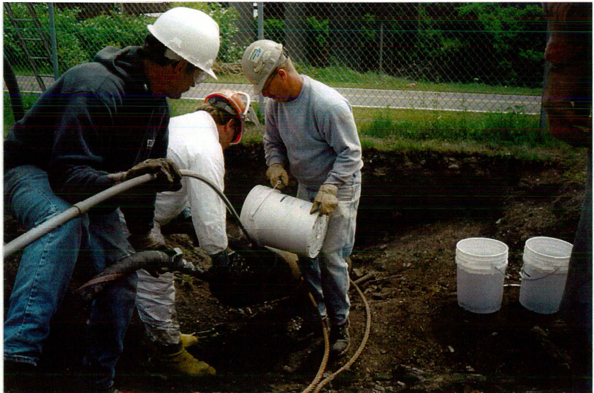
2B. Installing well materials.
