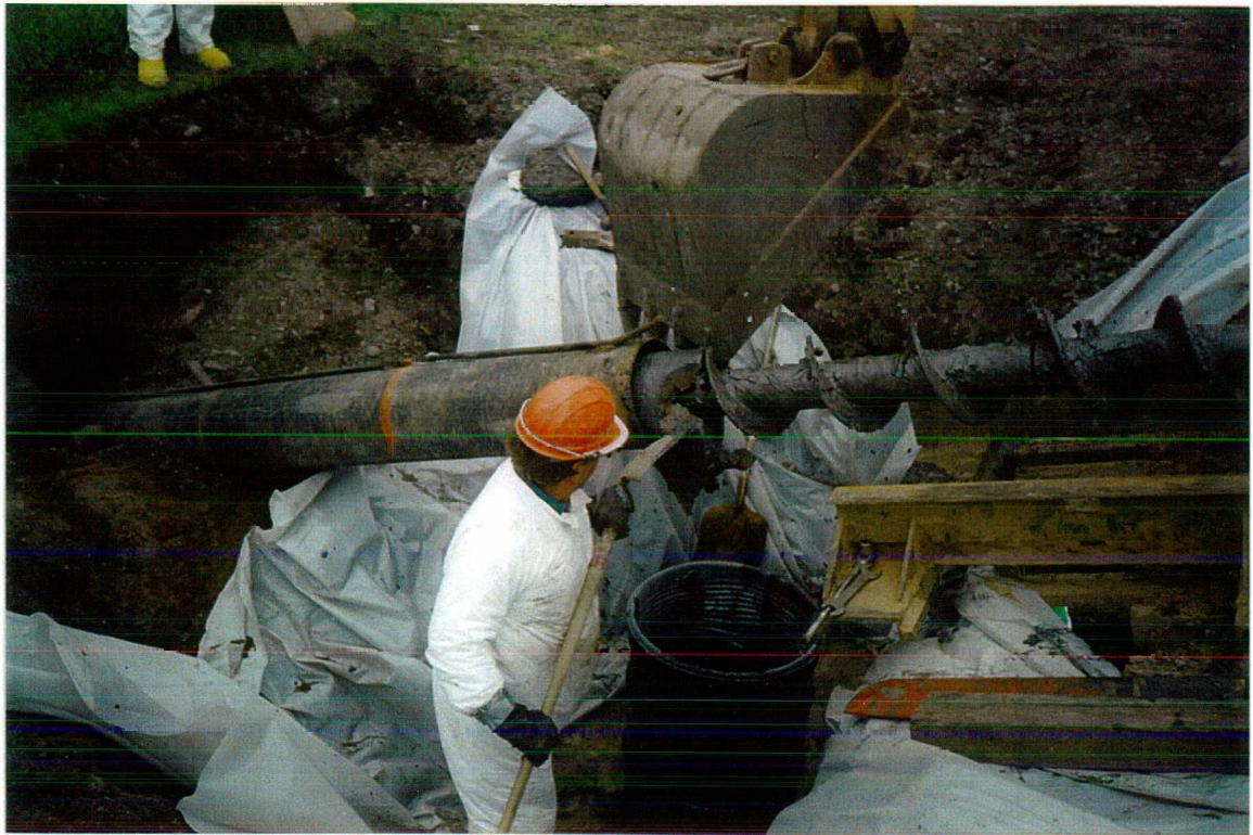
2A. Containerizing drill cuttings.
