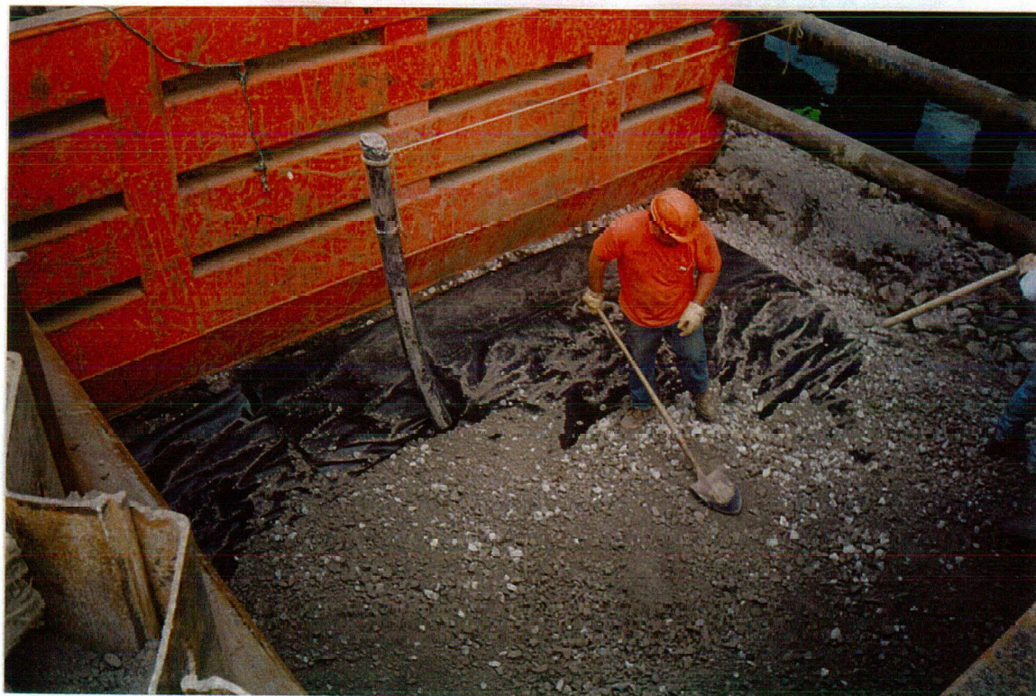
4B. Placing vault sub-base.
