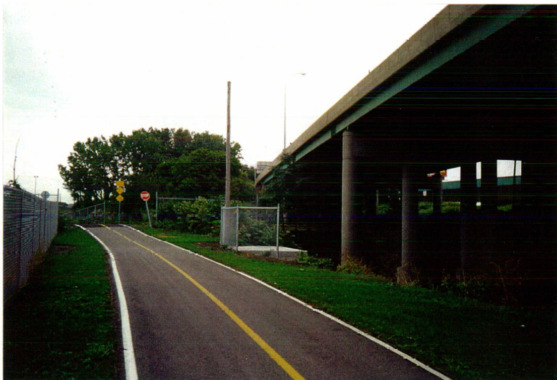
6B. Completed system (from south).
