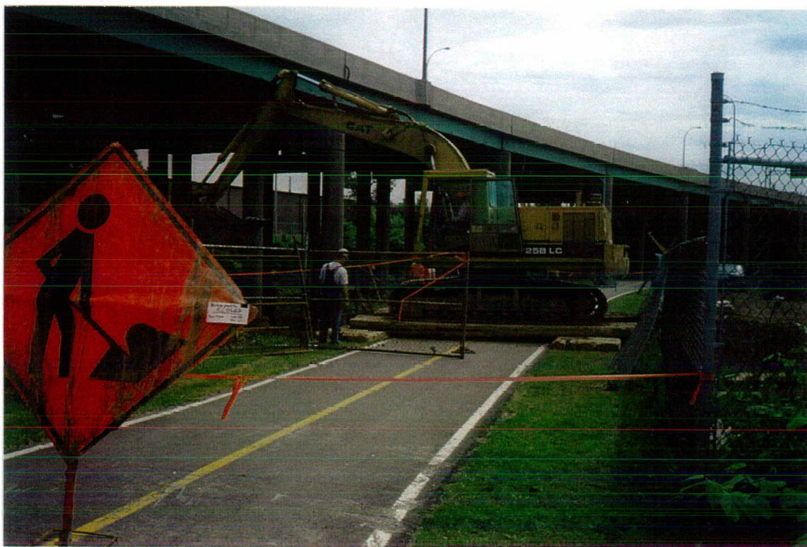
3A. Preparing for vault excavation.
