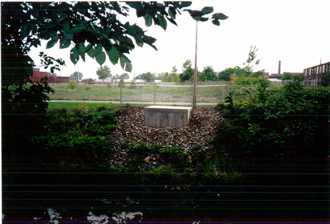
6A. Completed system (from east).
