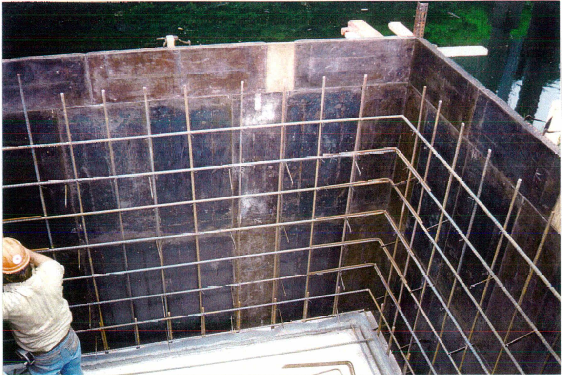
5A. Constructing vault form work.
