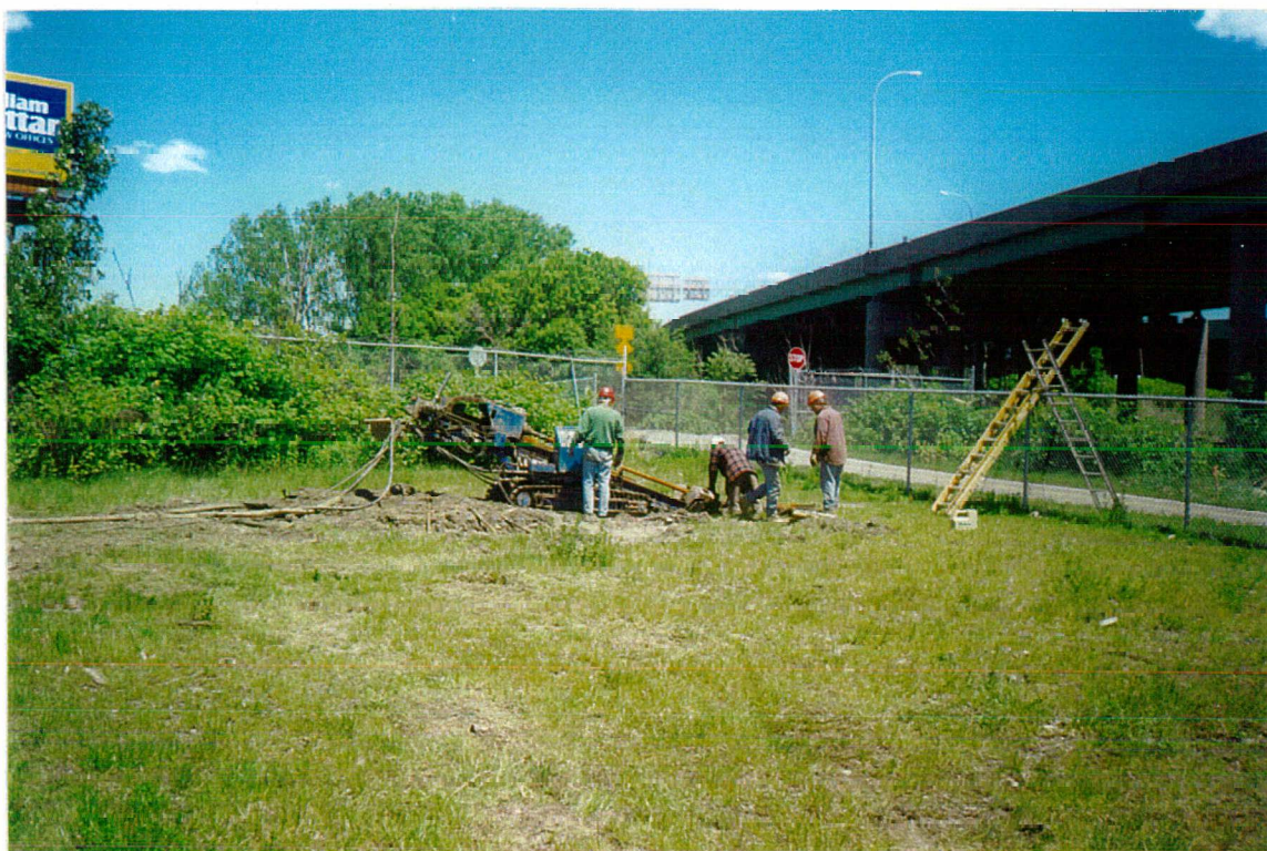
1A. Directional drilling to target area.
