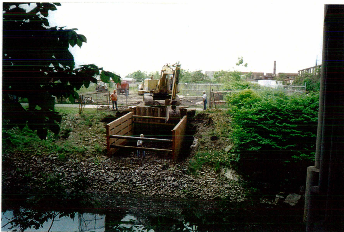
3B. Vault Excavation
