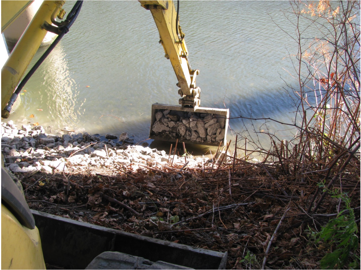
Placement of stone at Area 8.
