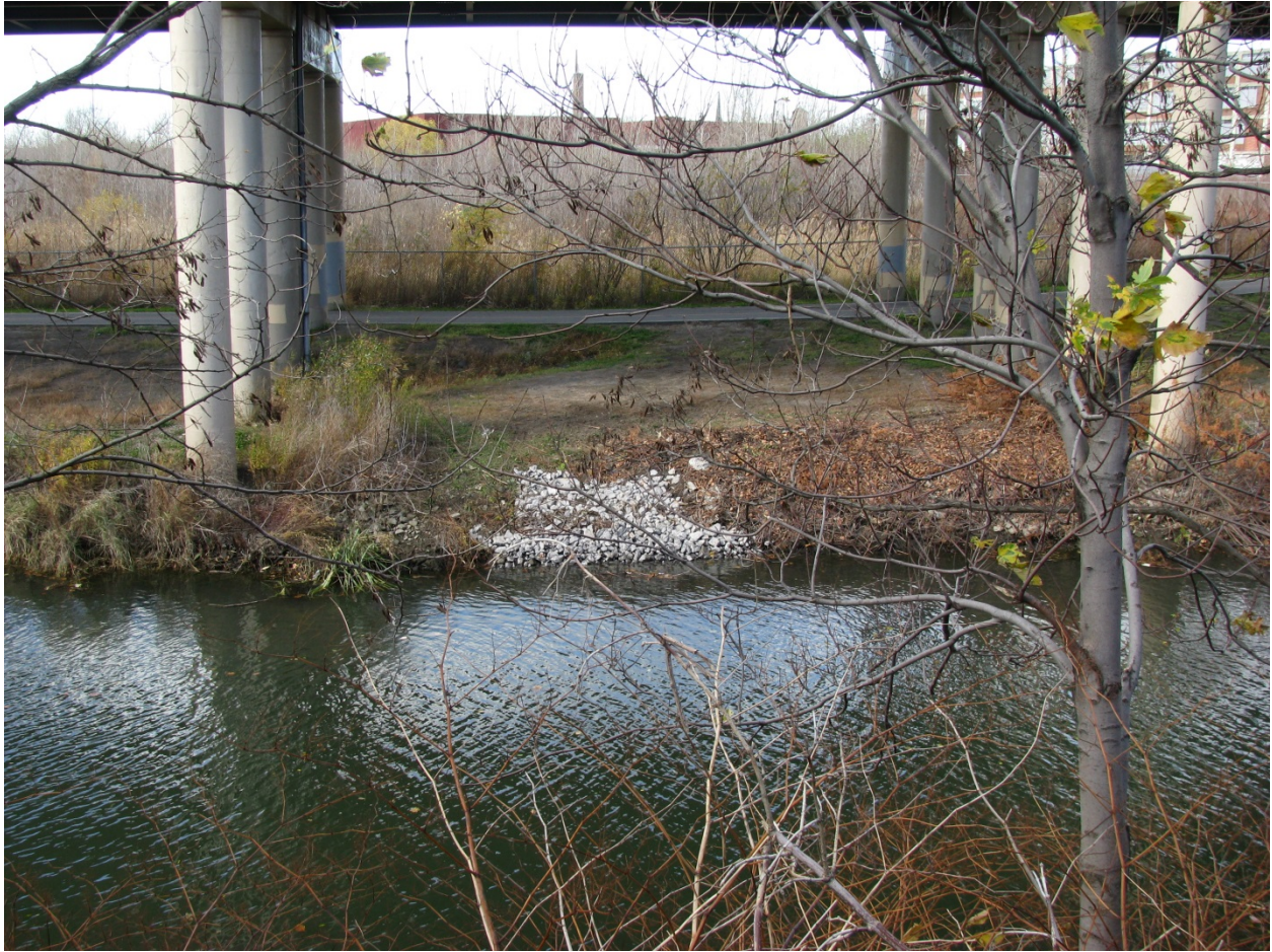
Completed maintenance activity at Area 7.
