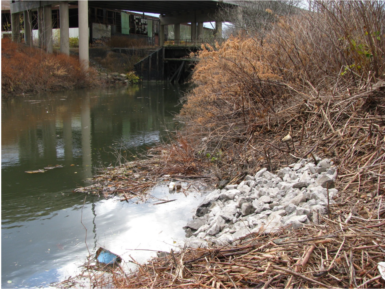
Completed maintenance activity at Area 6.
