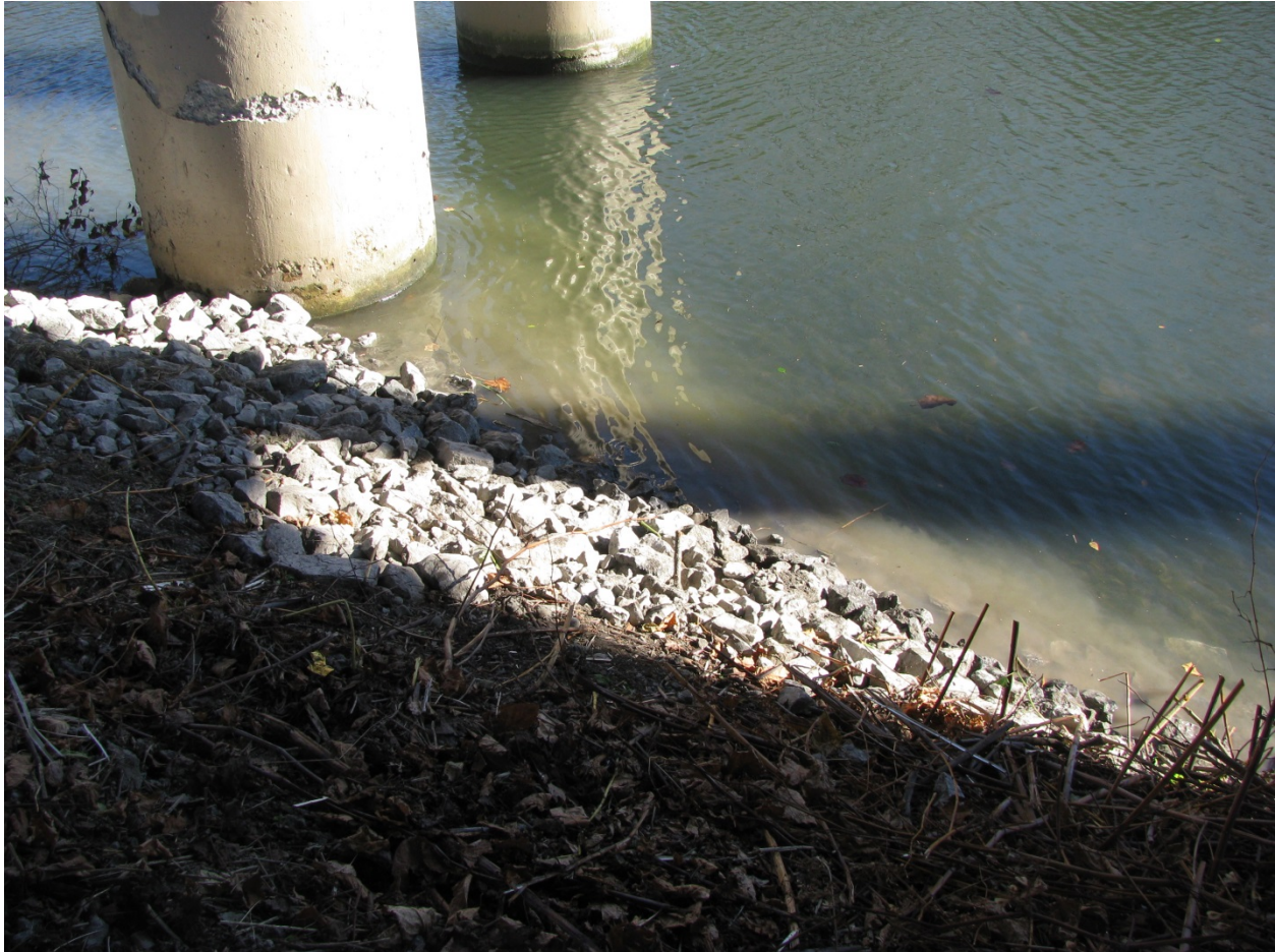
Completed maintenance activity at Area 8.
