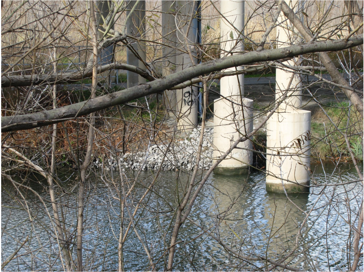
Completed maintenance activity at Area 8.
