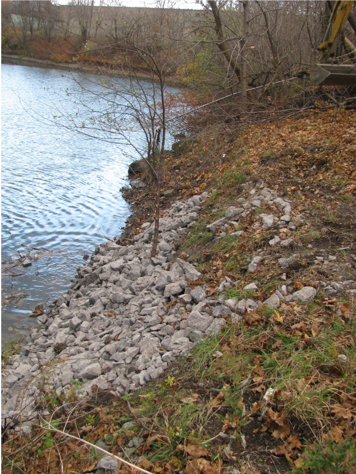
Partially completed maintenance activity at Area 2.
