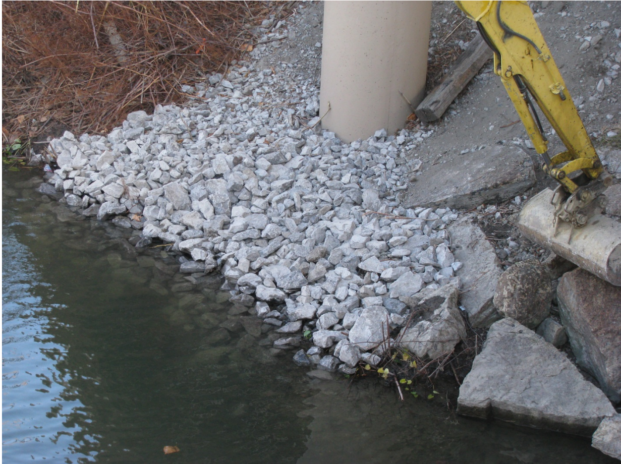
Completed maintenance activity at Area 5.
