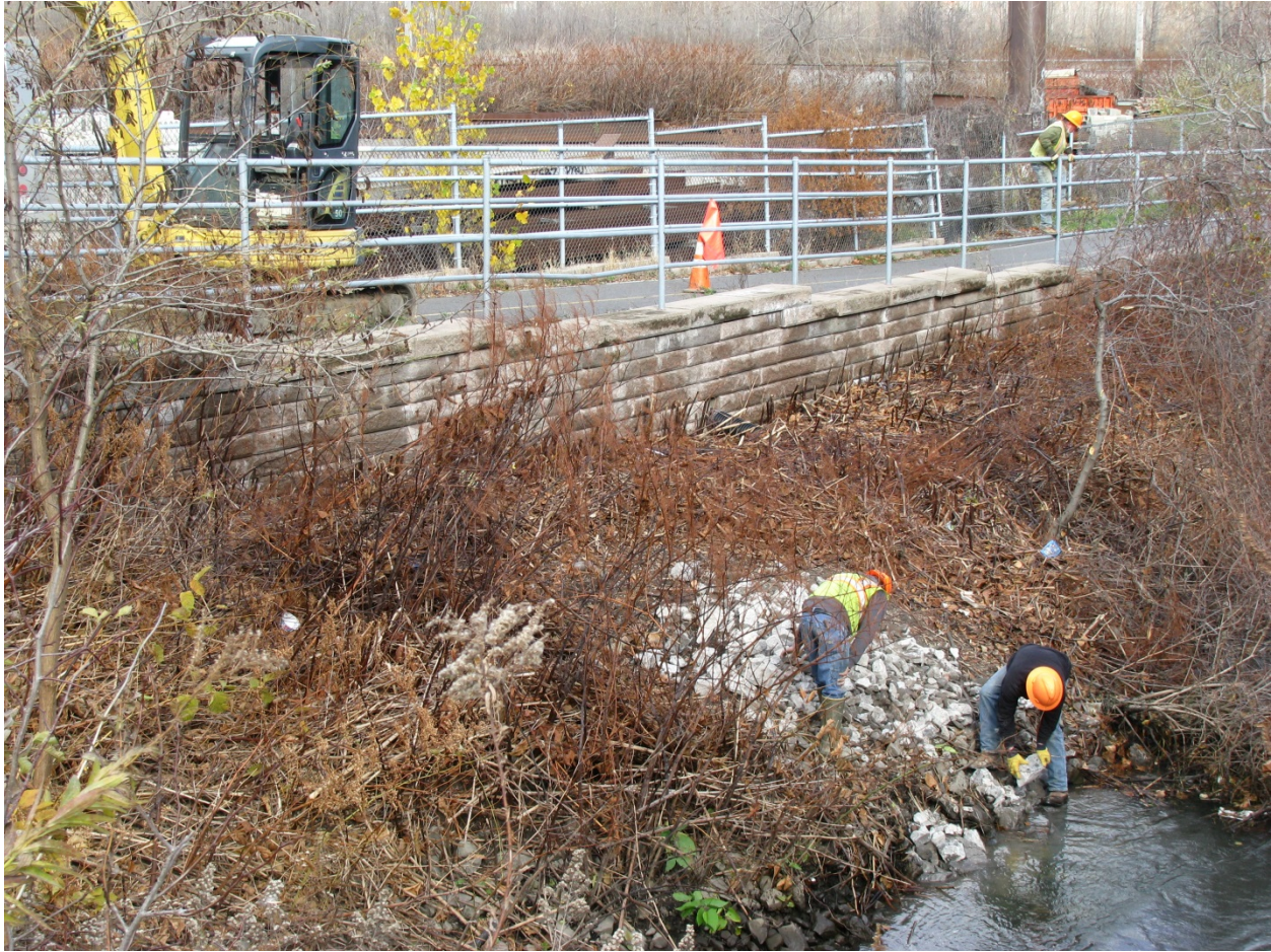
Performing maintenance activity of Area 1.
