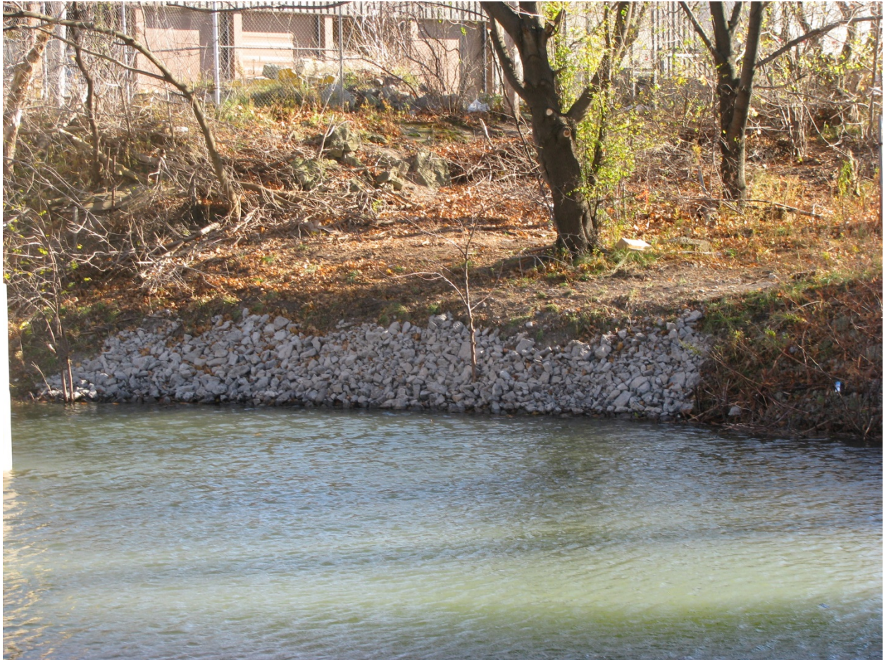
Completed maintenance activity at Area 2.
