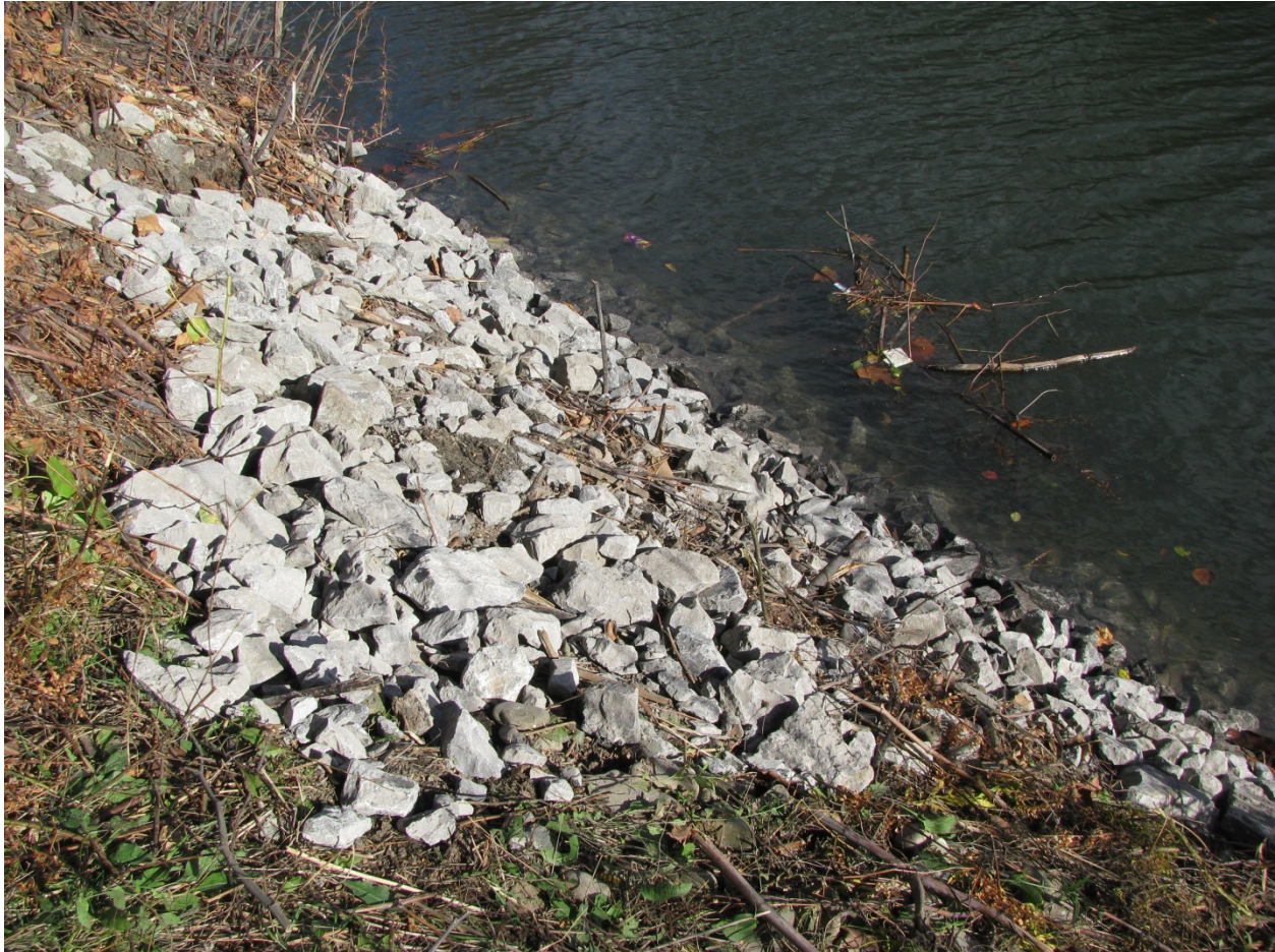
Completed maintenance activity at Area 7.
