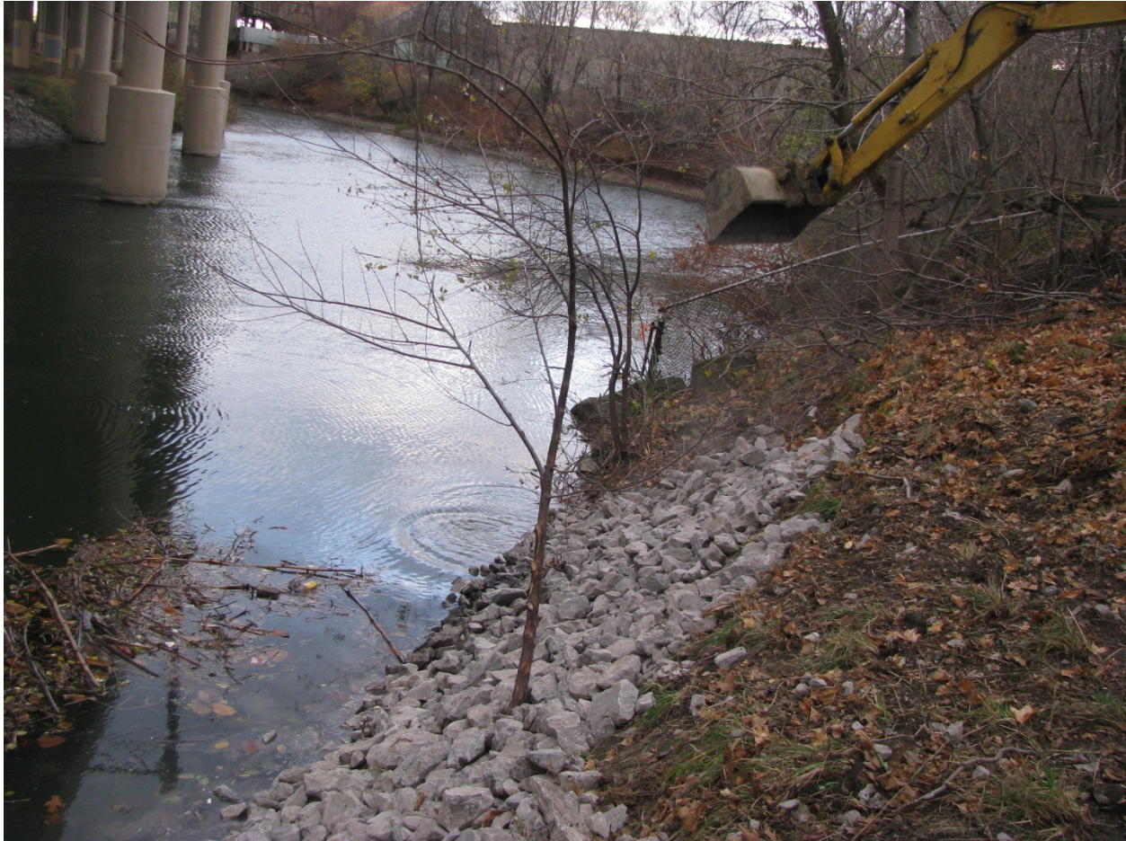
Partially completed maintenance activity at Area 2.
