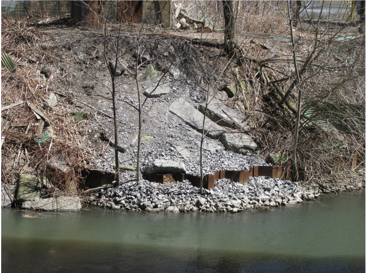
Looking east (across the Creek) at 2015 Maintenance Area 4. Though no vegetation has yet established itself on the slope above the maintenance area, there are no signs of erosion.
