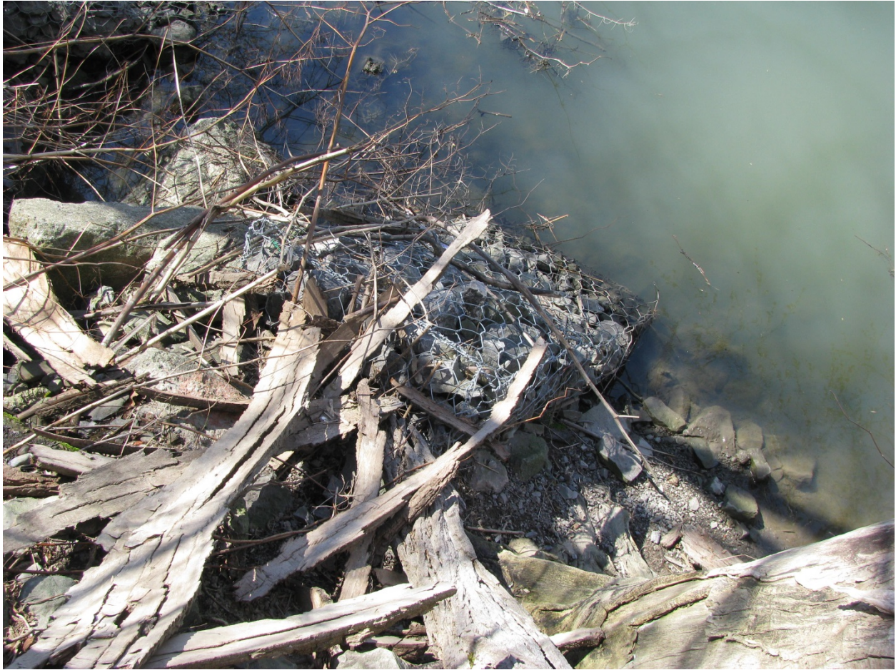
Looking downslope (west) at the gabion baskets at the outlet to the stormwater discharge pipe from the Westwood property, just south of the existing sheetpile wall. The gabions are in good shape.
