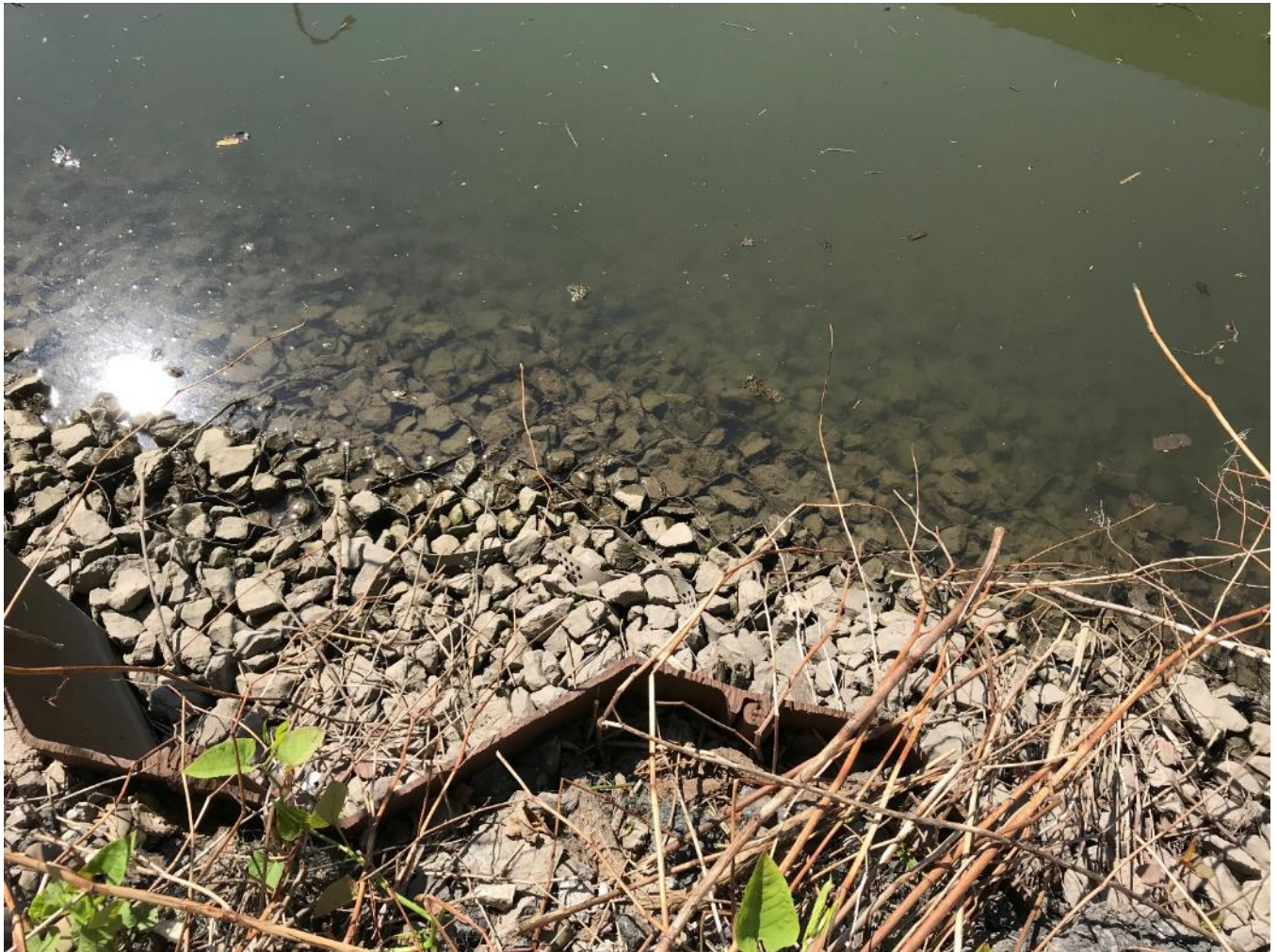
Photo 5. Top down closeup view of Maintenance Area 4 and sheet pile. Rip rap in good condition.
