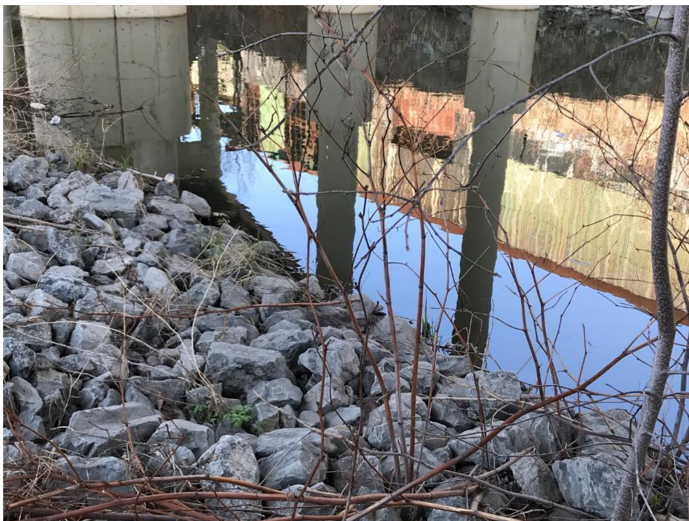
Photo 10. North view of west bank toward Conrail Bridge. No visible erosion.
