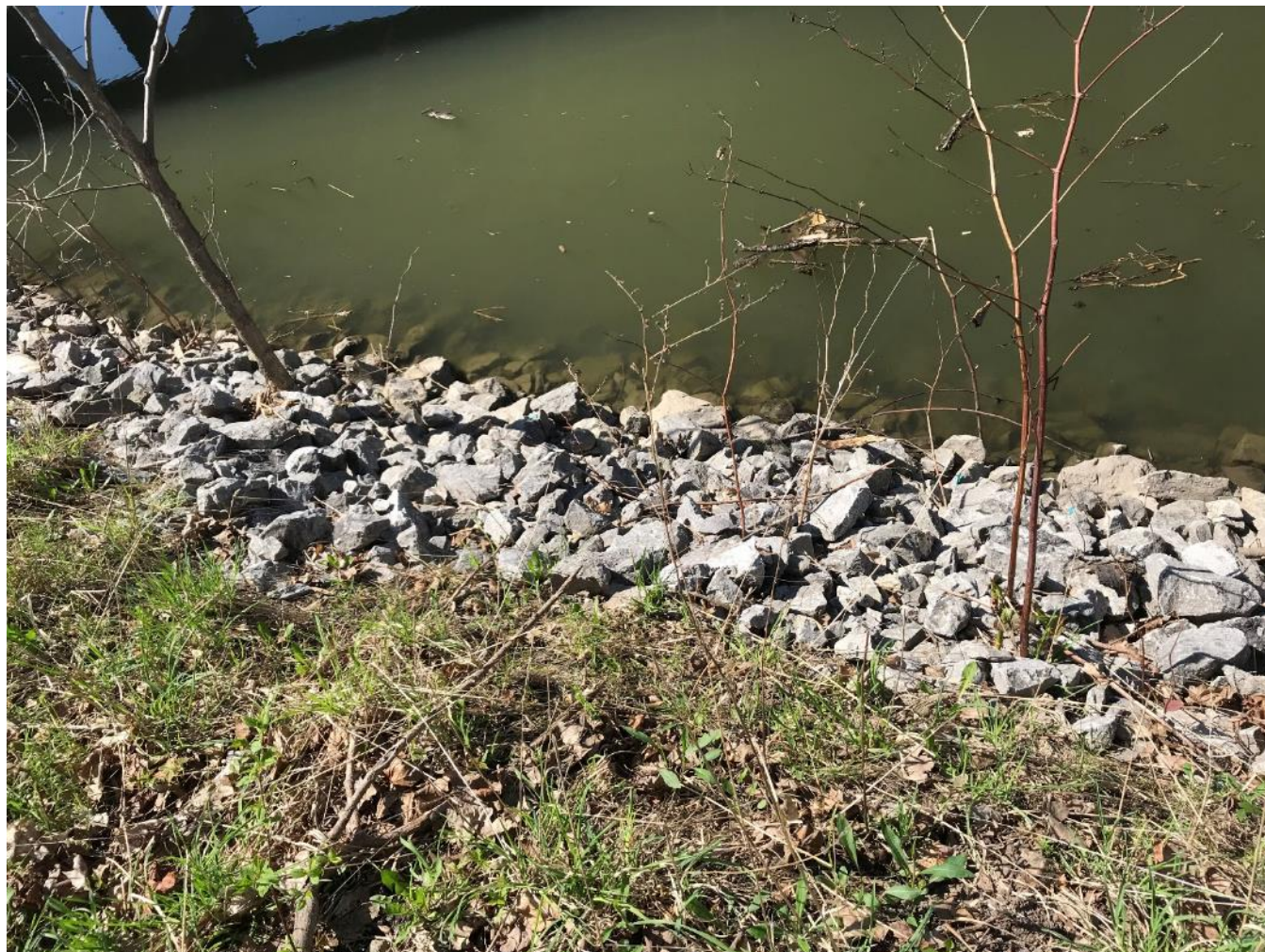
Photo 3. Downslope view on east bank of 2015 Maintenance Area 2. Rip rap in good condition.
