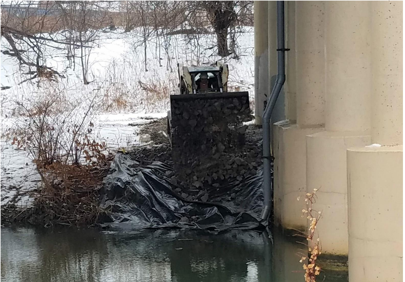
Photo 3. Placement of new armor limestone surge stone on new geotextile on February 10, 2020.
