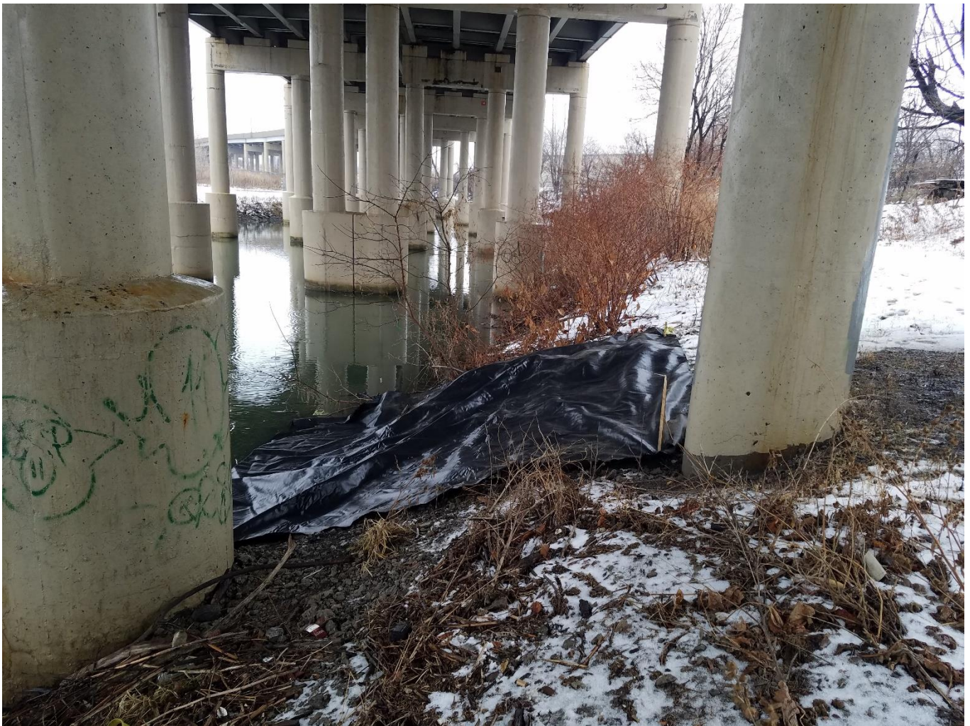
Photo 2. Layout of new geotextile fabric pinned to ground surface.
