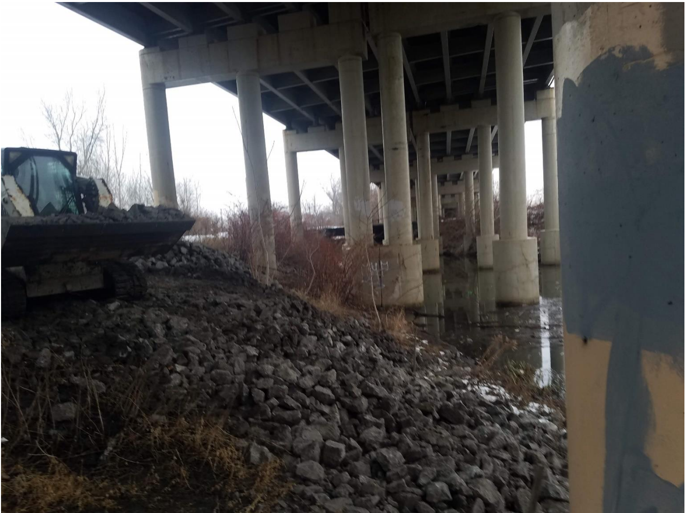
Photo 2. Placement of new armor limestone surge stone on new geotextile on February 11, 2020.
