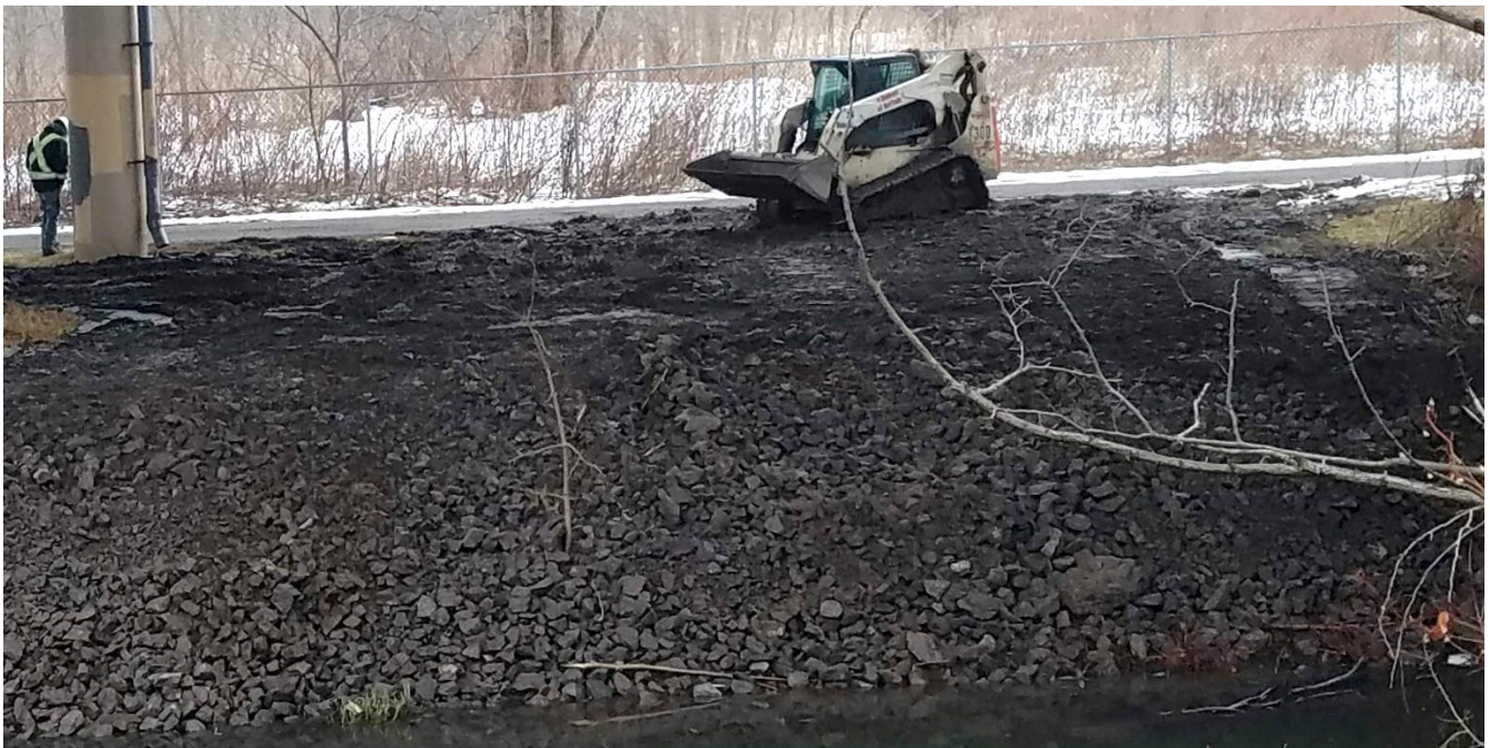
Photo 3. Placement of new armor surge stone at 2020 Maintenance Area 4 on February 11, 2020.
