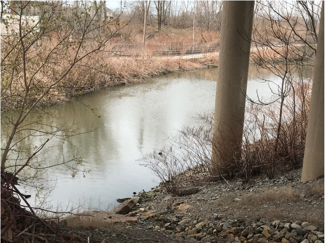
Photo 7. North view of Maintenance Area 5. No visible erosion. Rip rap and stone block in place.
