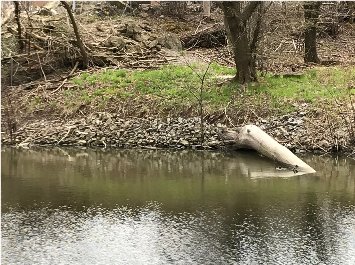
Photo 9. East bank view of 2015 Maintenance Area 2. No visible erosion.
