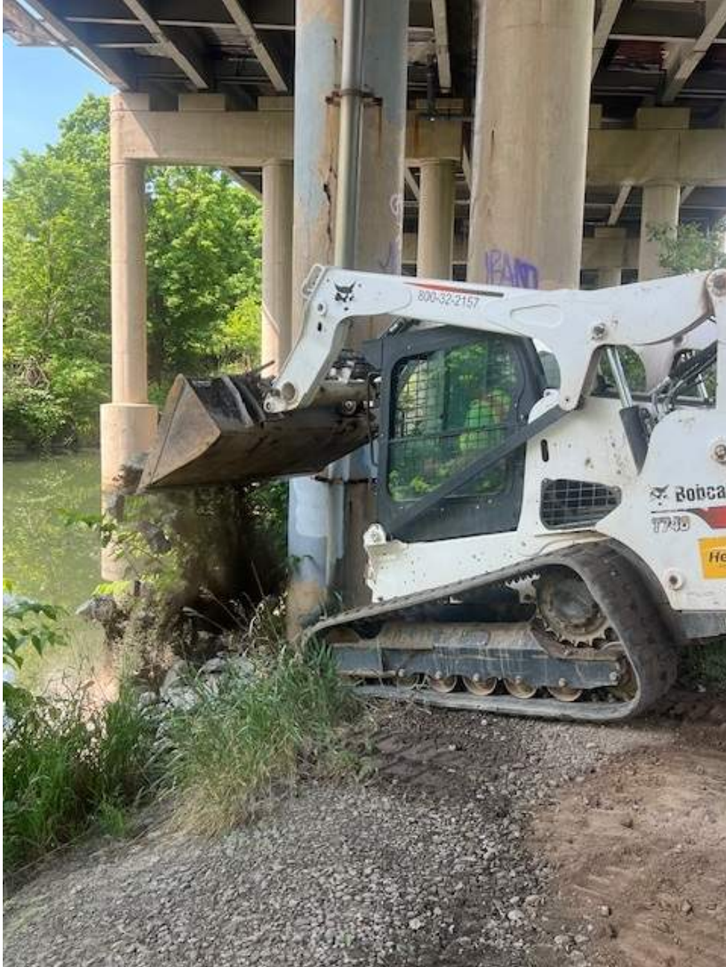
Photograph 2: Sun placing Light Stone Fill over Maintenance Area No. 7 (Looking south).
