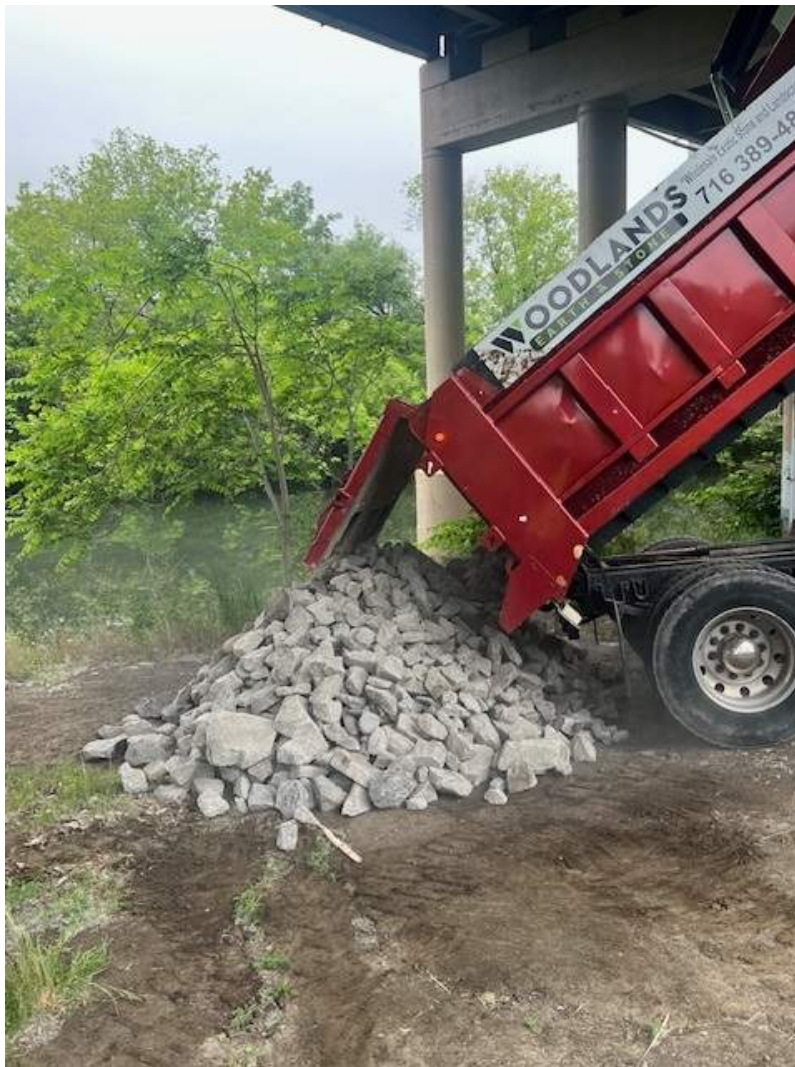
Photograph 1: Light Stone Fill being delivered to Site (Looking south).
