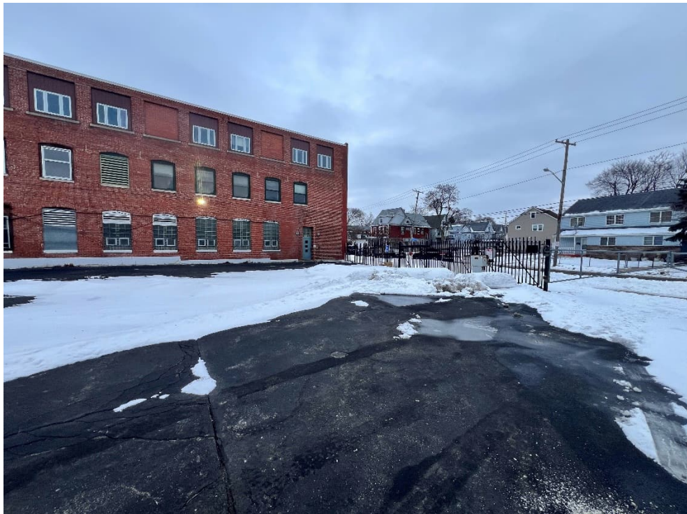
Photograph No. 6: Parking lot surface conditions. View is northeast.
