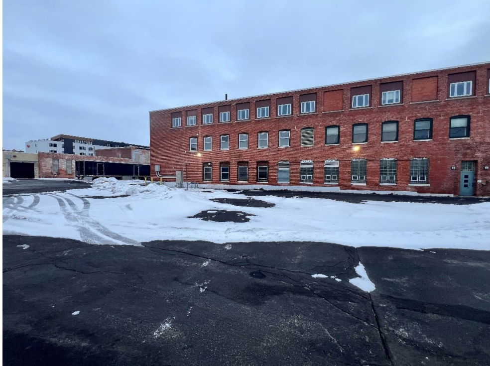
Photograph No. 5: Parking lot surface conditions. View is northwest.
