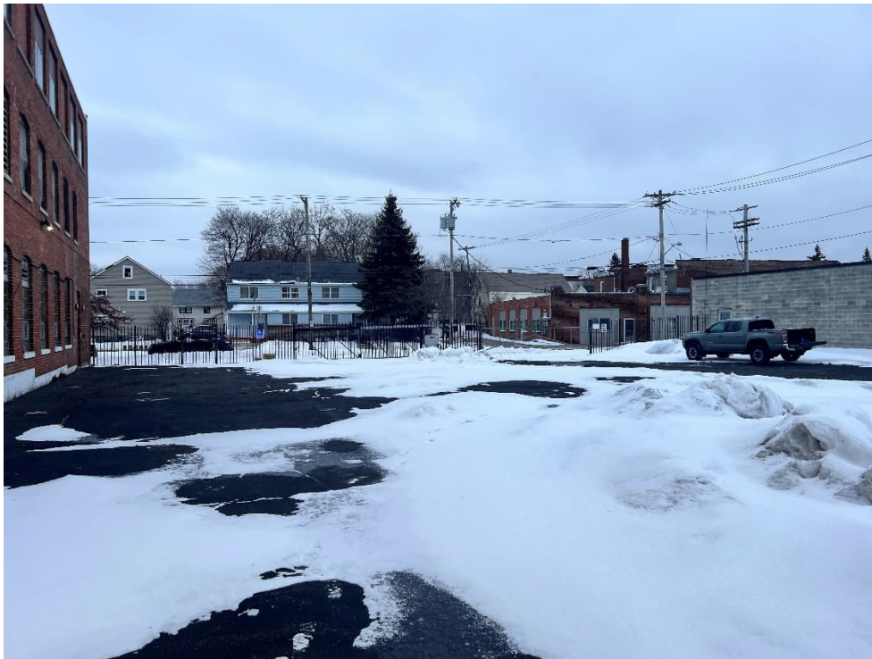
Photograph No. 2: Parking lot surface conditions. View is east.
