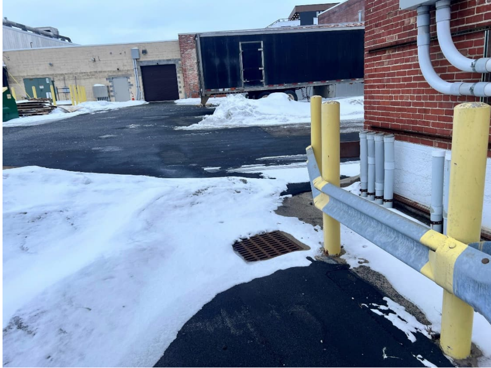
Photograph No. 1: Parking lot drainage and surface conditions. View is west.
