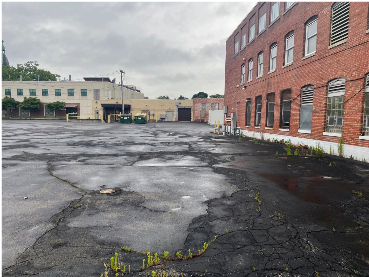
Asphalt cover conditions.
