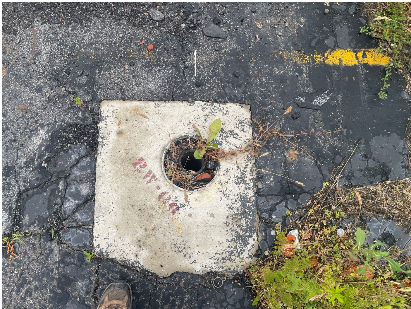
Aerial view of previously unknown well labeled "RW-06" with no cover and vegetation growing out of the side.
