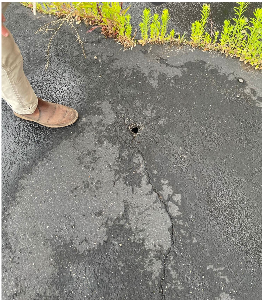
Small hole in asphalt near previously misidentified well.
