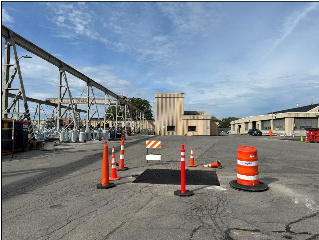
Site Conditions on September 28, 2023
