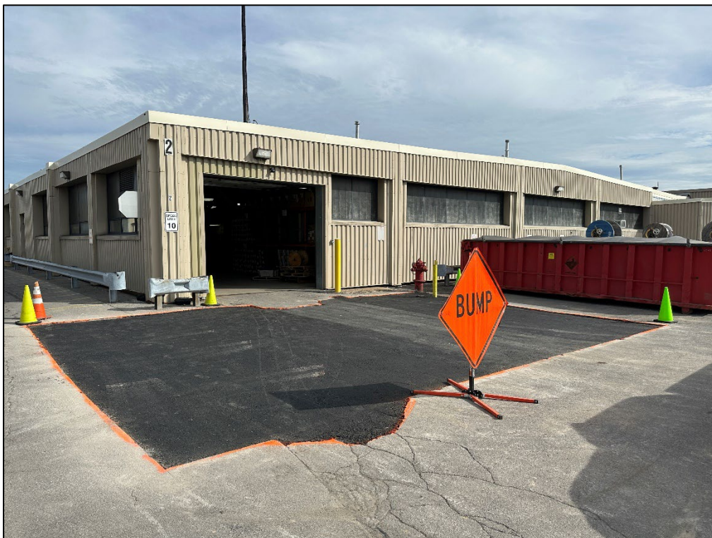
Site Conditions on September 28, 2023
