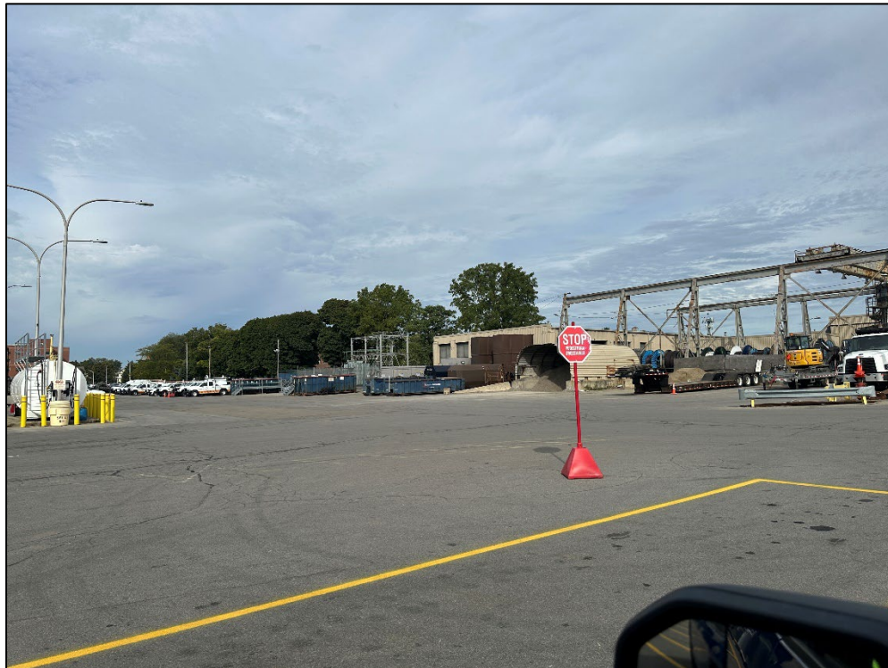
Site Conditions on September 28, 2023
