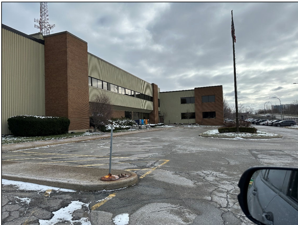
Site Conditions on March 21, 2024
