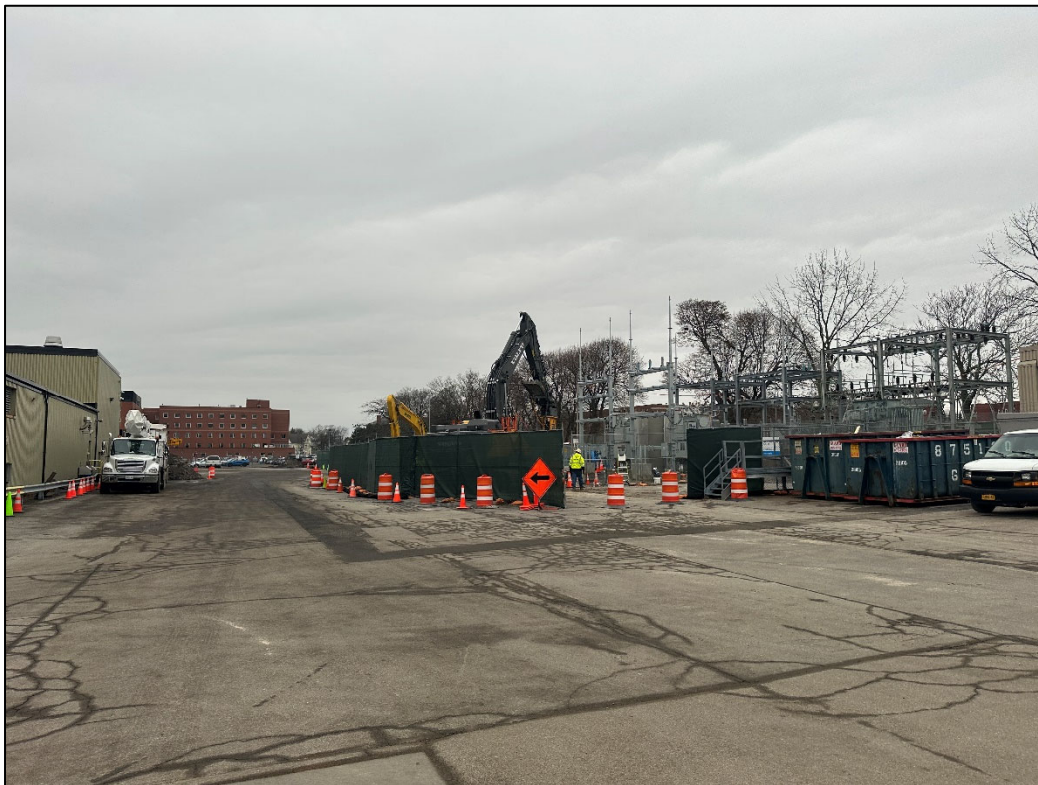
December 13, 2024 – Site Conditions
