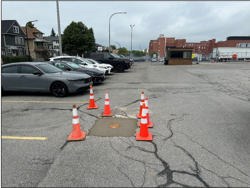
June 17, 2025 – Site Conditions
