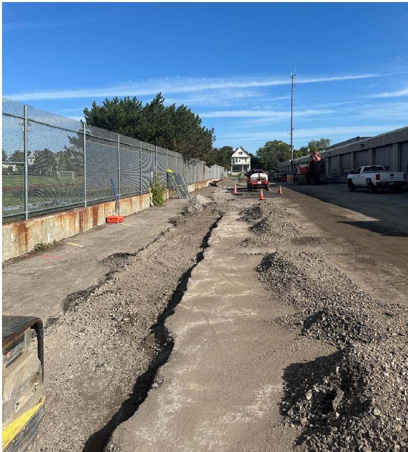
September 10, 2025 – Site Conditions
