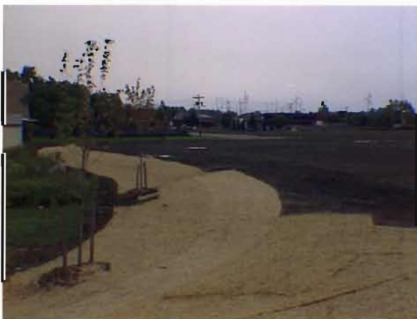
Figure 5 Yard Area, September 10, 1997 (Topsoil complete, erosion control fabric placed, ready for seed, mulch and fertilizer. View looking north.)
