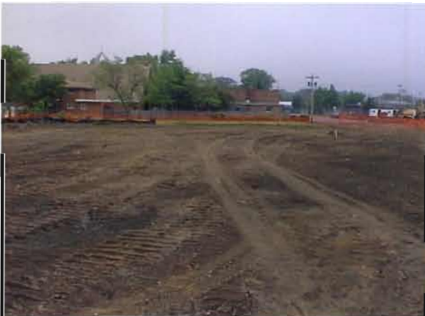
Figure 3 Yard Area, June 17, 1997 (Excavation complete ready for offsite soil cover. View looking north.)
