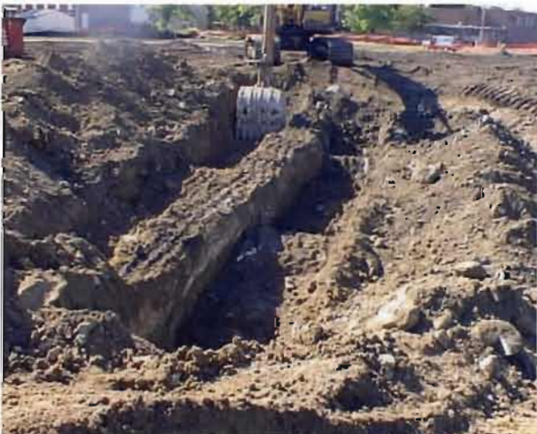
Figure 5 Concrete encased conduit found in northwest leg of I-Basin. July, 1997.
