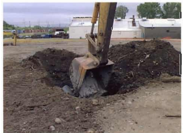
Figure 4 The UST was placed into the waste cell, crushed and covered.
