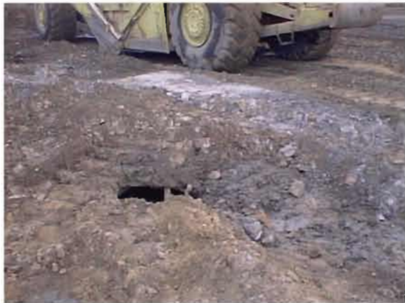
Figure 2 During the one foot excavation this pan uncovered this UST.
