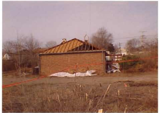
Figure 2 Building No.1, April 11, 1997 (Asbestos removal operations underway. Note darkened triangle which contained extra ACM.) See Appendix 2.
