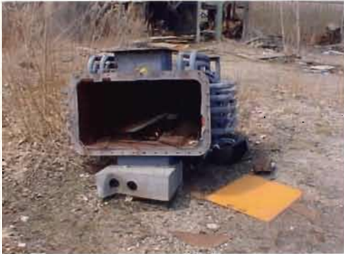
← PCB CONTAMINATED TRANSFORMER
