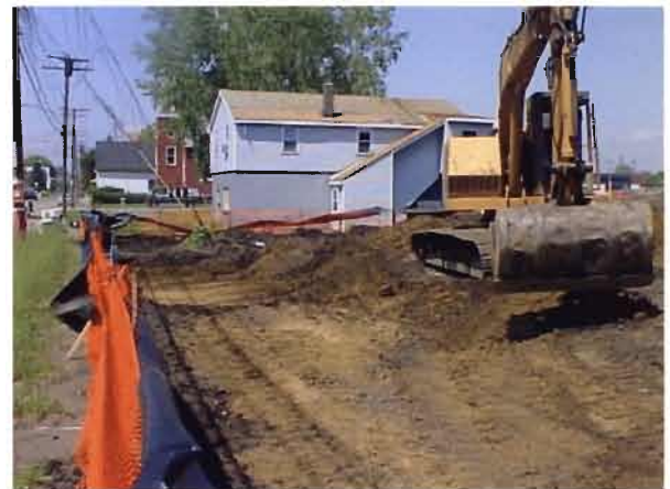
Figure 4 Ingham Avenue, June 19, 1997, Excavation to one foot. View looking north.)
