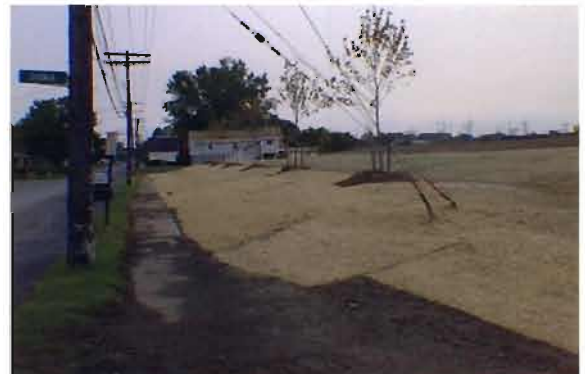
Figure 5 Ingham Avenue, September 10, 1997 (Erosion control mat placed over topsoil, trees planted. View looking north.)
