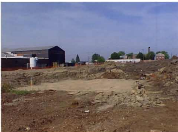
Figure 5 PCB Hotspot Number 4, June 11, 1997 (Area backfilled with Type "A" clay and compacted after confirmatory sampling results)
