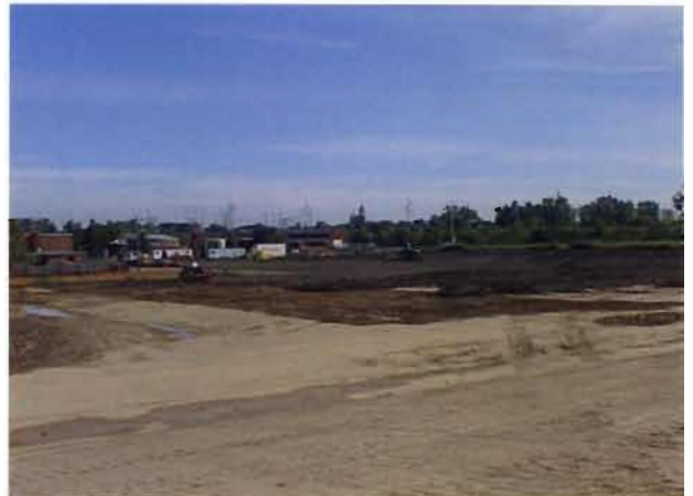
Figure 4 Yard Area, August 19, 1997 (Placing topsoil. Note compacted Type "A" clay disked to accept topsoil. View looking northeast.)
