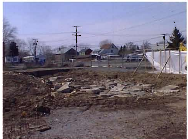
Figure 4 Building No. 1, April 30, 1997 (Demolished foundation walls placed flat in excavation.)
