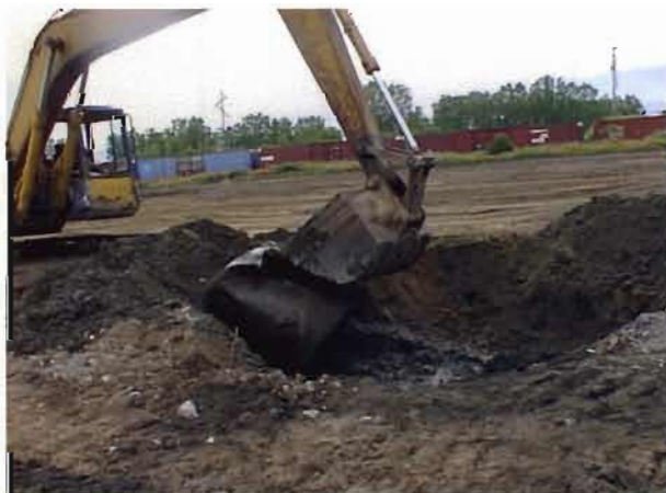
Figure 5 The UST was removed from the excavation.
