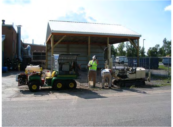
Date: August 6, 2009 Site: Former Scott Aviation - Area 2 SI
