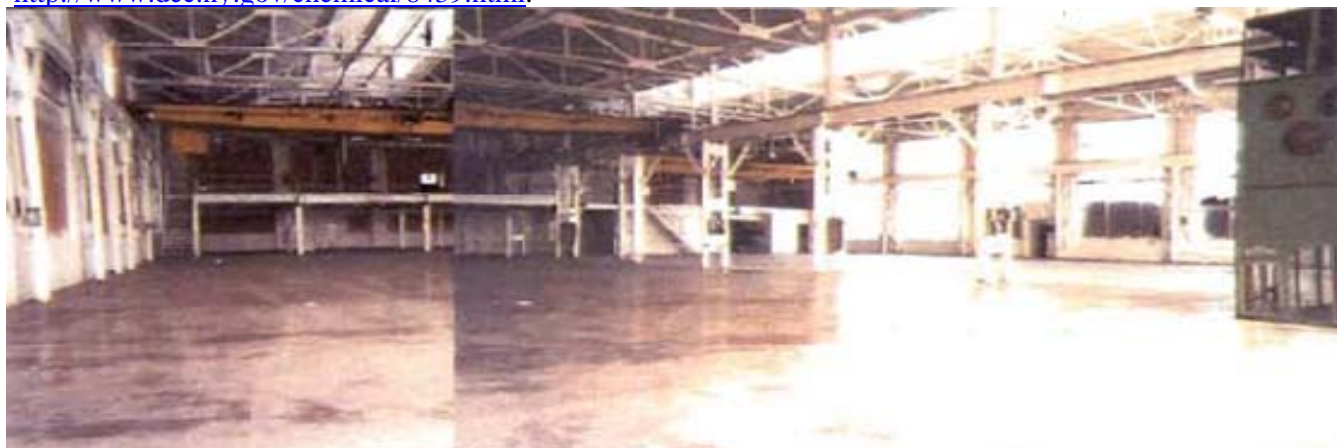
After remediation: Panoramic photo of building interior after debris removed, new floor and interior painting
