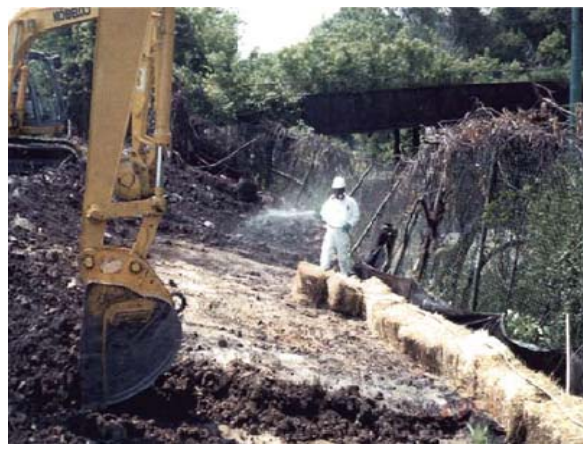
During remediation: Excavation along fence line, using water for dust control
