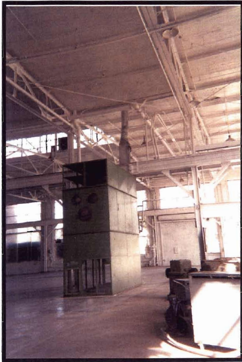
Photo 37: Johnson Heater Following Interior Painting Construction of New Floor
