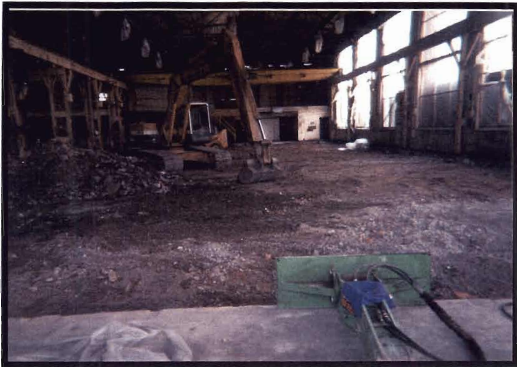
Photo 25: Removal of Concrete Floor
