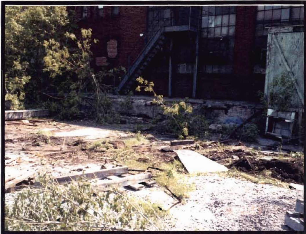
Photo 1: Debris and Loading Dock West of Building Prior to Beginning Work [View to East]
