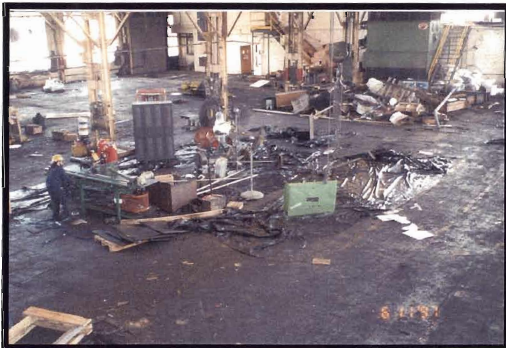
Photo 20: Stockpiling of Cleaned Equipment Inside Building
