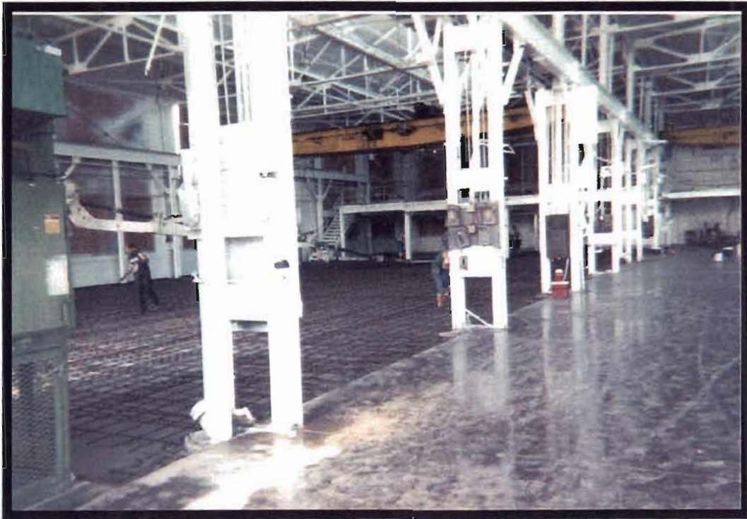
Photo 29: Placing Steel Mats on South Floor, New North Floor on Right
