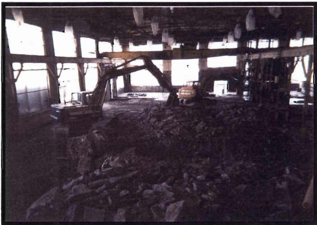
Photo 26: Stockpiling of Floor Waste (Concrete)
