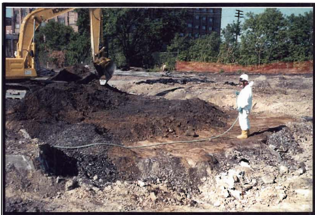
Photo 6: Excavation of Northwest Corner (Area 1) Under Former Concrete Pad Using Water for Dust Control [View to West]
