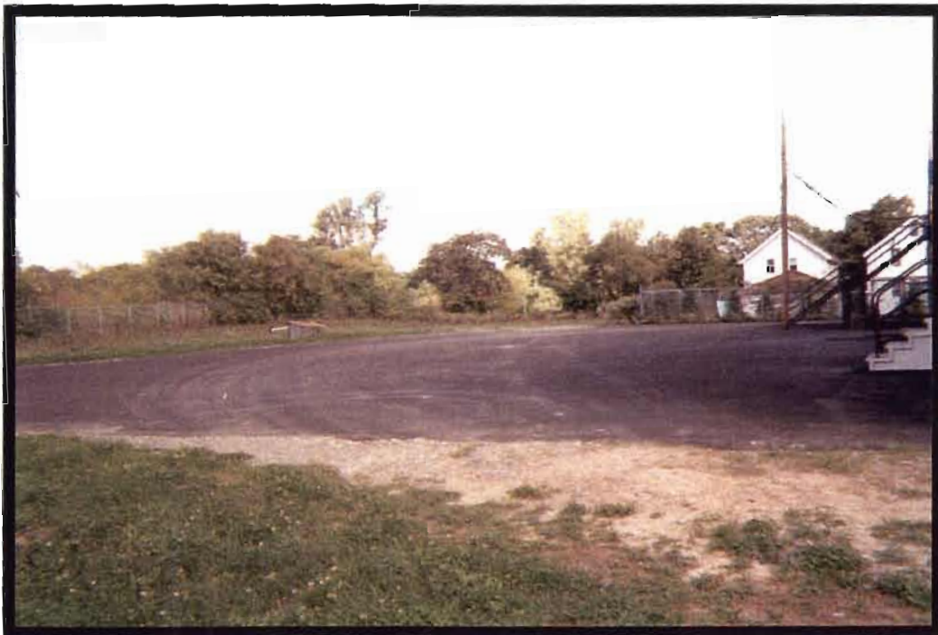
Photo 35: New Asphalt West of Building [View to North]
