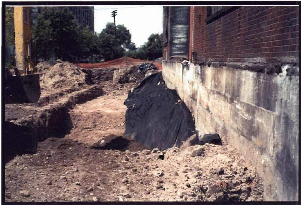
Photo 11: Geotextile Placed Along South Building Wall (VOC Area) [View to West]
