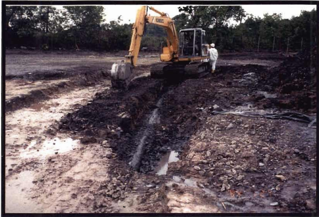
Photo 15: Excavation of Rail Spur and Drainline West End of Property (Area 3) [View to West]
