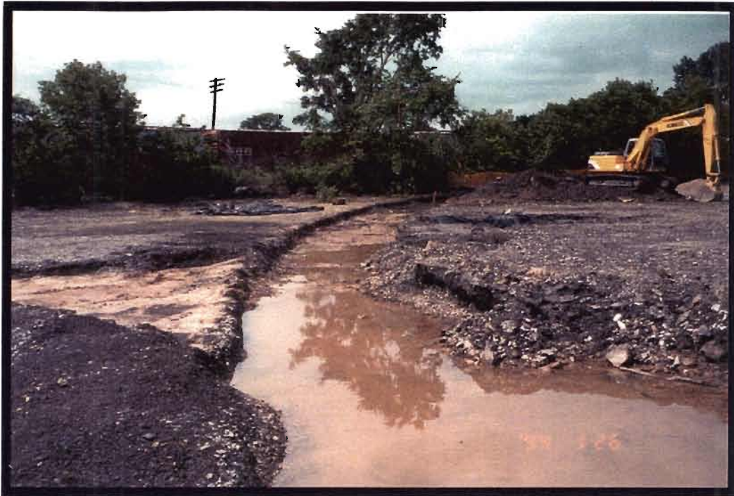
Photo 13: View of West End of Property (Area 3) Following Heavy Rainfall [View to Northwest]
