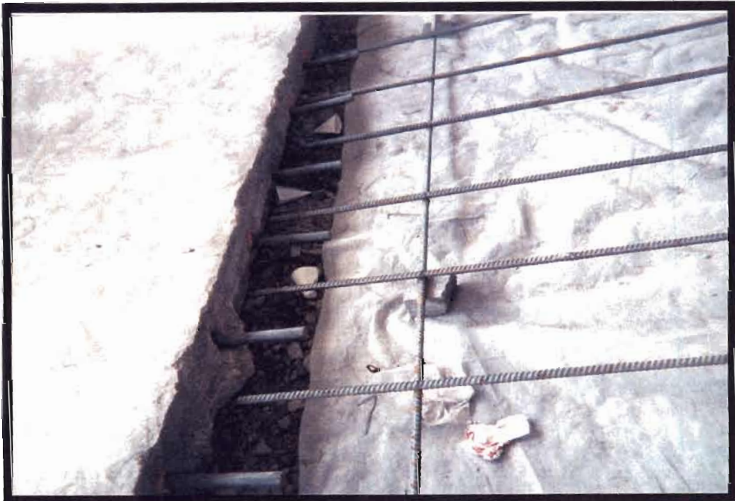
Photo 30: Steel Dowels Along East Floor Joint
