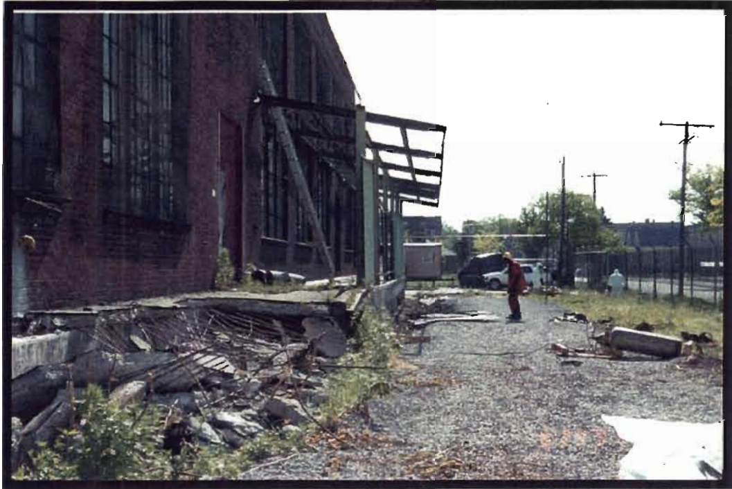
Photo 7: Demolition of South Loading Dock [View to East]
