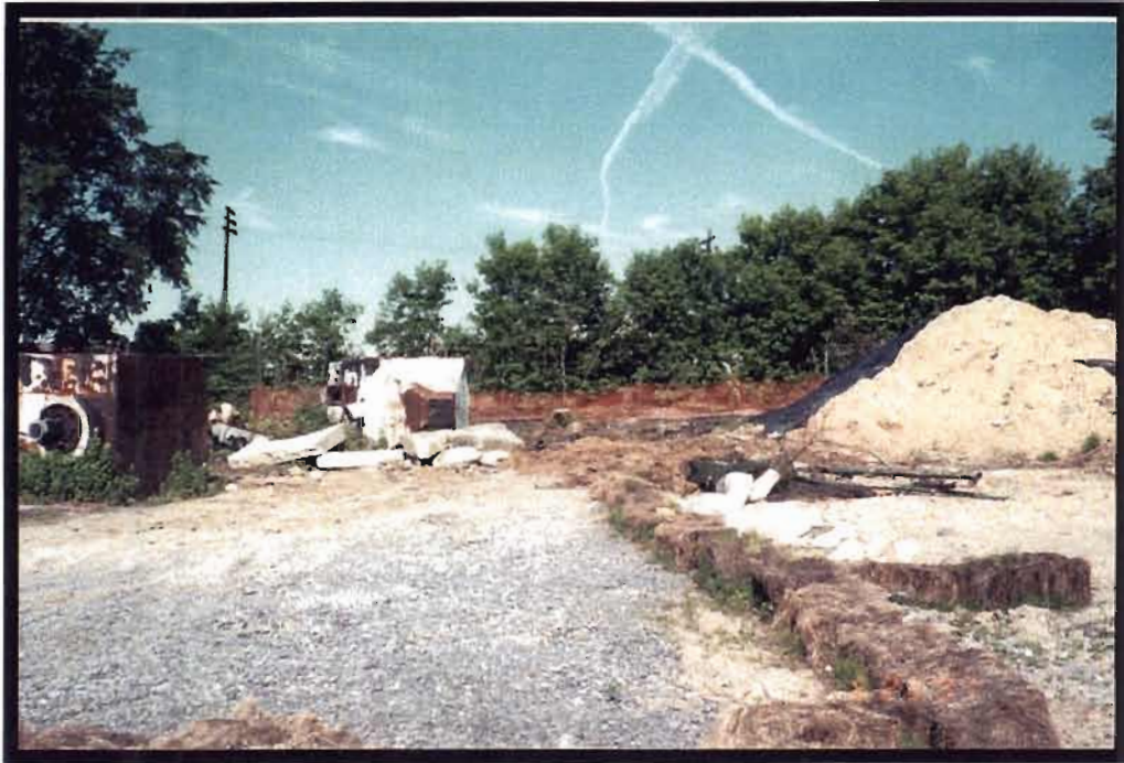
Photo 3: Miscellaneous Debris and Soil Piles on West End of Building prior to Start of Field Work [View to West]
