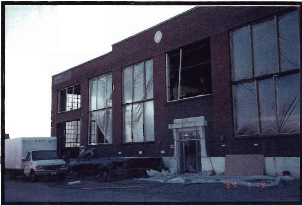
Photo 23: Removal of Windows and Installation of Temporary Enclosures [View to Southwest]
