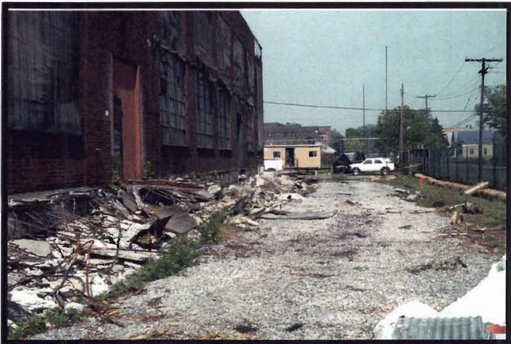
Photo 8: Demolition of Loading Dock [View to East]
