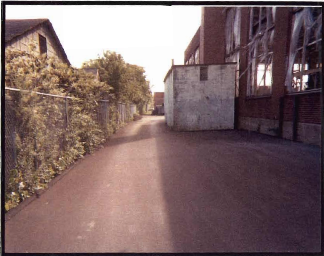
Photo 34: New Asphalt North of Building [View to East]
