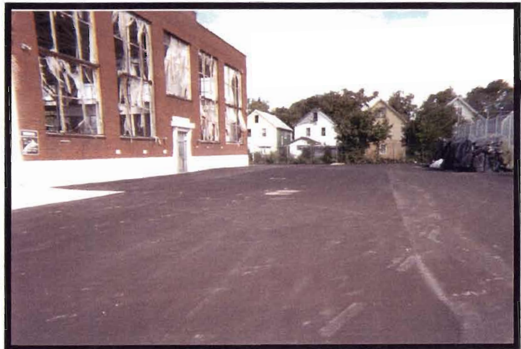
Photo 33: New Asphalt East of Building [View to North]
