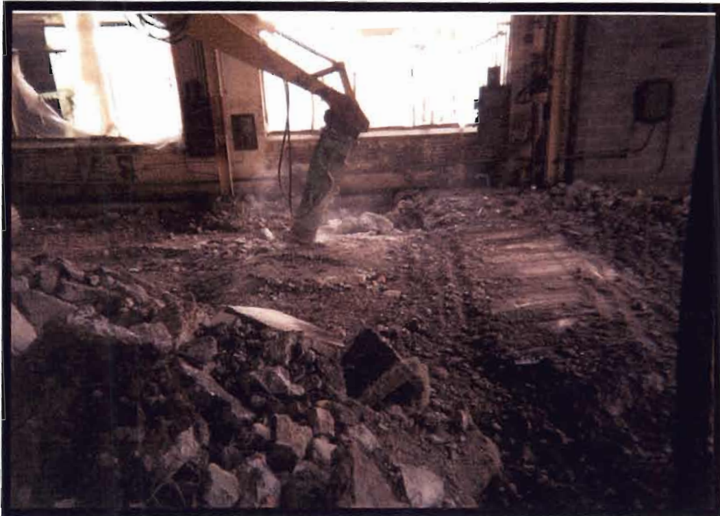
Photo 27: Removal of Concrete Floor
