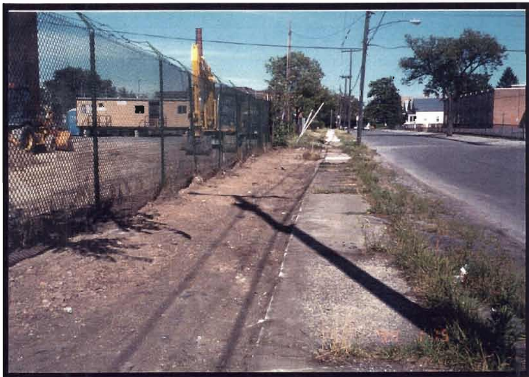
Photo 12: Removal of Surface Soils Along City of Buffalo Right-of-Way [View to East]
