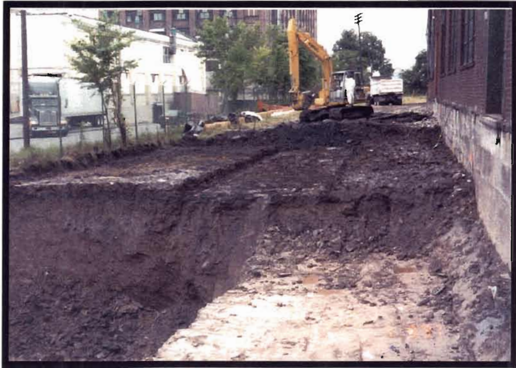
Photo 9: Excavation South of Building, Former Rail Spur Location in Center of Photo [View to West]
