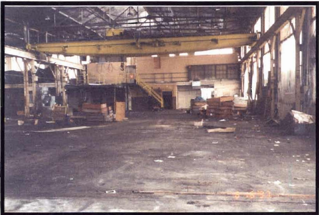
Photo 18: Building Interior with 90% of Equipment Removed
