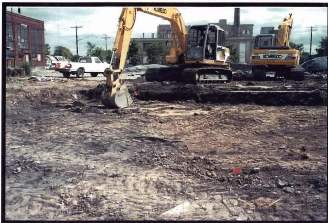
Photo 5: Excavation of Area 1 - Northwest Corner. Concrete Pad Under Trackhoe [View to South]
