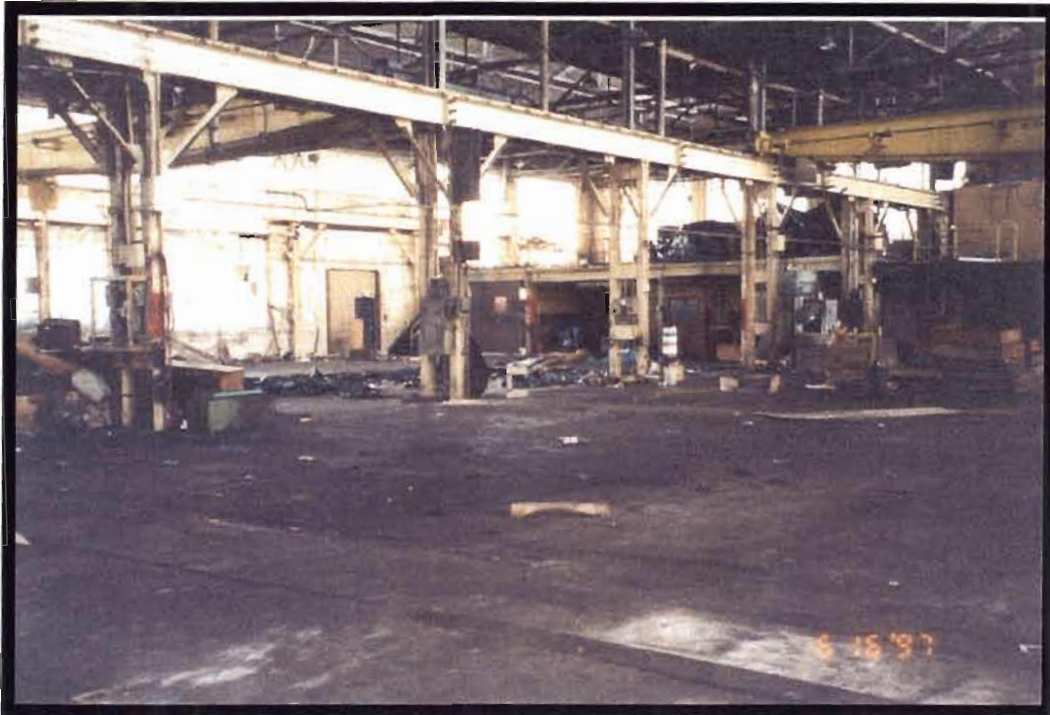
Photo 19: Building Interior with 90% of Equipment Removed
