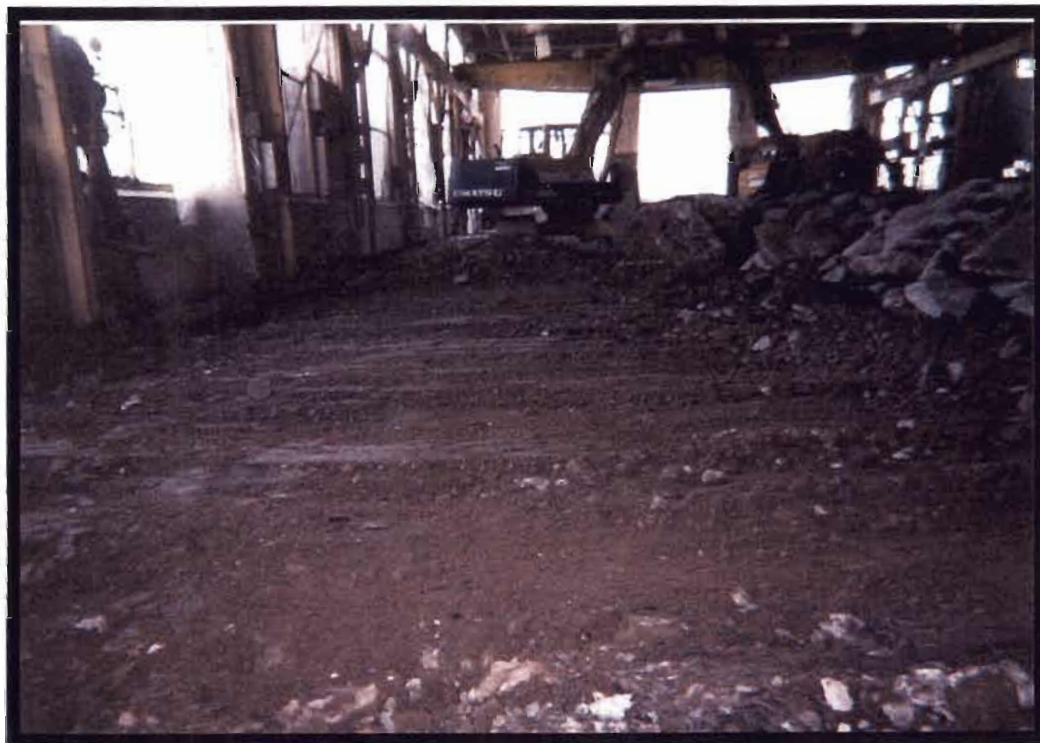
Photo 24: Removal of Concrete Floor
