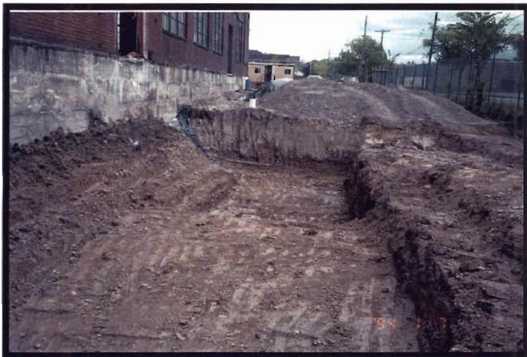
Photo 10: Deep Excavations South of Building (Area 2) [View to East]
