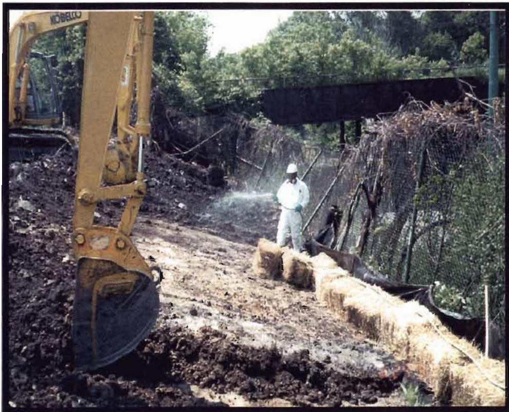
Photo 4: Excavation Along Fenceline Area 1, Using Water for Dust Control [View to West]
