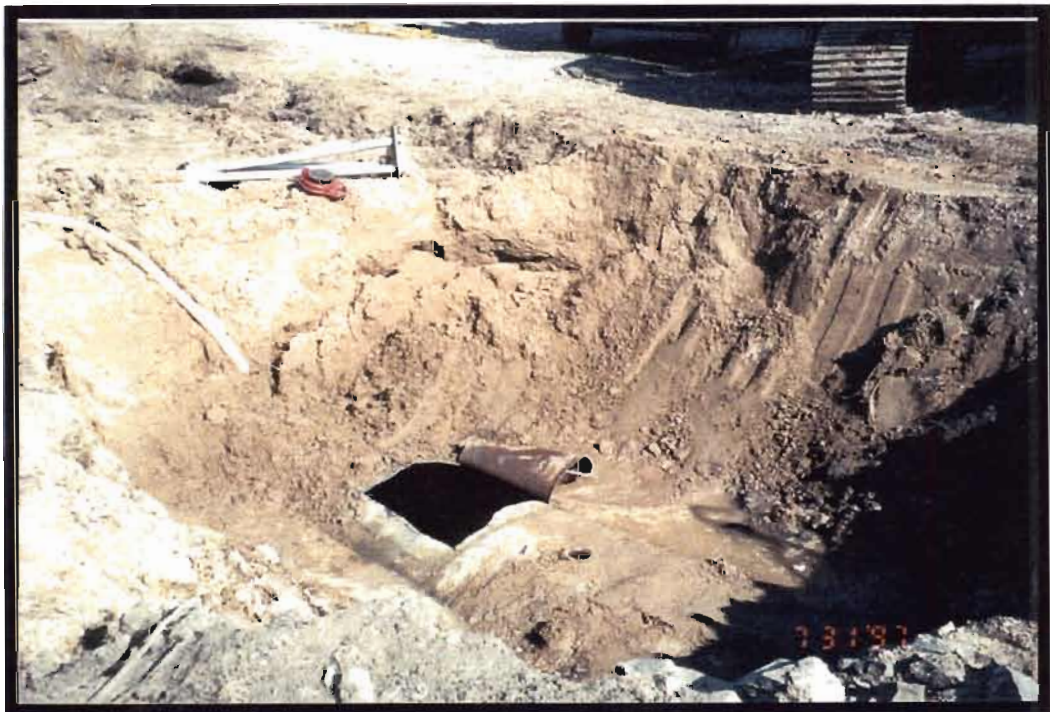
Photo 16: UST Exposed for Cleaning Prior to Removal. Southwest of Building [View to Southeast]
