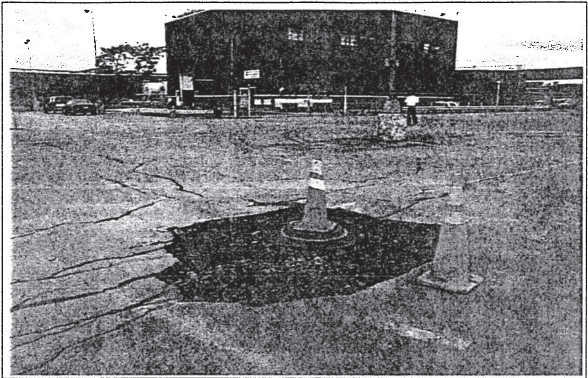
Photograph 31: Phase I paving area during prep work. Manhole repair area in forefront.
