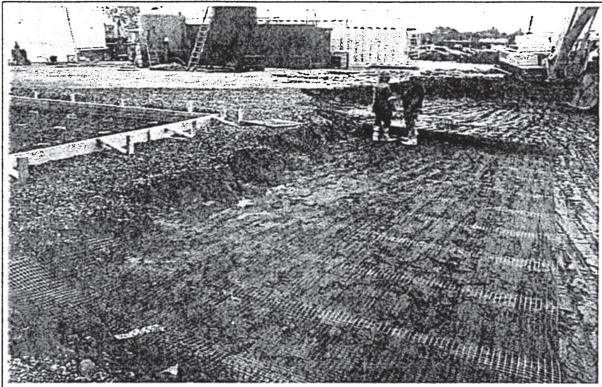
Photograph 25: Looking southward across main excavation at placement of Geogrid.
