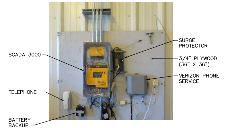
TYPICAL SCADA 3000 MOUNTING DETAIL
