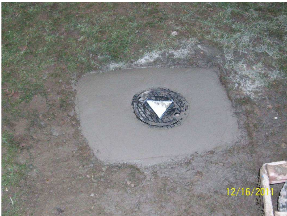
Figure 18: View of Finished Well Pad at EE-3
