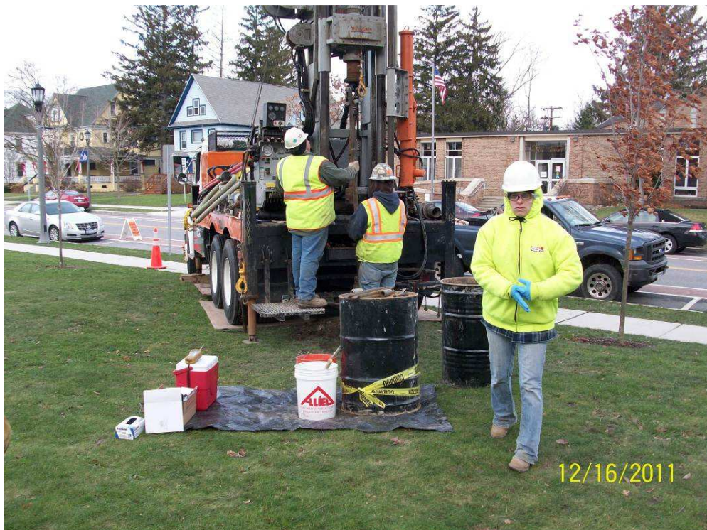
Figure 20: View of Work Zone during Drilling
