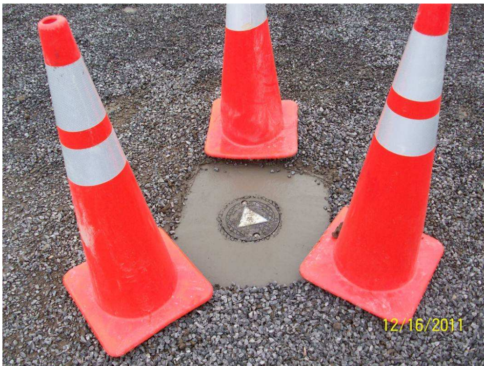
Figure 2: View of finished well pad at EE-4 (AM)
