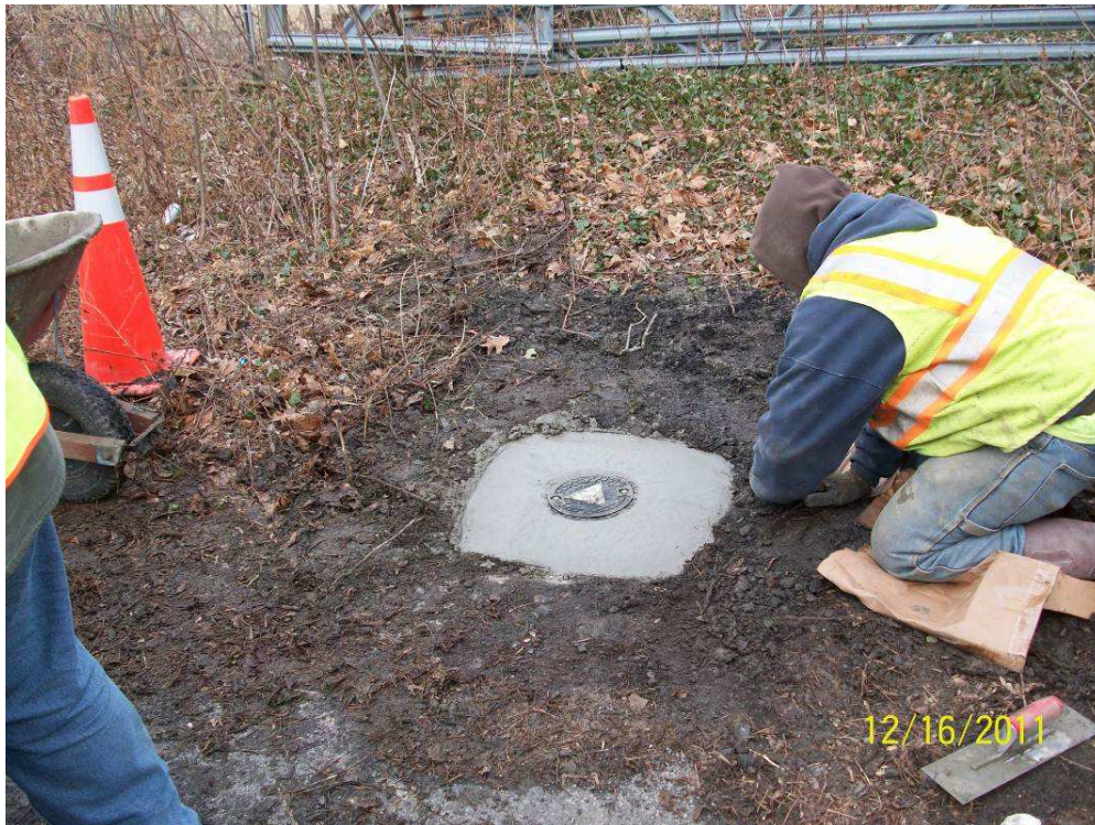
Figure 3: View of Finished Well Pad at ESI-2-R (AM)
