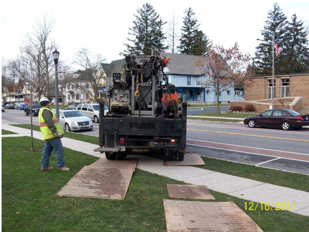
Figure 4: View of GES setting the rig on EE-3 (AM)
