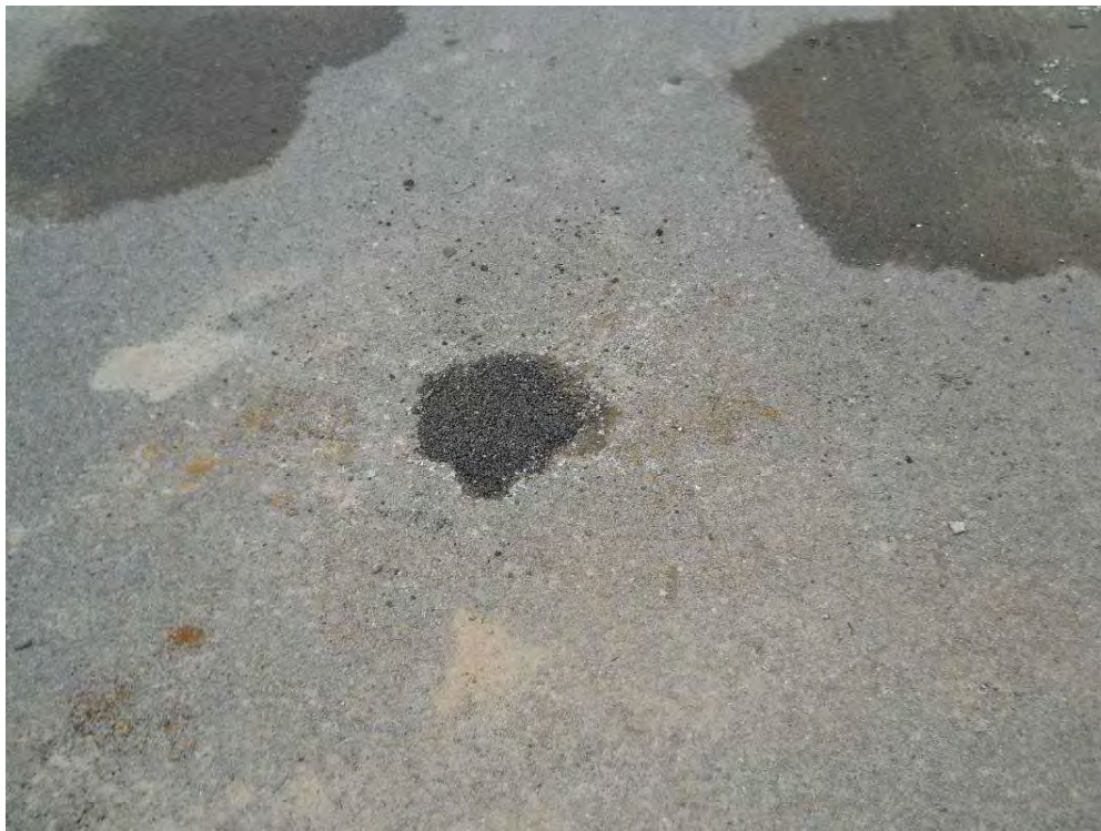
Figure 11: View of patched ESI-5 after decommissioning of the well (Looking down, PM)
