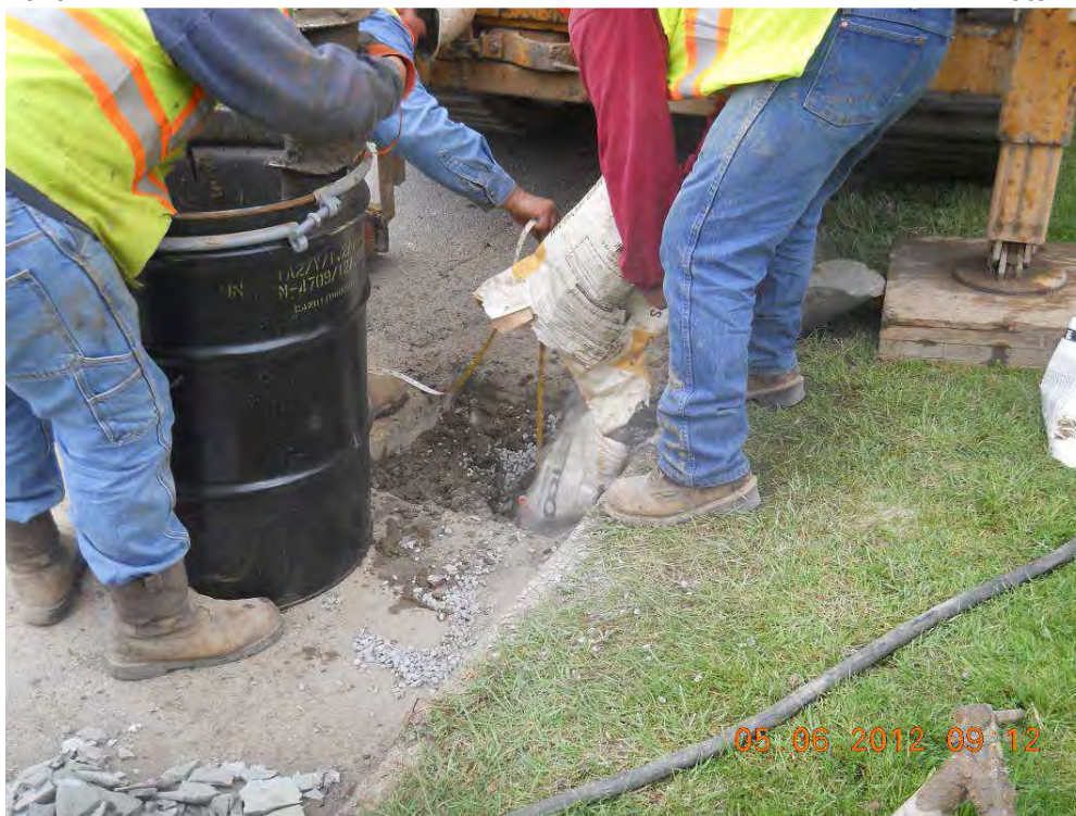
Figure 1: View of bentonite seal in MPI-8S-R (Looking WSW, AM)
