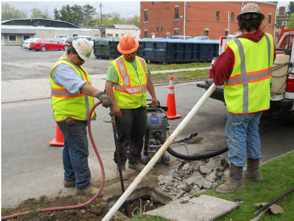
Figure 2: View of hand clearing borehole MPI-8S-R (Looking S, PM)
