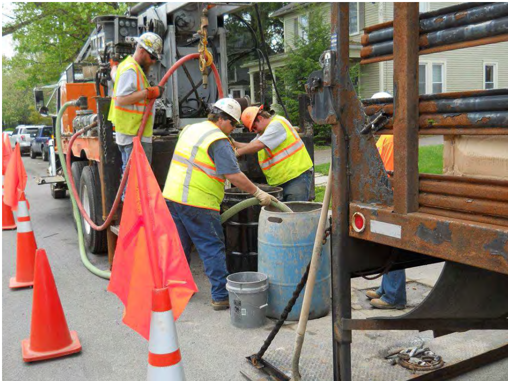
Figure 6: View of tremie grouting at ESI-5 (Looking W, PM)
