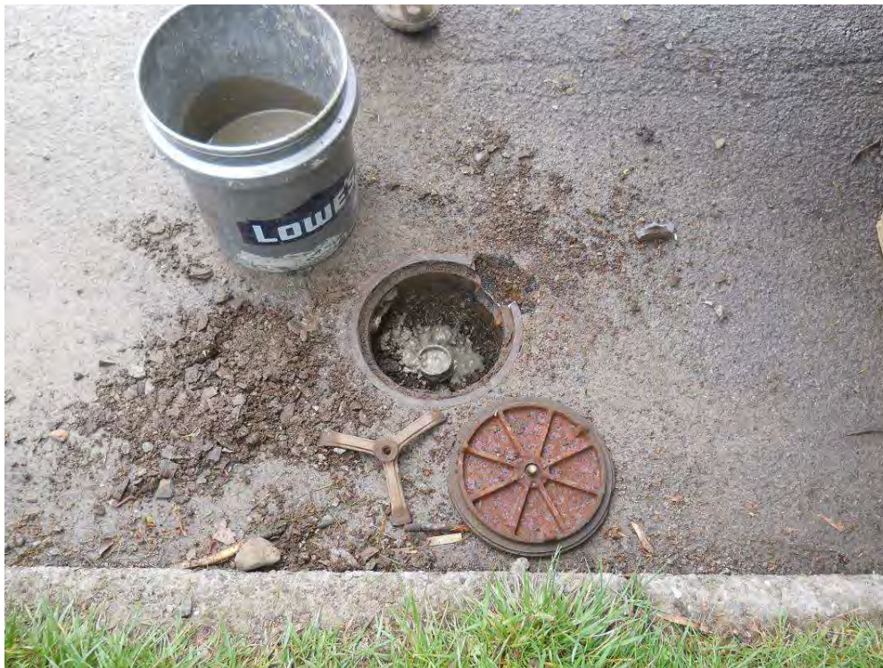
Figure 1: View of grouted well MPI-8S (Looking S, AM)
