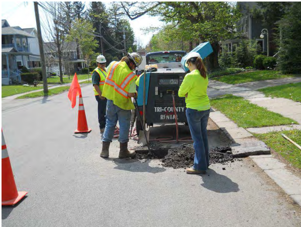
Figure 5: View of hand clearing ESI-5-R to a depth of 5-8 feet (Looking W, PM)
