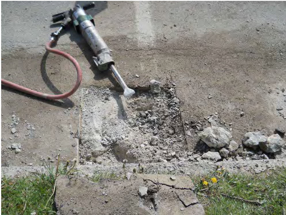
Figure 1: View of hand clearing borehole MPI-8S-R (Looking S, PM)
