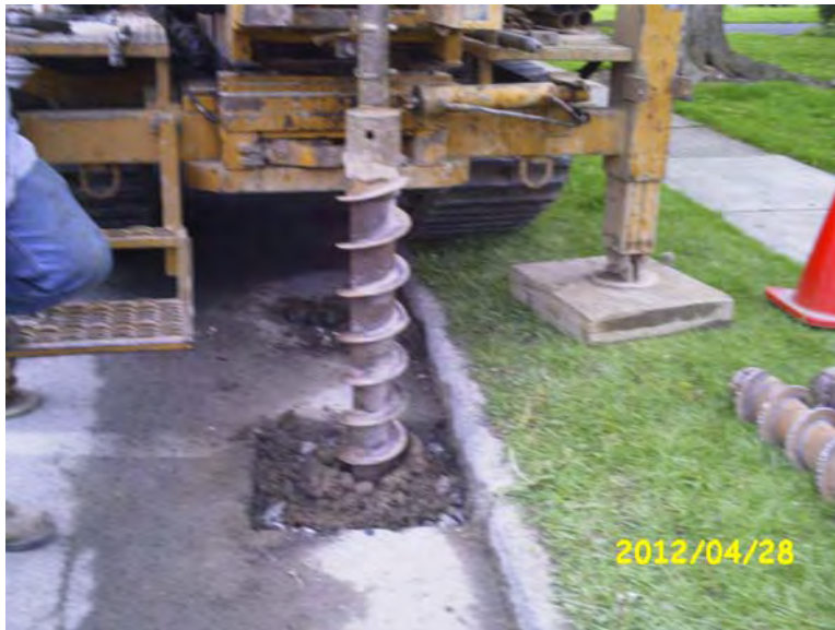
View of augering MPI-13B-R.
