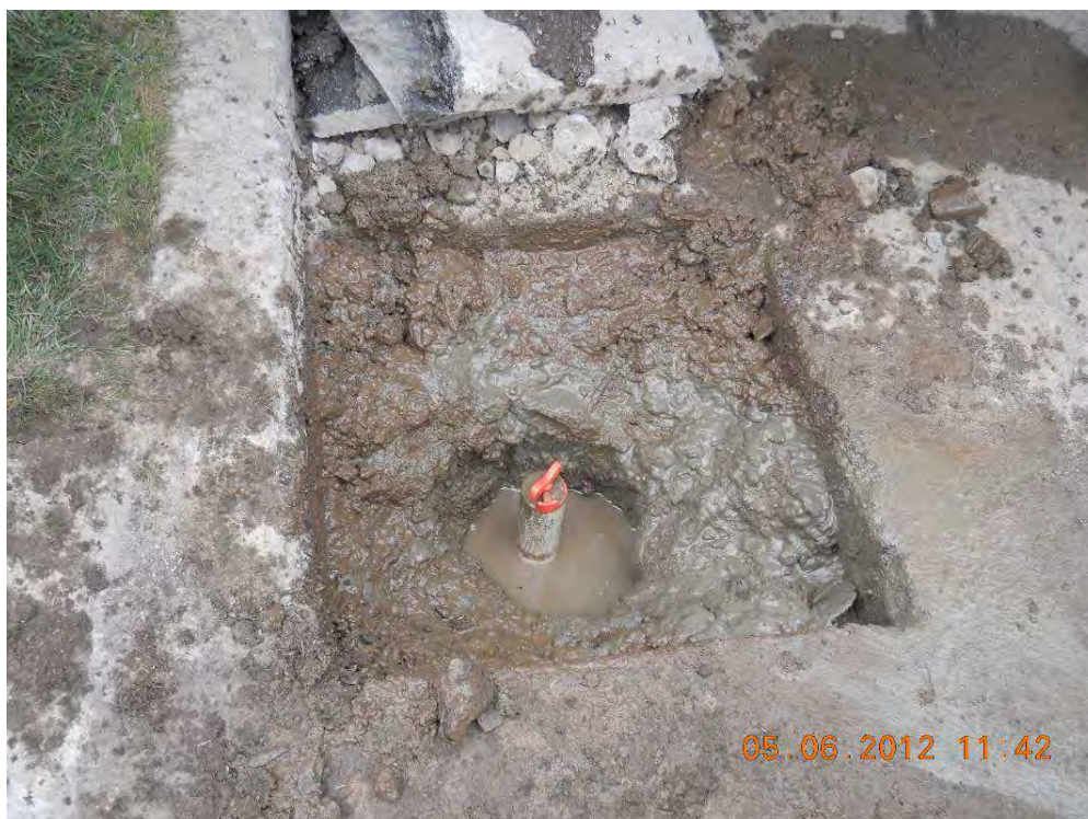
Figure 4: View of grout at MPI-9S-R (Looking NE, AM)
