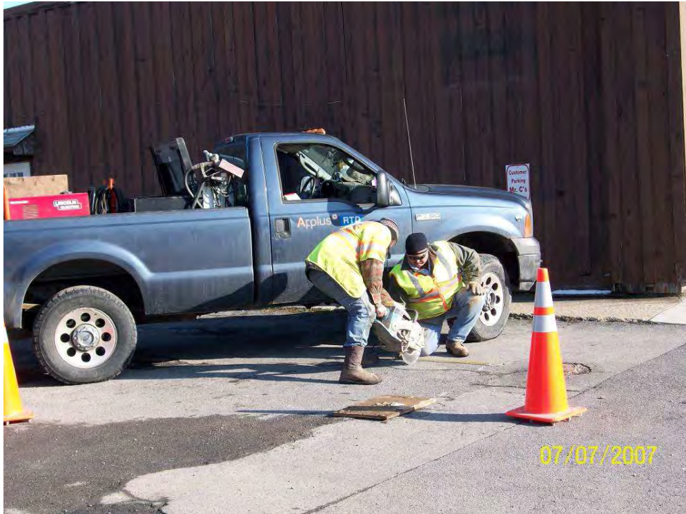
Figure 1: View of Saw Cutting for Utility Clearance at MPI-7I-R (Looking NE)
