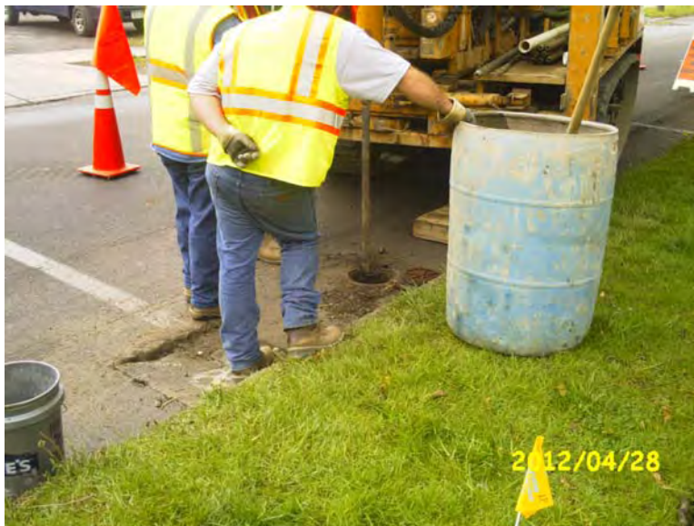
Hammering out road box ring for MPI-14B in preparation for abandonment.
