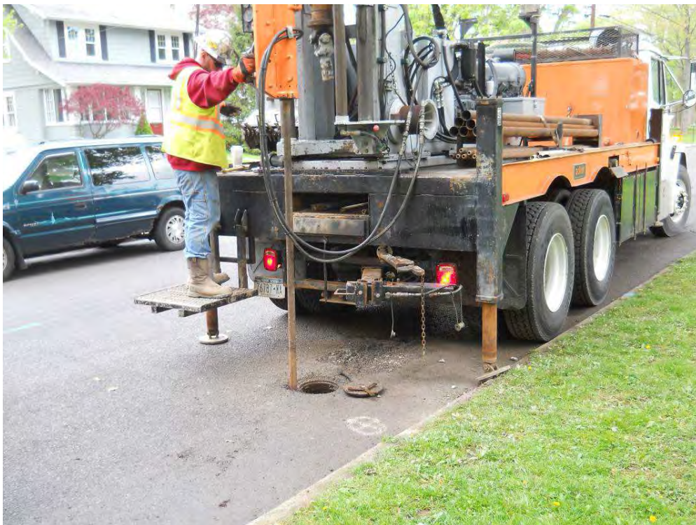
Figure 4: View of removal of MPI-13B manway by slam bar around the cast iron ring (Looking SSE, AM)
