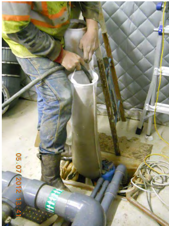
Figure 4: View of discharging decon water through filter into treatment system sump (Looking S, PM)
