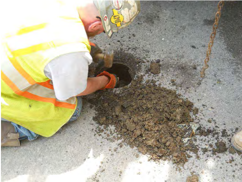
Figure 7: View of removal of cub box at ESI-5 (Looking down, PM)
