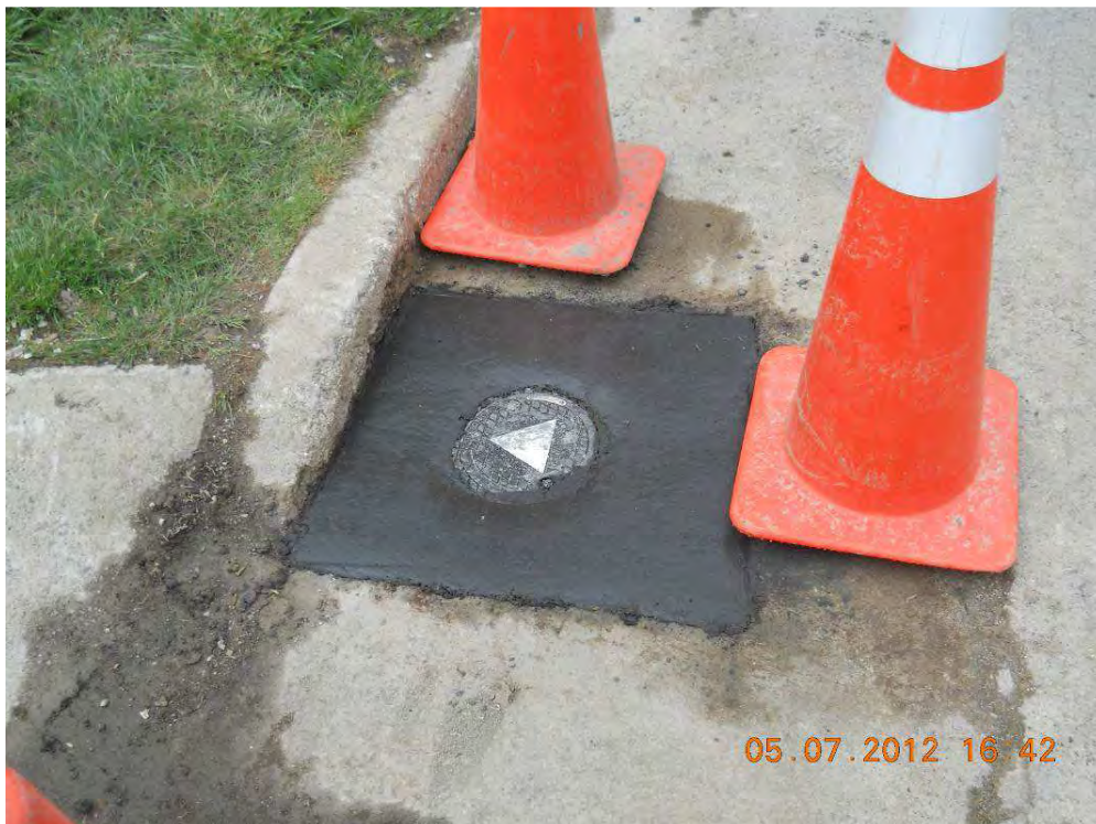
Figure 8: View of MPI-9S-R after construction of well pad (Looking E, PM)
