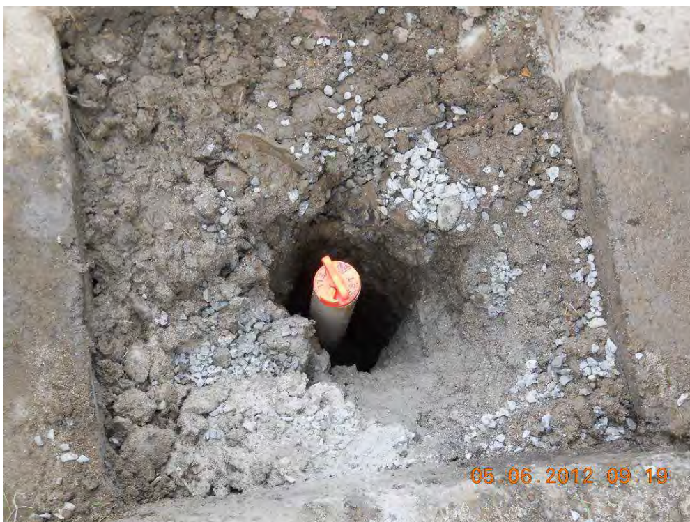
Figure 2: View of well following placement of bentonite in MPI-8S-R (Looking S, AM)
