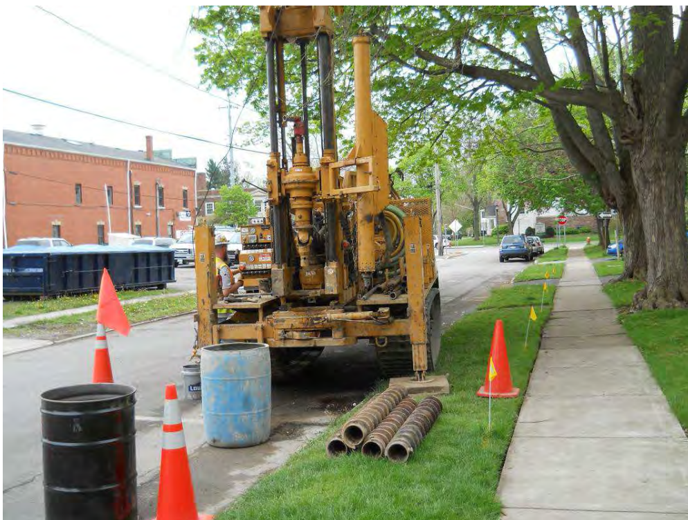
Figure 8: View of drill rig set up at MPI-8S to install new well (Looking W, PM)
