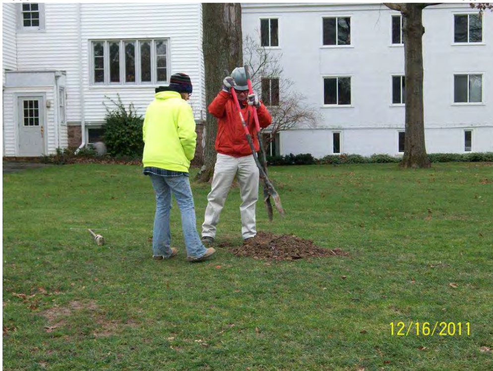
Figure 1: View of Hand Excavation to 5' for Utility Clearance at EE-3 (Looking South AM)
