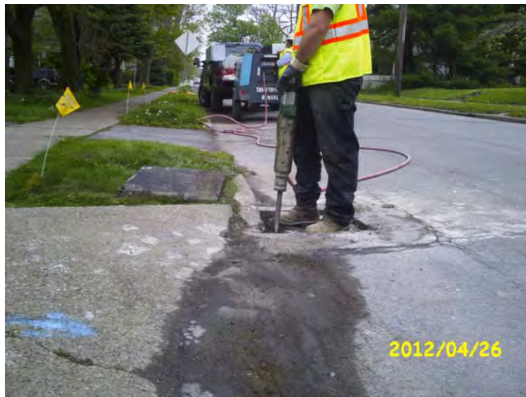
Jack hammering MPI-8S-R location through concrete in preparation to hand clear.
