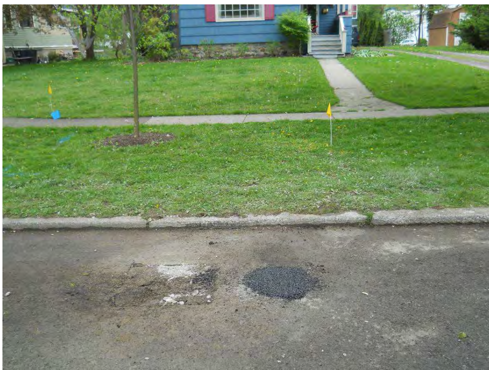
Figure 12: View of patched MPI-13B after decommissioning of the well (Looking W, PM)
