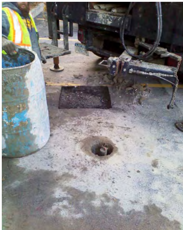
View of MPI-2S abandonment location (square patch) and MPI-2S-R prior to building well pad.
