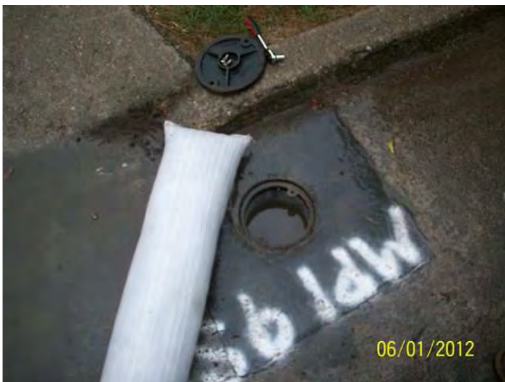
Figure 6: View sand bag to deflect rainstorm runoff from filling well vault at MPI-9S-R (Looking N)
