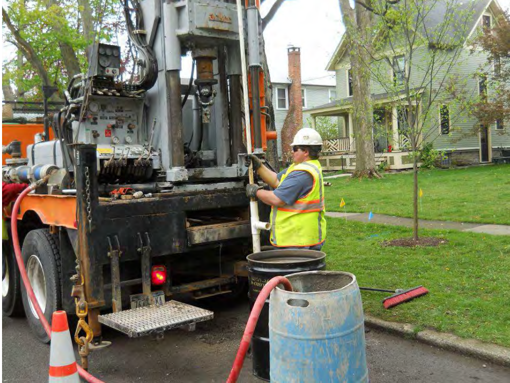
Figure 5: View of set up for tremie grouting MPI-13B (Looking SW, AM)
