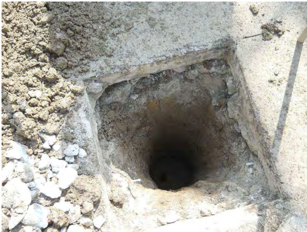
Figure 3: View of hand-cleared borehole MPI-9S-R to 6.5 feet, hitting cobble rock (Looking S, AM)
