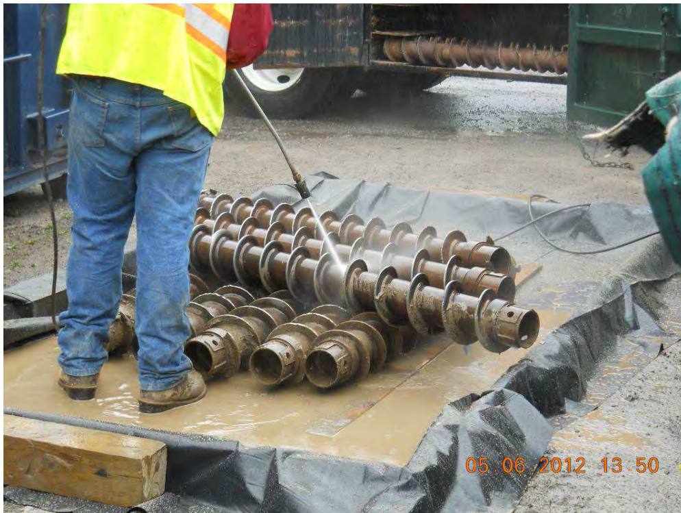
Figure 7: View of auger decon (Looking E, PM)
