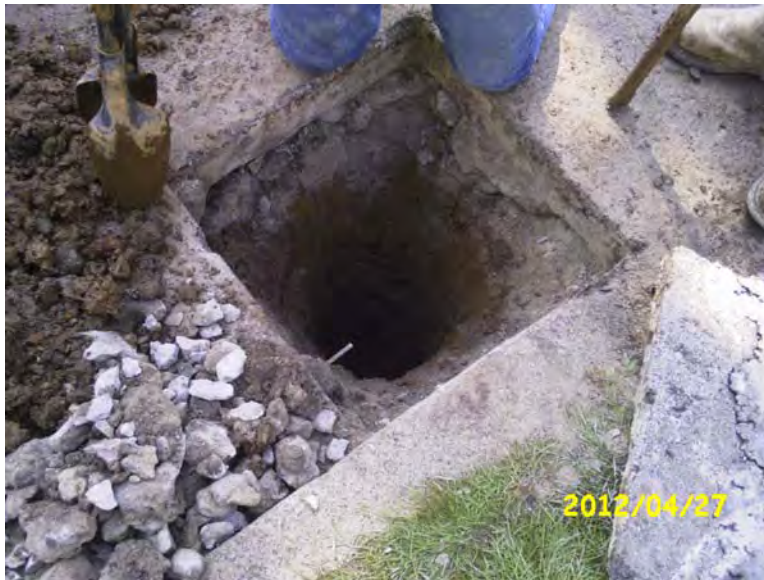
Hand cleared borehole for MPI-9S-R.
