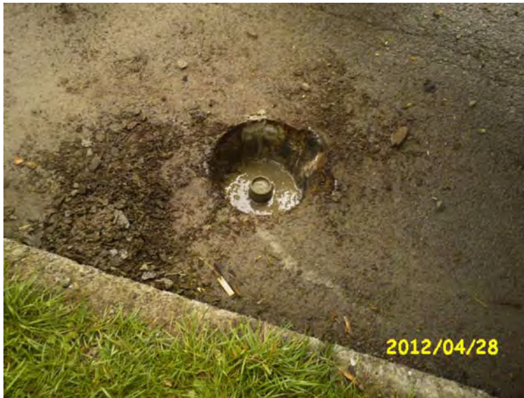
Grout mixture in MPI-14B for abandonment.
