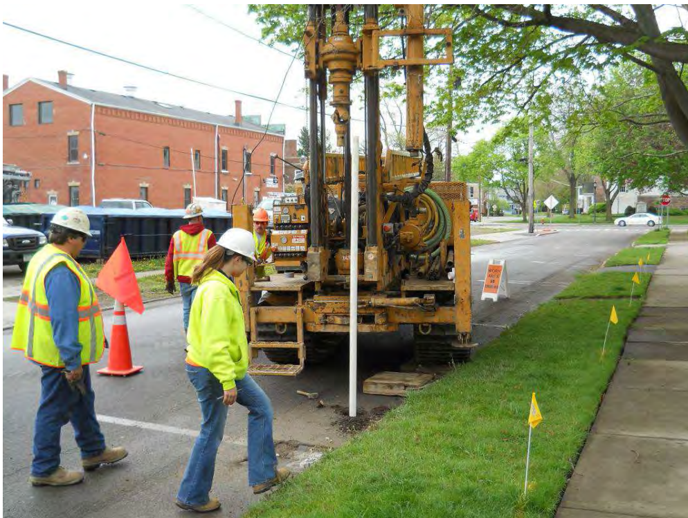
Figure 10: View of installation of well riser at MPI-8S (Looking W, PM)
