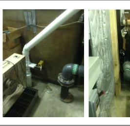
2. Installing riser pipes with valves west and east of tank
