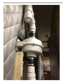
LEFT: Extraction fan (RadonAway, model GP5001; rated 80 cfm at 2" WC static suction) with condensate bypass on discharge side to drain moisture during cold weather.
