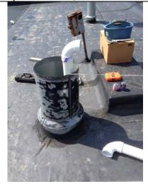
6. Installing pipe through air stripper inlet vent on the roof
