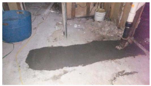
Example of repair to floor penetration with concrete.
