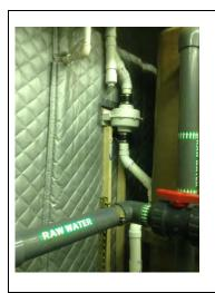
4. Extraction Fan on wall behind southeast corner of tank (RadonAway Model GP501; rated 80 cfm at 2" WC)
