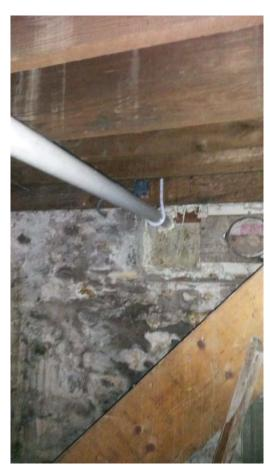
SSDS piping beneath fitness center exiting building through former basement window.
