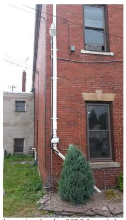
View of eastern exhaust pipe showing SSDS fan and electrical components.
