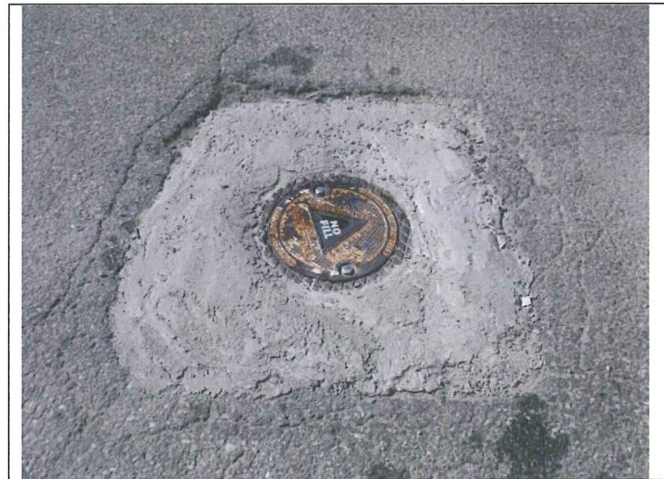
2. PZ-1B after concrete repair with MG-KRETE
