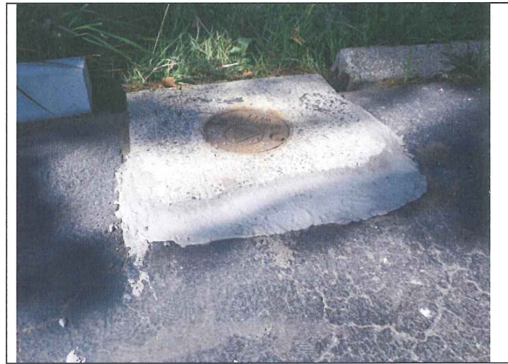
4. PZ-6C after snowplow damage repair with MG-KRETE
