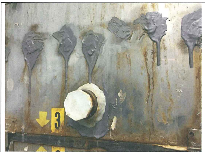
3. Air Stripper showing epoxy repairs on corroded areas
