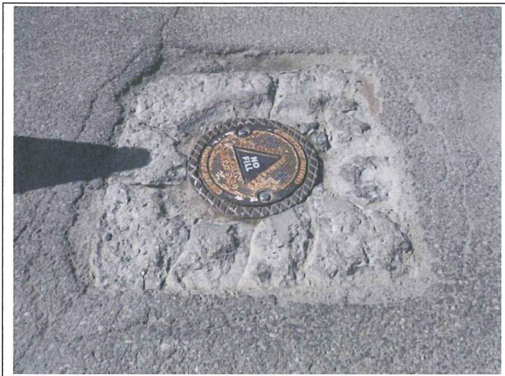
1. PZ-1B showing concrete damage from winter conditions
