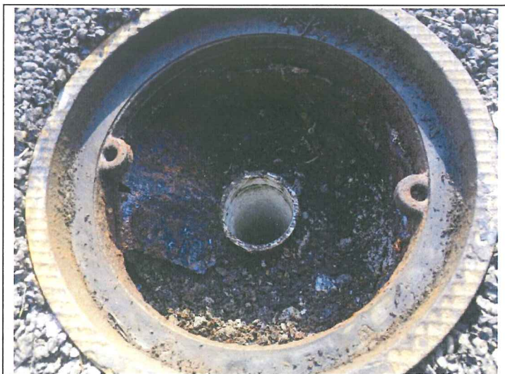
1. PZ-4B showing snowplow damage to inner ring
