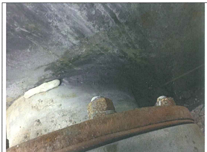
4. Air Stripper effluent fitting showing epoxy repairs
