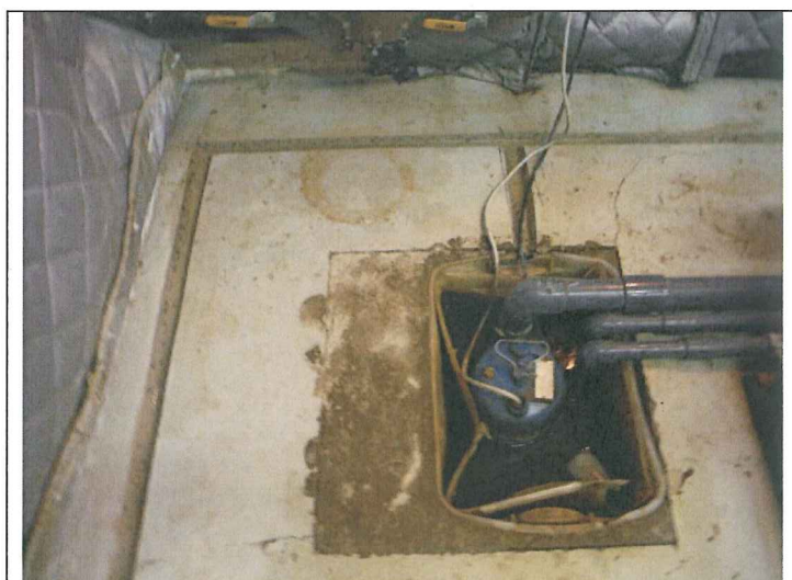
6. Liquid Containment Trench at southeast corner of the Treatment Room
