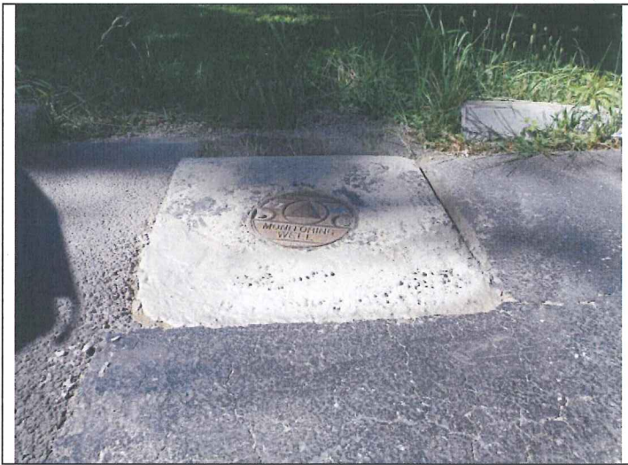
3. PZ-6A after snowplow damage repair with MG-KRETE
