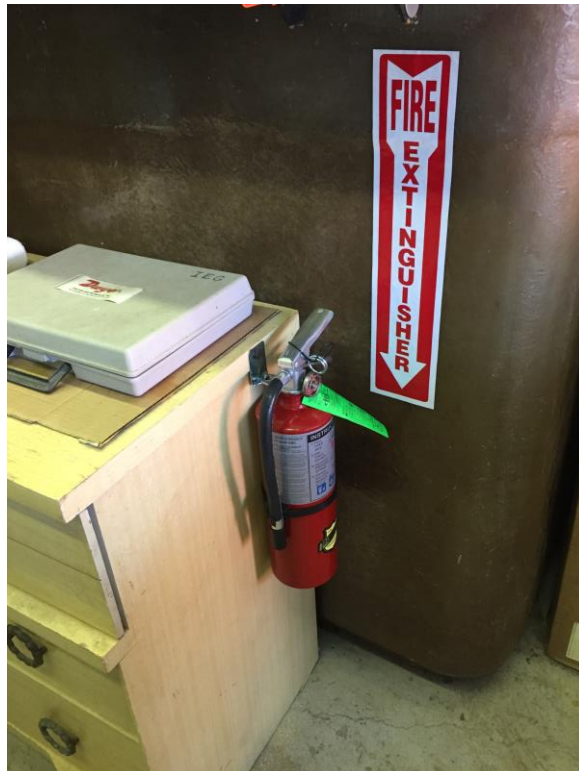
COMMERCIAL FIRE EXTINGUISHER INSTALLED IN FRONT OF EQUALIZATION TANK
