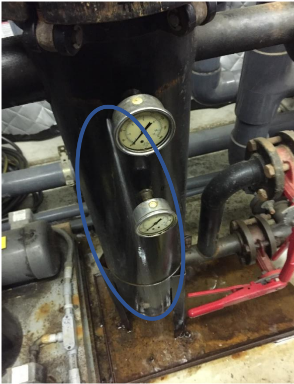
BEFORE REPAIR: LEFT BAG FILTER HOUSING LEAKING
