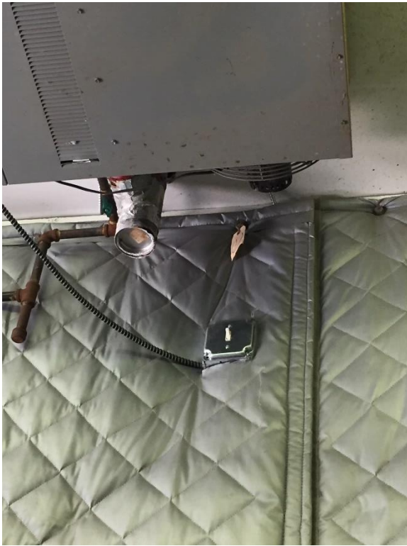
ELECTRICAL SWITCH BOX INSTALLED IN NORTH WALL FOR ROOM HEATER
