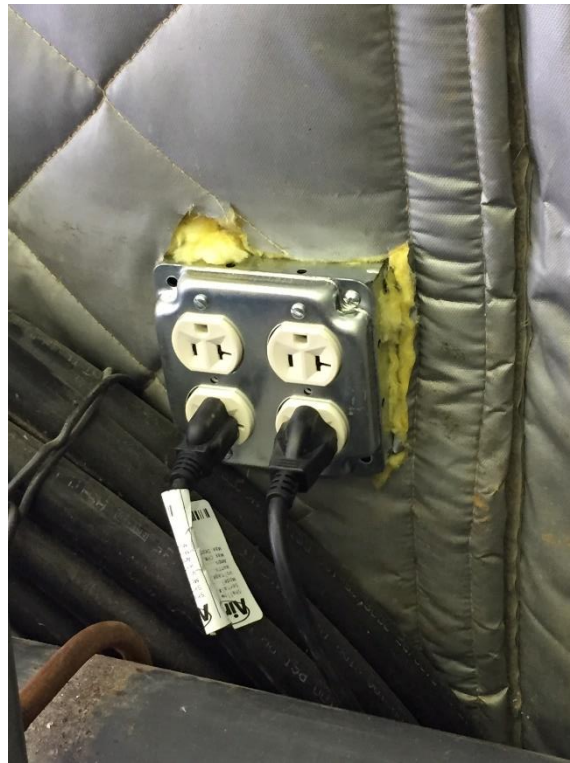
ELECTRICAL OUTLET INSTALLED IN NORTH WALL FOR AIR SPARGER PUMPS AND OTHER USE (insulation to be covered with duct tape)
