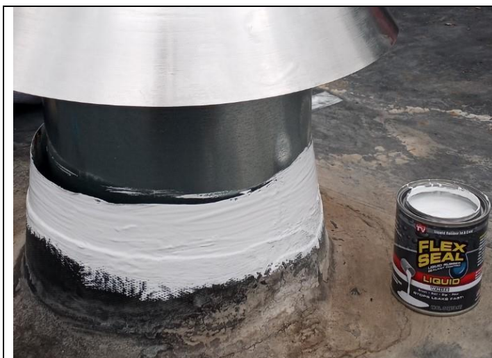
4. A new pipe was installed and sealed
