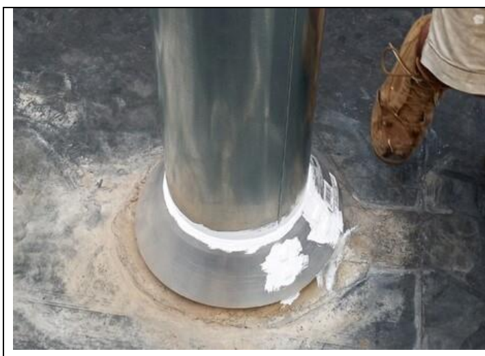
6. Finally the rain guard is sealed
