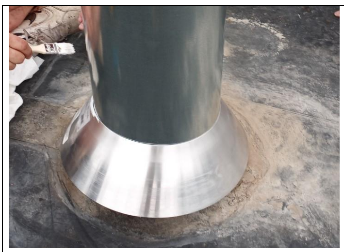
5. A rain guard was fitted into place
