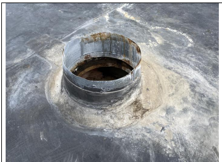
3. After cutting away the corroded part of the stack
