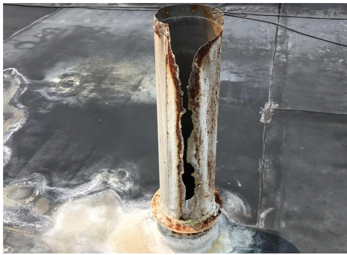
1. The old corroded Air Stripper exhaust stack on the roof
