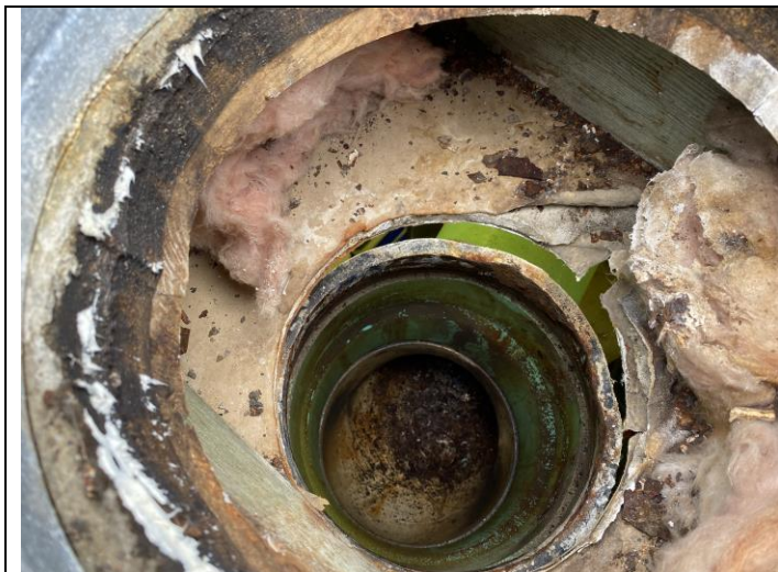
2. View down the exhaust after the stack was removed
