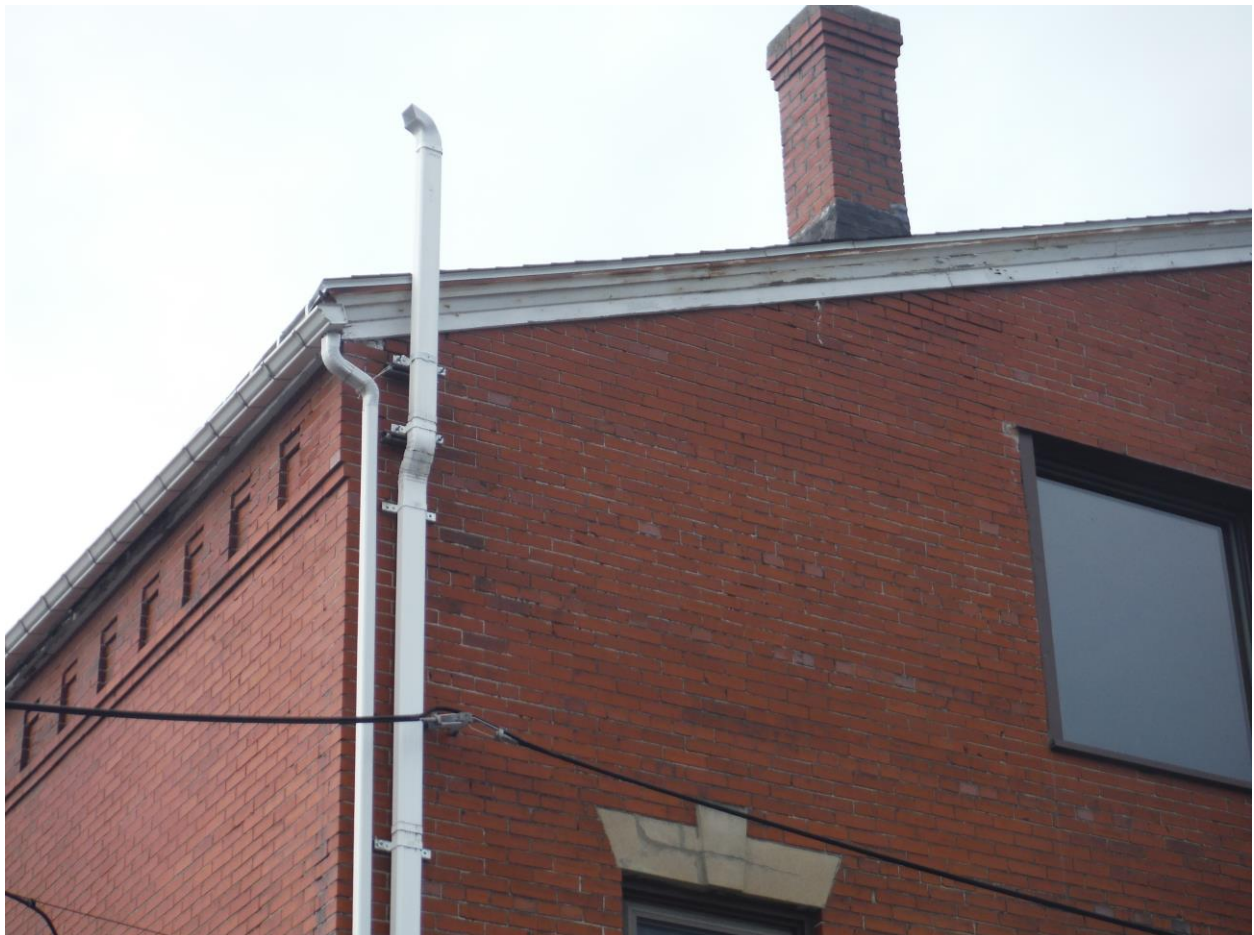
The top section was reinstalled with a new cap and bracket
