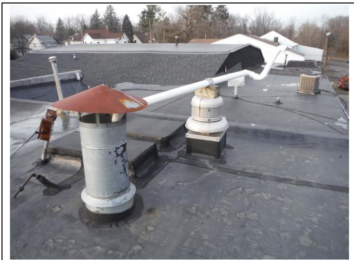
1. View of Treatment Room vent, SVE Exhaust Pipe and Fan
