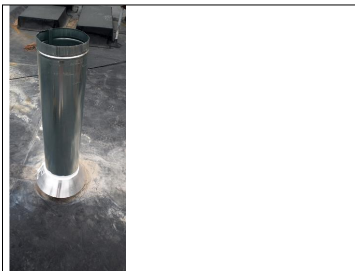
6. New Air Stripper exhaust pipe
