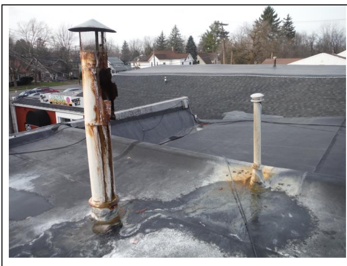
5. Old Air Stripper exhaust pipe and gas heater vent pipe
