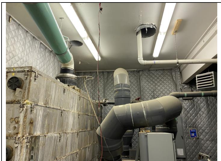
4. Exhaust fan vent and Treatment Room vent
