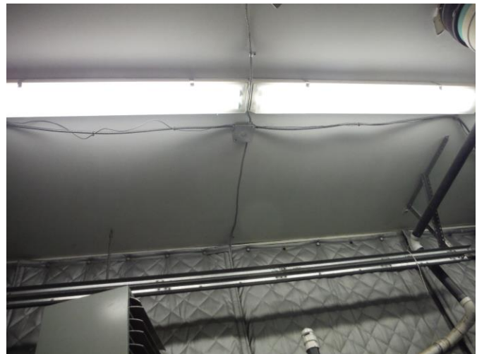
Junction Box mounted on Treatment Room ceiling. Loose BK wire was secured to the ceiling during the installment.
