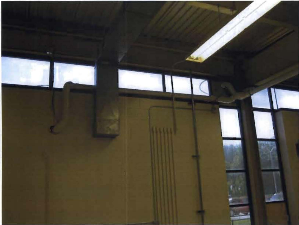
Looking east at junction of piping from suction point "East" (left), piping from suction points "South" and "North" (right) and exit of system piping to outside mounted fan.
