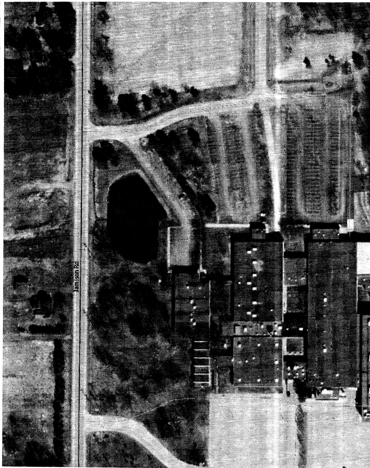
Figure 4. Moog Plant 11 Aerial Photograph
