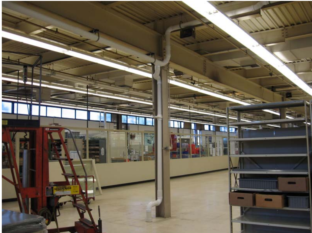
Looking southwest at routing of pipe from suction point “South” to system fan (left) and to suction point “North” (right).
