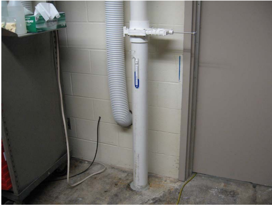
Looking west at suction point “East” with flow adjustment valve and manometer.
