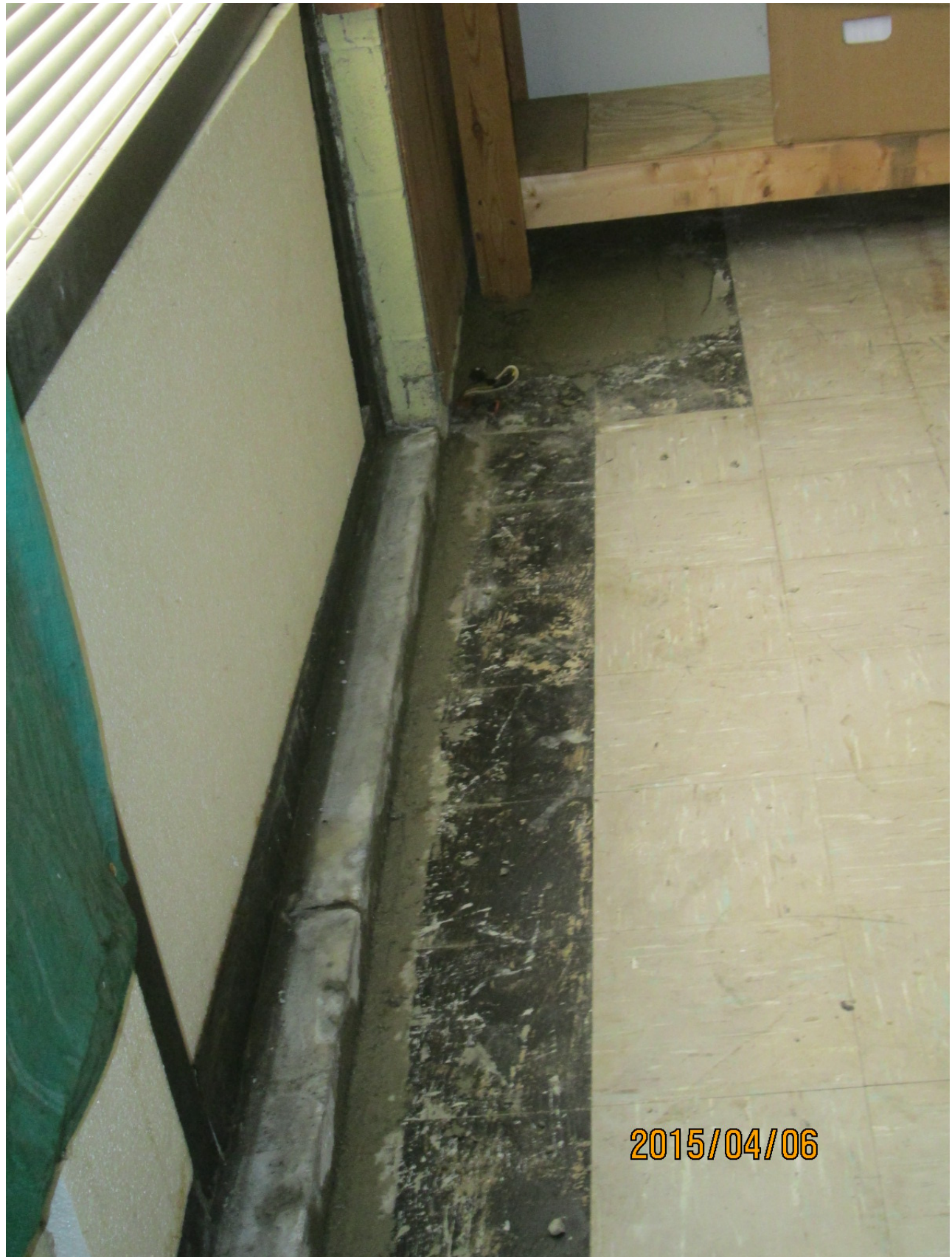
TYPICAL COMPLETED PERIMETER JOINT SEAL (Concrete mortar - east - south end of building)
