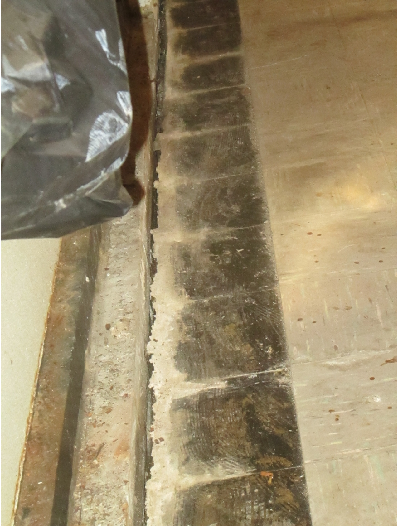
TYPICAL OPEN PERIMETER JOINT BEFORE SEALING (West - South end of building)
