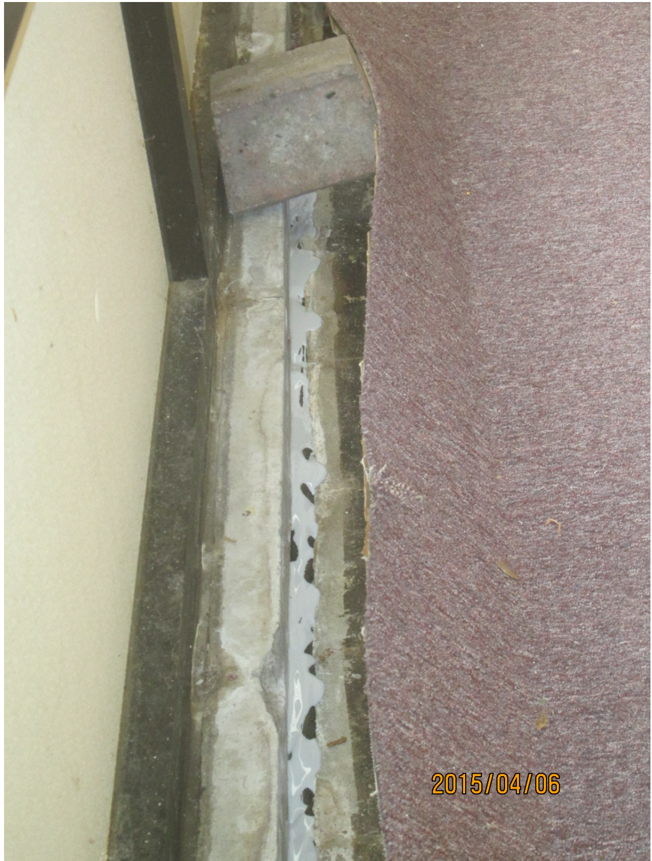
TYPICAL COMPLETED PERIMETER JOINT SEAL (Backer Rod/Urethane Sealant - east south end building)
