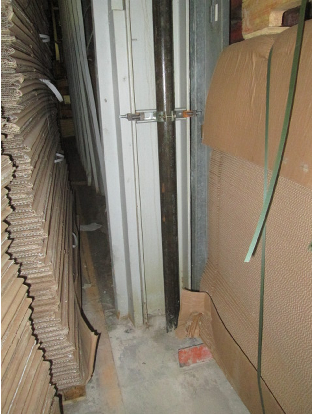
TYPICAL COMPLETED SUCTION DROP
