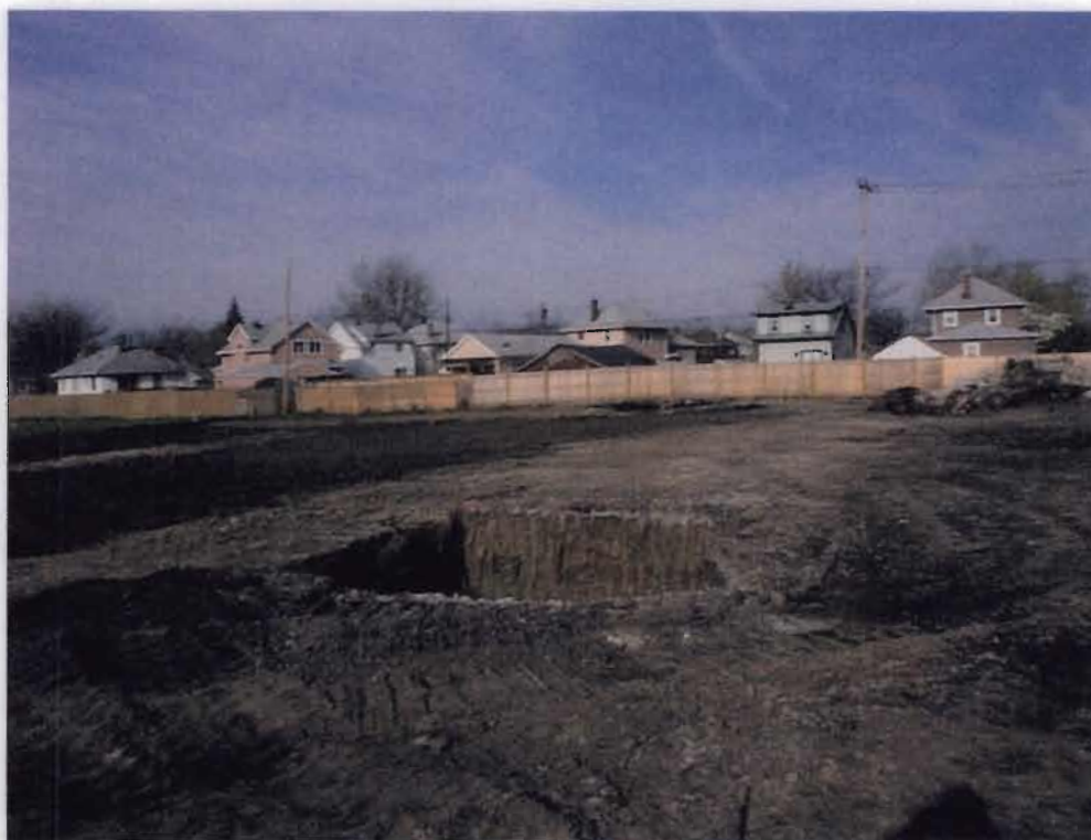
Lackawanna Foundry Site - PCB vault excavation in main building area.
