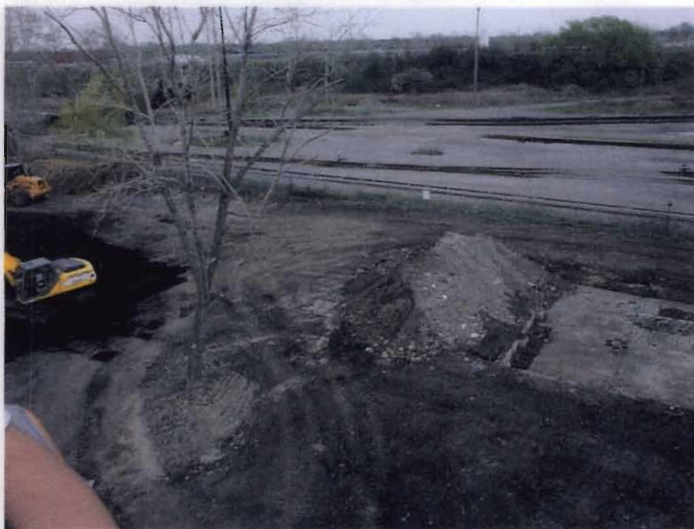
Lackawanna Foundry Site - PCB soil awaiting disposal in production area.
