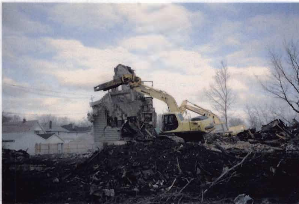
Lackawanna Foundry Site - Demolition of office building in main building area
