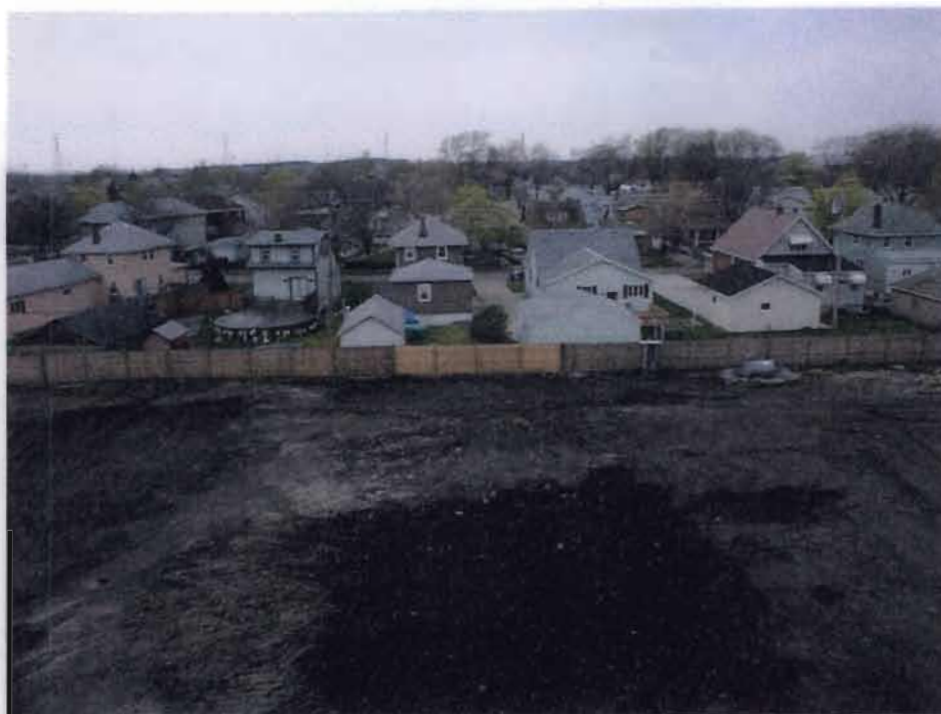
Lackawanna Foundry Site - Backfilling and grading prior to topsoil placement
