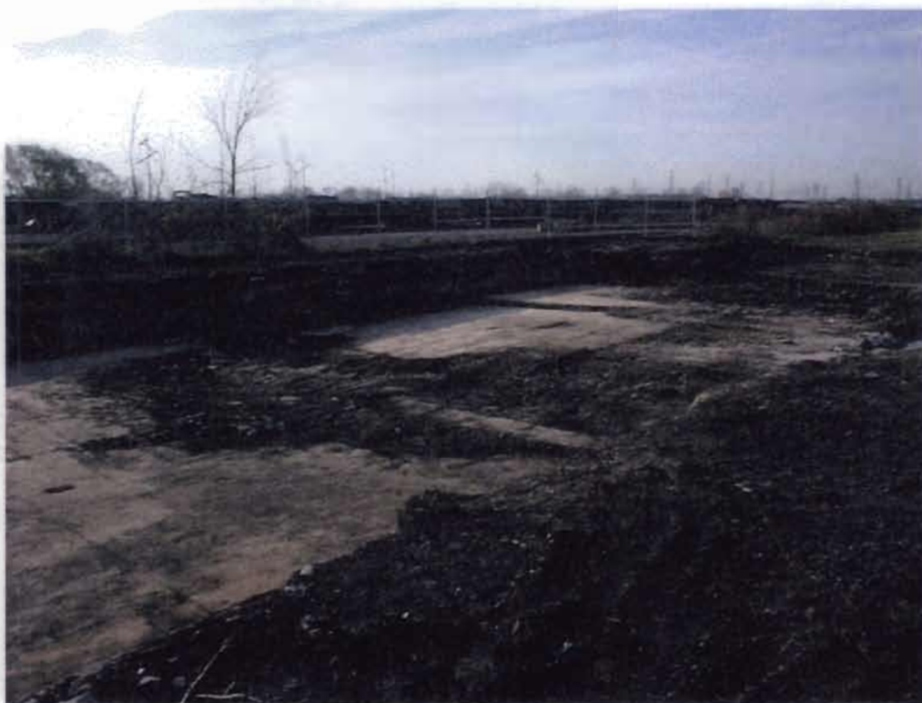
Lackawanna Foundry Site - (top bottom photo) Concrete pad in production building prior to backfill and topsoil placement.
