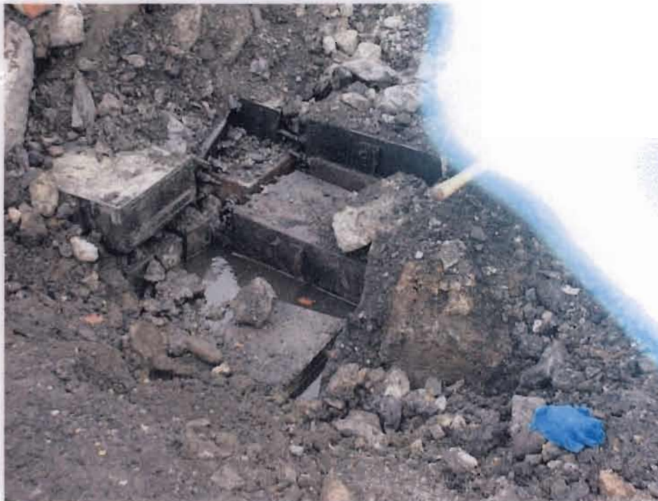
Lackawanna Foundry Site - PCB Capacitors in vault in main building area.
