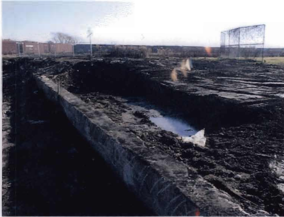
Lackawanna Foundry Site - Excavation of PCB vault area contaminated soils.
