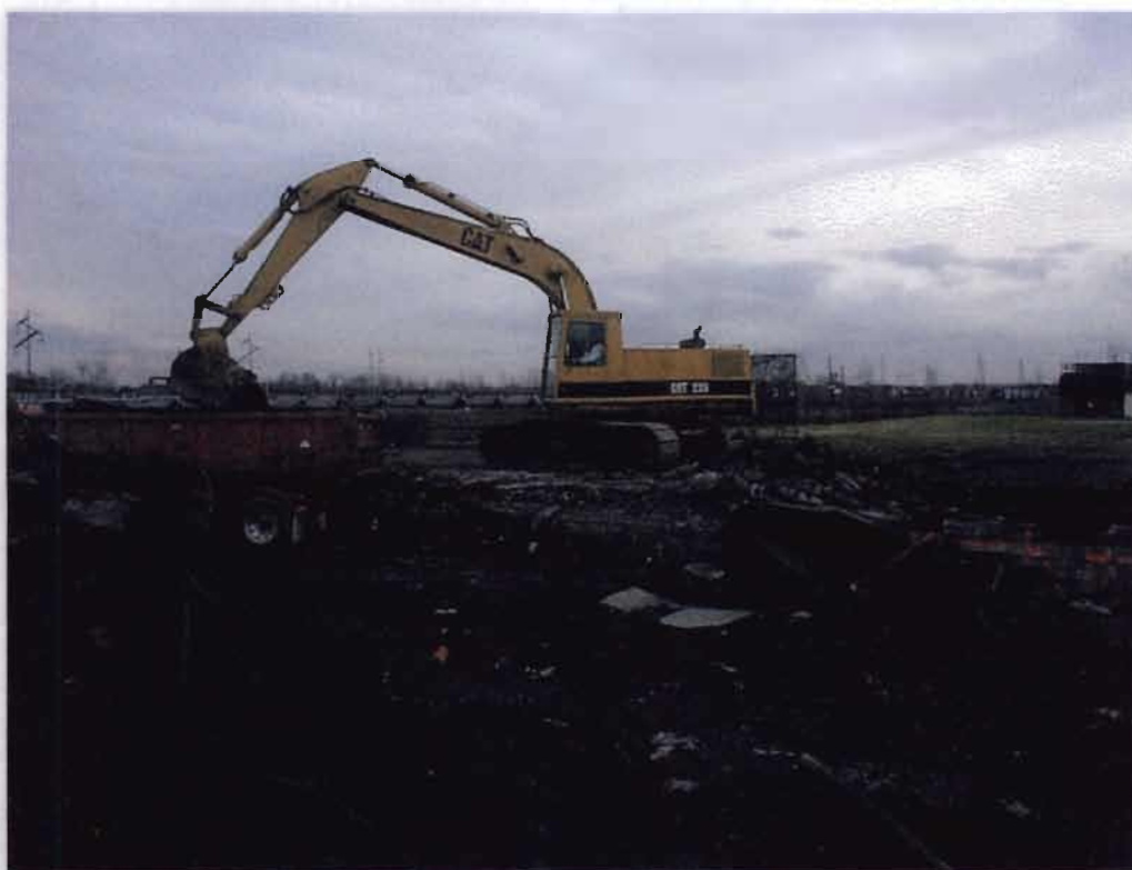
Lackawanna Foundry Site - Excavation of PCB Contaminated soils from PCB vault area
