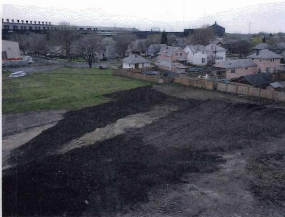
Lackawanna Foundry Site - Backfilling and grading site, prior to topsoil placement
