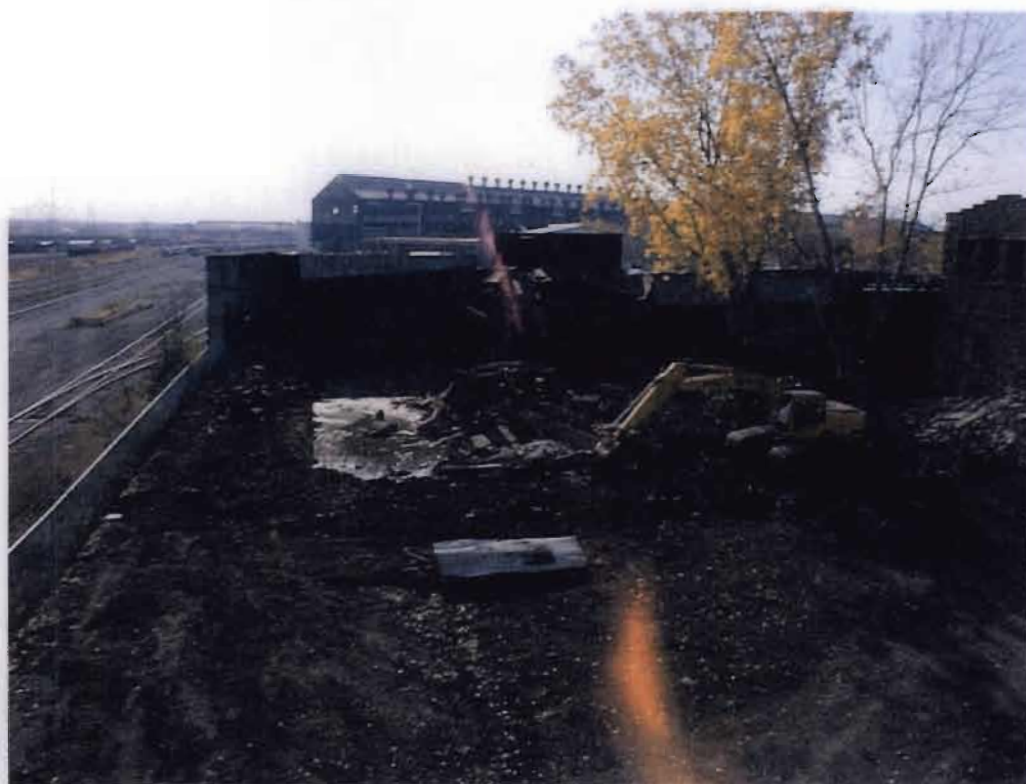
Lackawanna Foundry Site - Production building demolition
