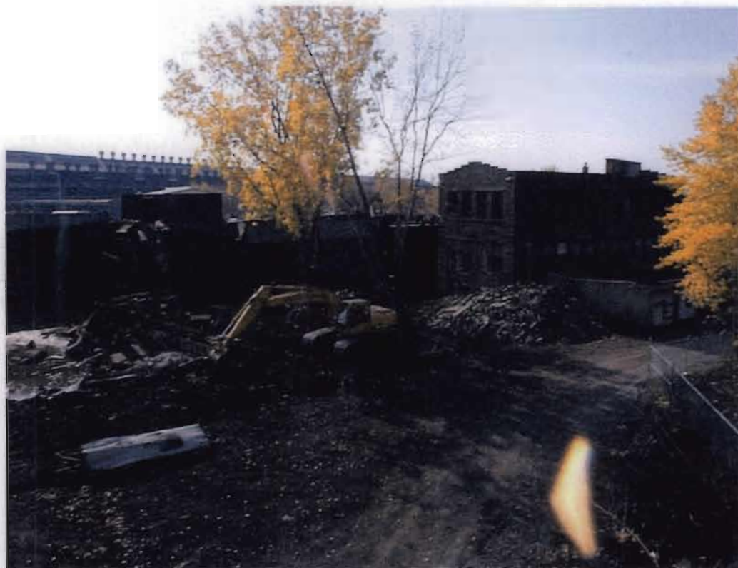
Lackawanna Foundry Site - Production building demolition
