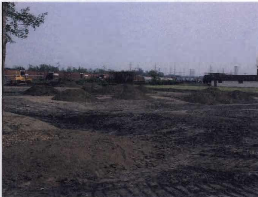
Lackawanna Foundry Site - (top and bottom) Final grading after topsoil placement.
