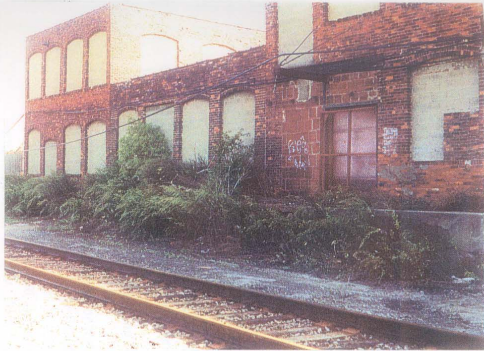
2. Looking northeast at the back of the Chem-Core building with railroad in foreground.
