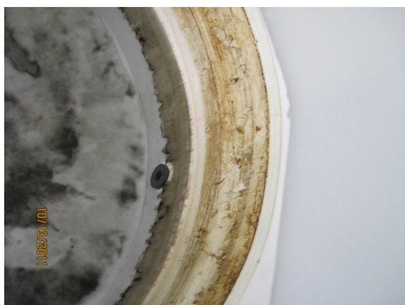
Interior of the equalization tank prior to powerwashing.
