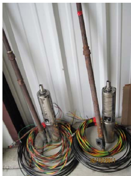
Well pumps, transducers, pitless adapters, and associated wiring staged within the system enclosure.
