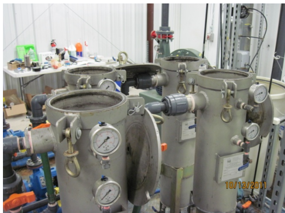
Bag filter housings drying subsequent to being drained and cleaned.
