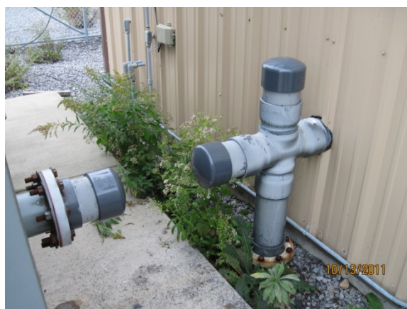
Capped and sealed Cat-Ox and vapor discharge stack piping.
