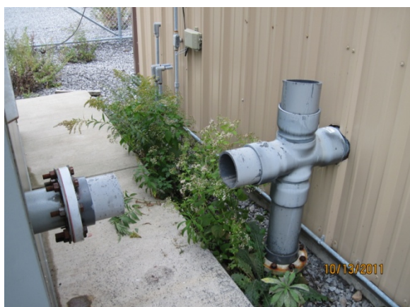
Disconnected Cat-Ox and vapor discharge stack piping prior to capping.
