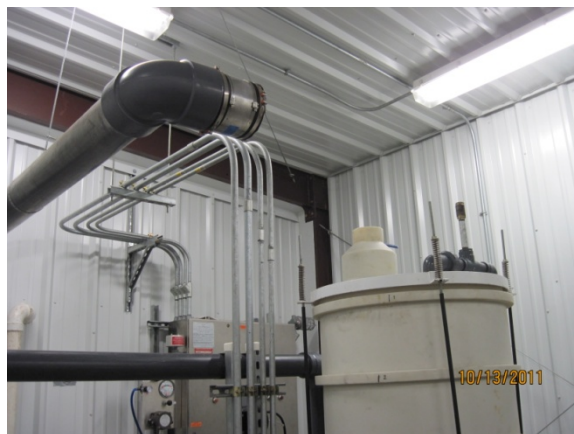
Effluent air line disconnected from cleaned air stripper unit.
