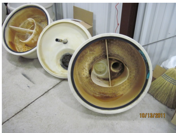
Air stripper trays drying in the system enclosure following powerwashing.
