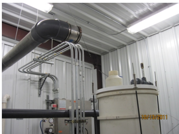
Vapor discharge piping disconnected from the cleaned and reassembled air stripper unit.
