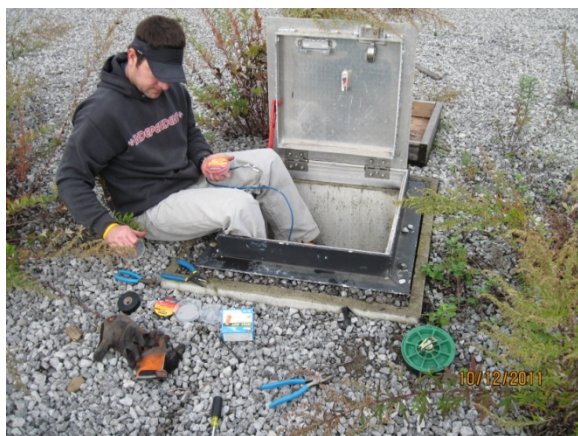
Weatherproofing remaining electrical lines within the WP-2 vault.
