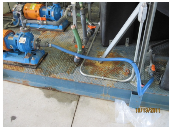
Plumbing setup used to drain remaining water from the equalization tank.
