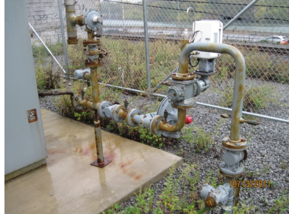
Cat-Ox natural gas service that has been disconnected by the utility provider.
