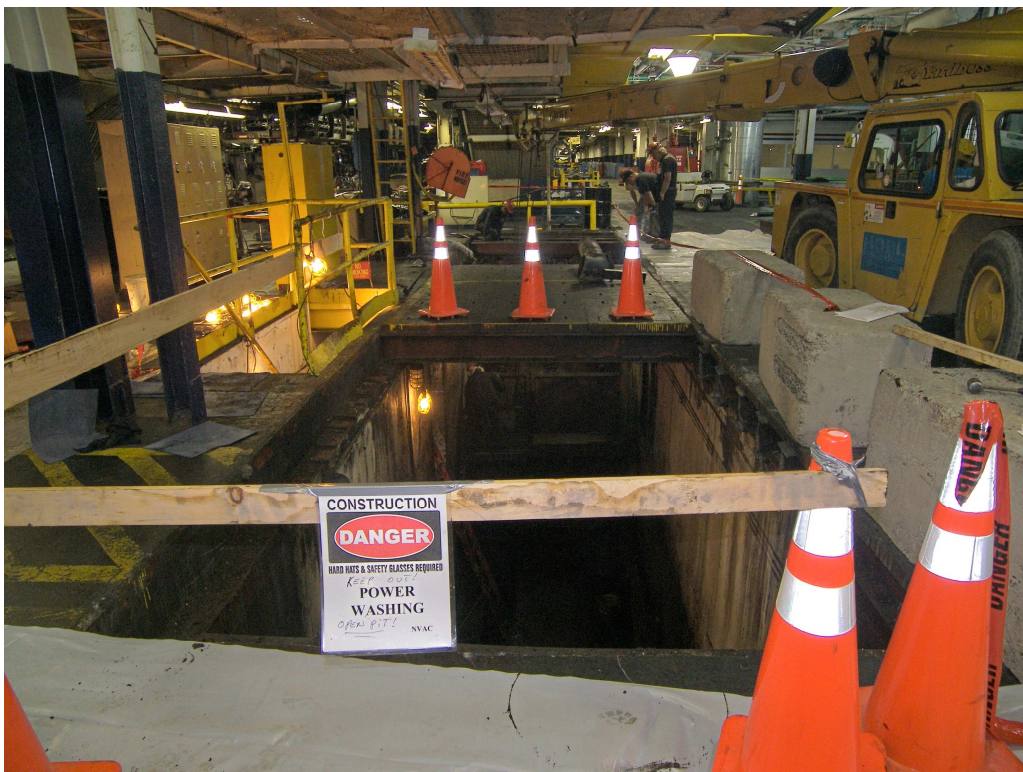
Picture 2 - Looking north across pit. Crew preparing to lift steel debris.
