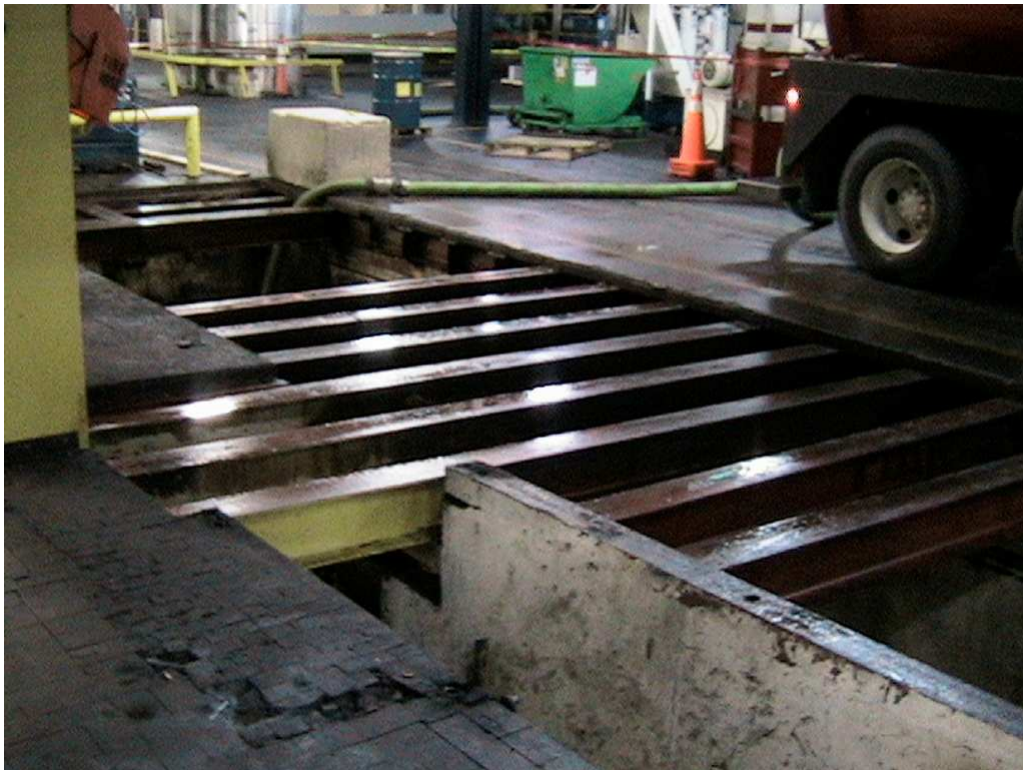
Picture 6 – Looking northeast across pit. Removal of washwaters in progress.
