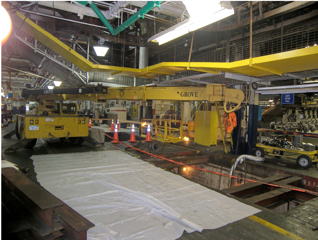
Picture 1 - Looking southwest toward pit. Laydown area for steel debris.
