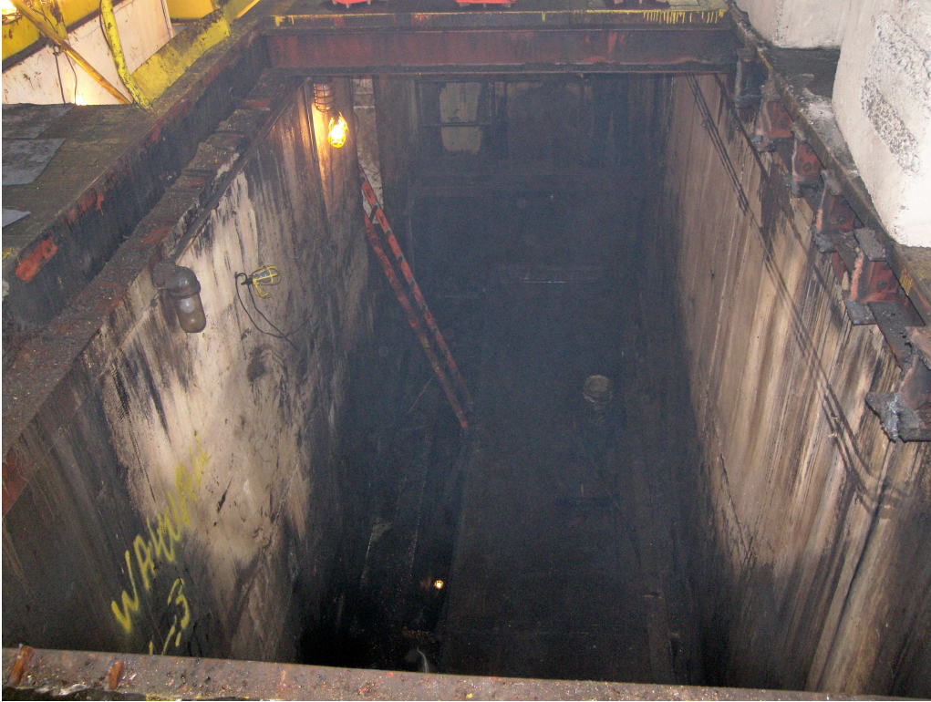
Picture 3 – Looking north into pit. Cleaning in progress.
