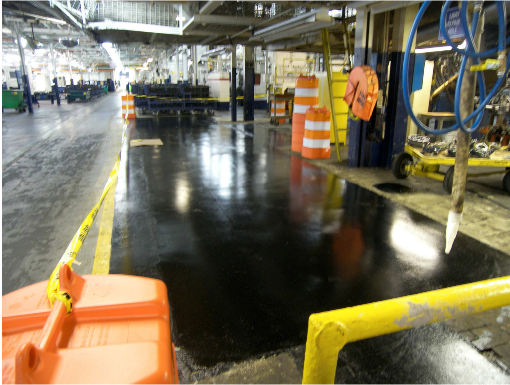
Picture 7 - Looking south across finished pit.
