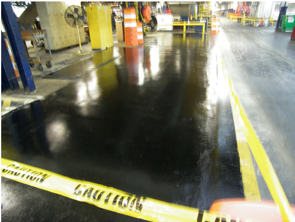
Picture 8 - Looking north across finished pit.
