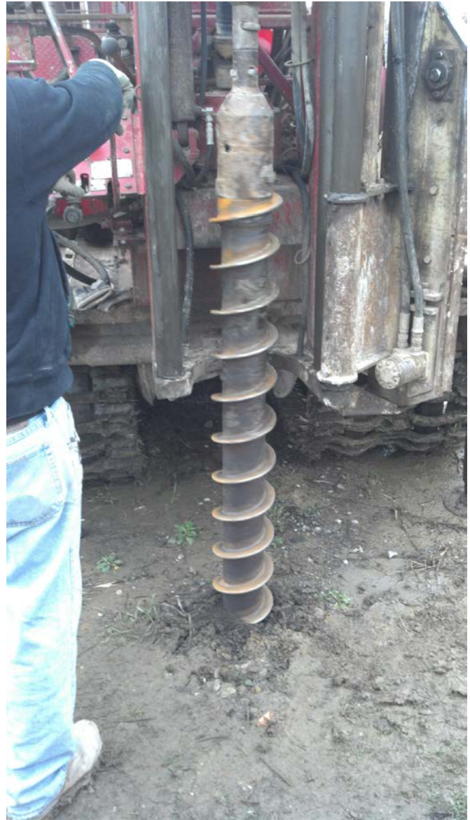
View of hollow stem augers drilling at MW-03A.
