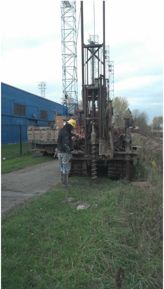
GeoLogic drilling MW-08.
