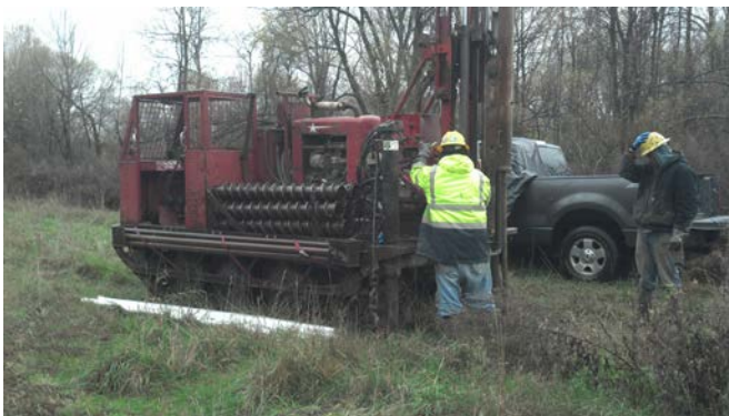
View of GeoLogic drilling MW-05.
