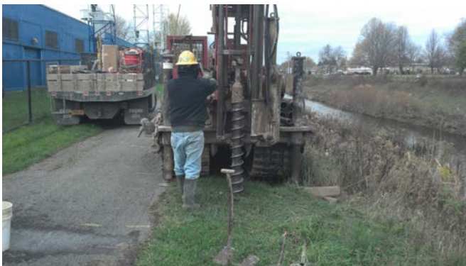
View of GeoLogic drilling MW-08.
