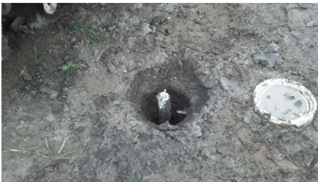
View of MW-03A PVC riser installed.
