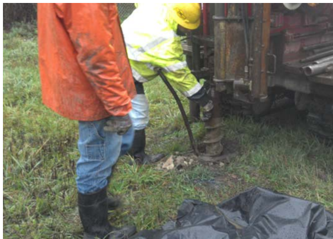
View of hollow-stem augers and drill head assembly at MW-02A.
