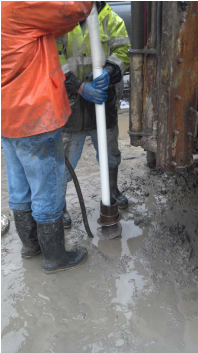
View of GeoLogic installing MW-05 well materials.
