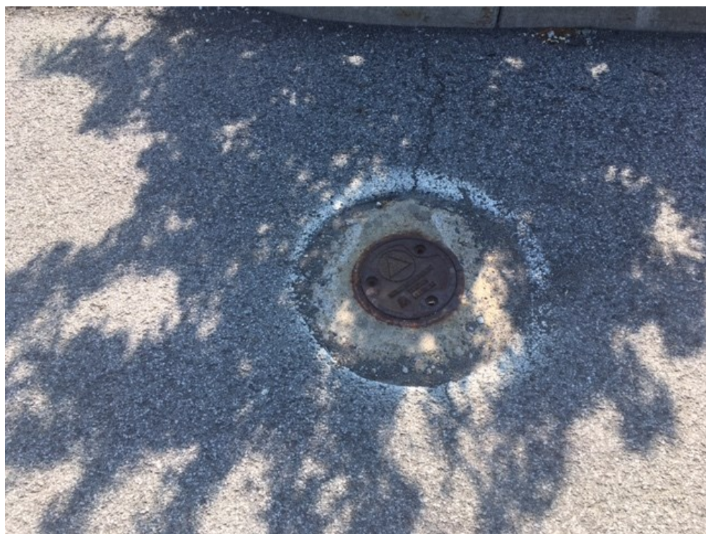
Photo #6: MW-1S,D. EPSVT recommends monitoring well repair work to be done.
