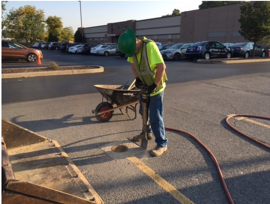
Photo #1: Well Abandonment Activities September 25, 2017 through September 28, 2017.
