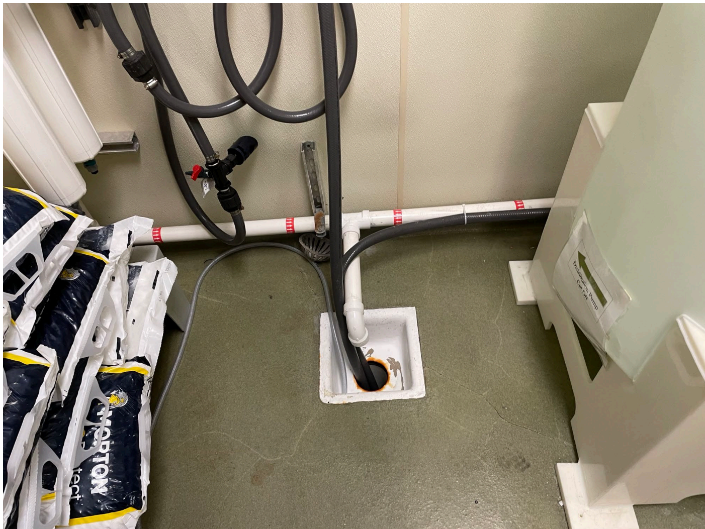
Floor drain in water treatment room inside US Renal Care building.
