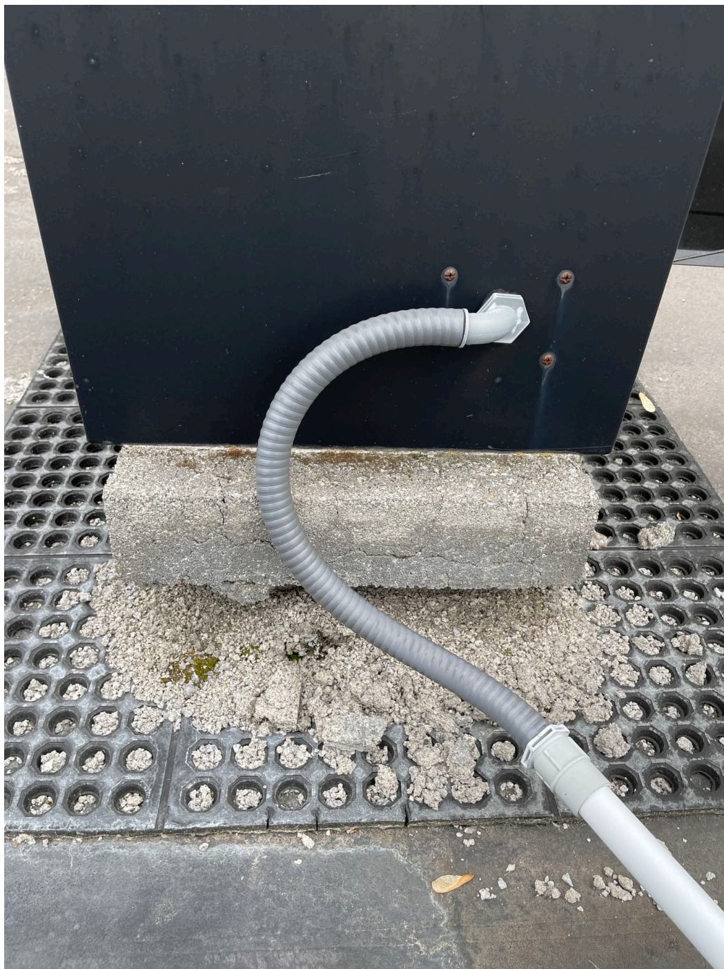
Crumbling cinder blocks supporting SDS enclosure.
