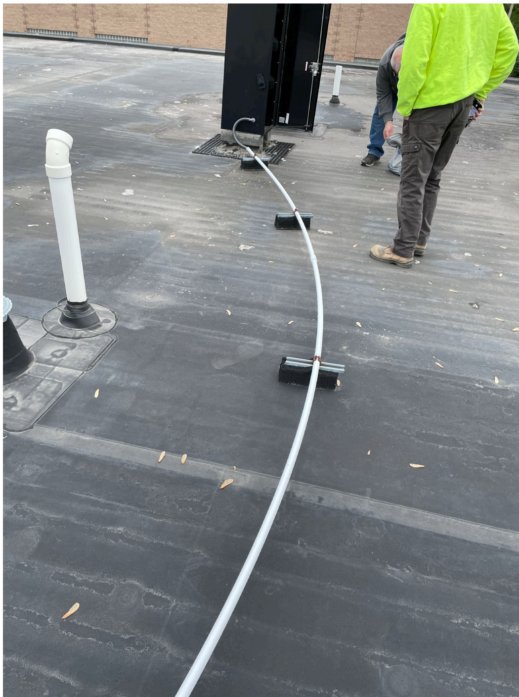
Electrical conduit leading to SSDS enclosure.
