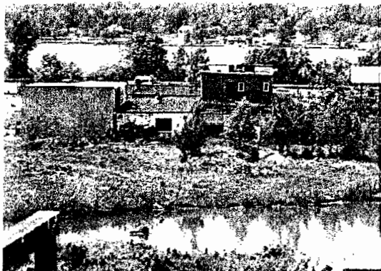
Site building looking northwest
