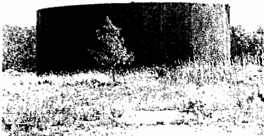
5,000,000-gallon AST on northwest portion of Site
