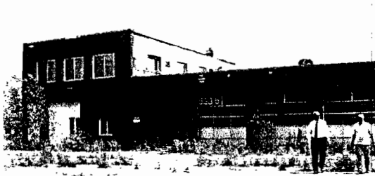
Site building looking southeast
