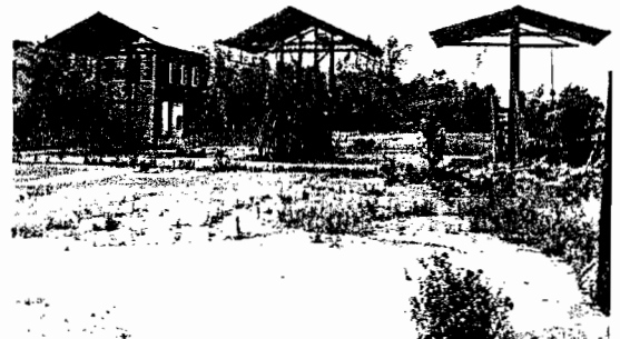
Truck racks on northwestern portion of the Site looking southwest
