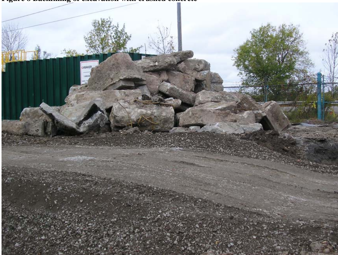
Figure 9 Contaminated concrete to be broken and disposed
