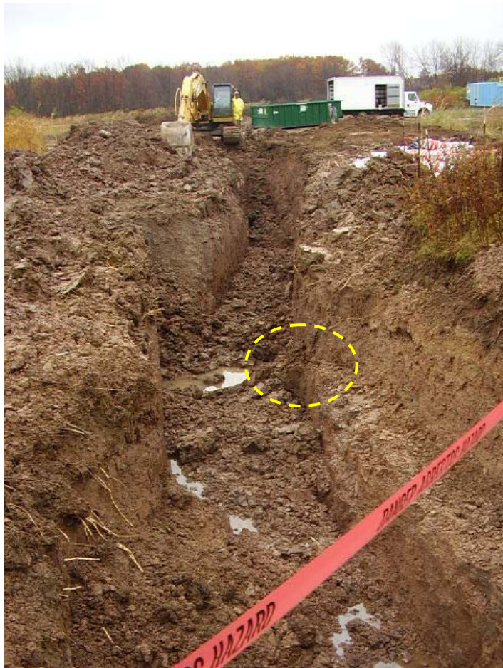
Location of unknown clay pipe with suspected petroleum contamination
