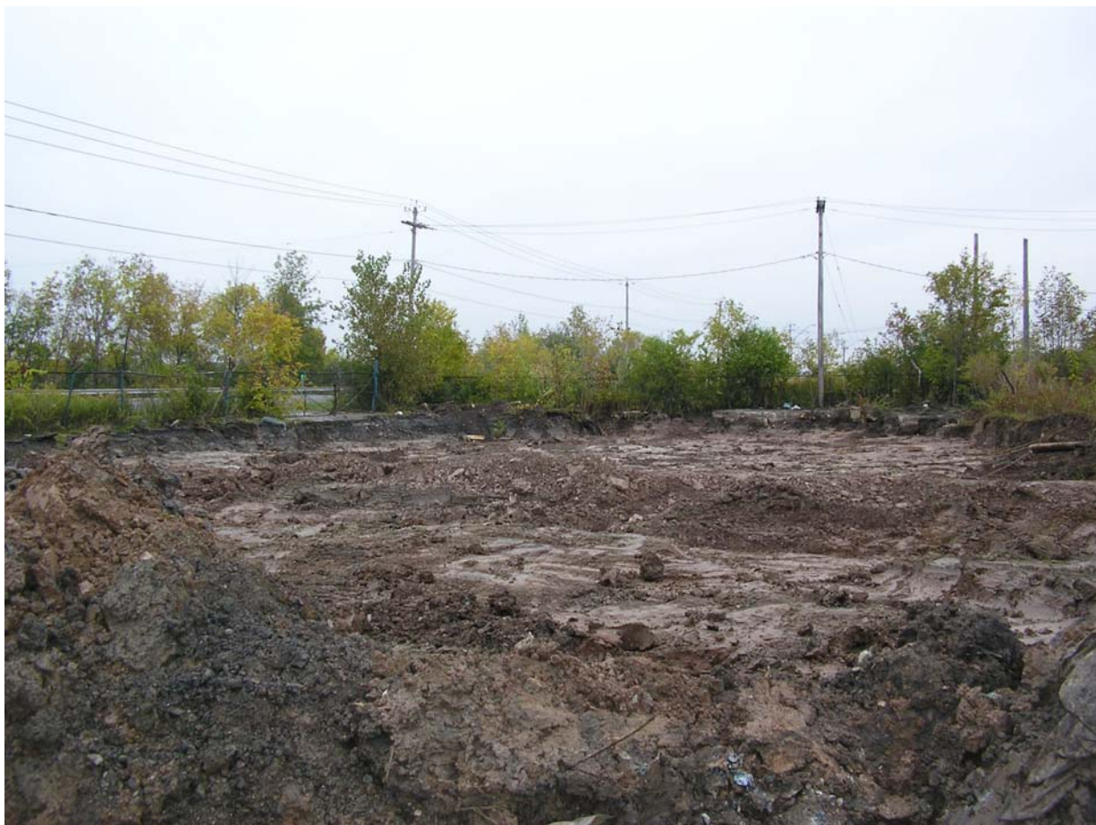
Figure 5 Berm created to prevent oily liquids from migrating east
