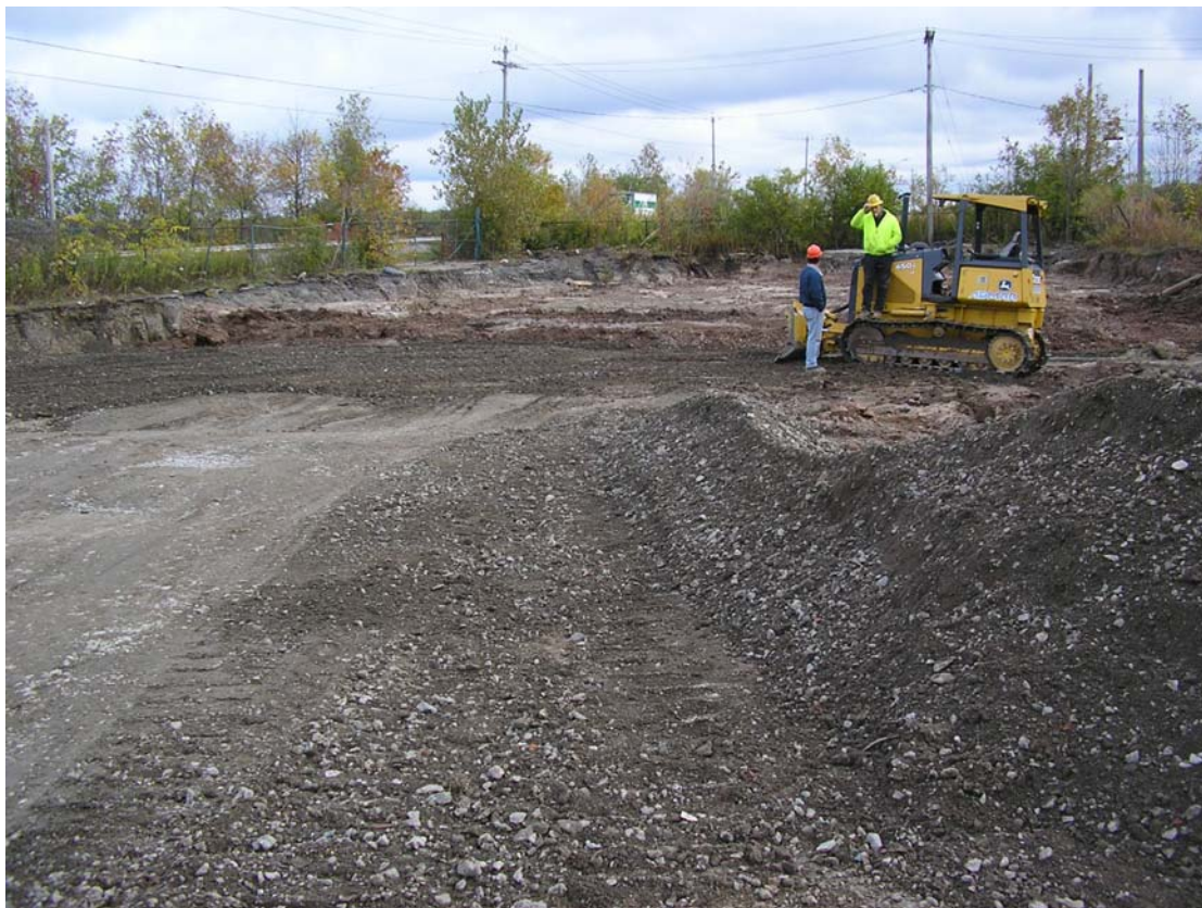
Figure 8 Backfilling of excavation with crushed concrete
