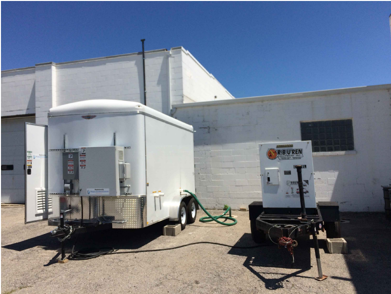
PILOT STUDY PHOTOGRAPH SHOWING SVE TRAILER AND DIESEL GENERATOR (green tubing connected to extraction well SVE-1)
