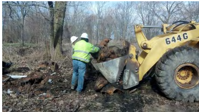
Hand loading crushed drums into the clamshell loader.
