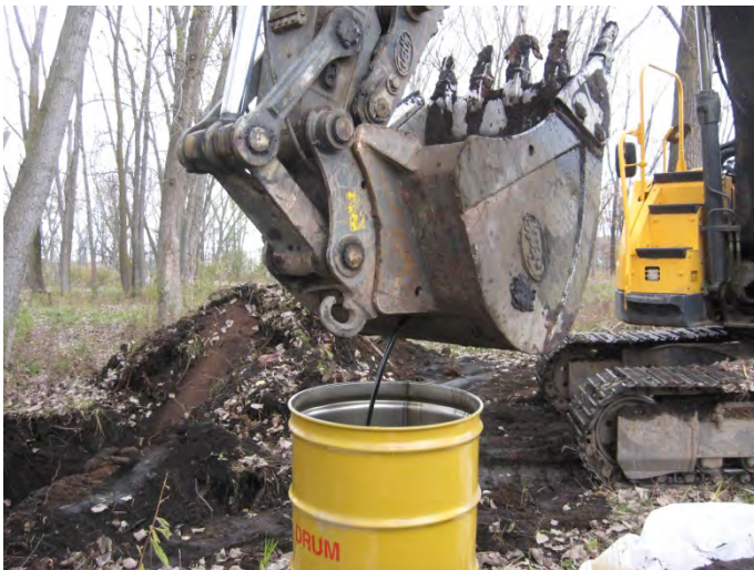
Draining drum contents into overpack at TP-06.
