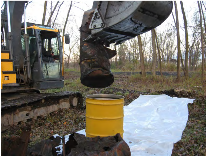
Placing drum into overpack at TP-07.
