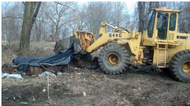
Crushing drums prior to loading into roll offs in AOC04.
