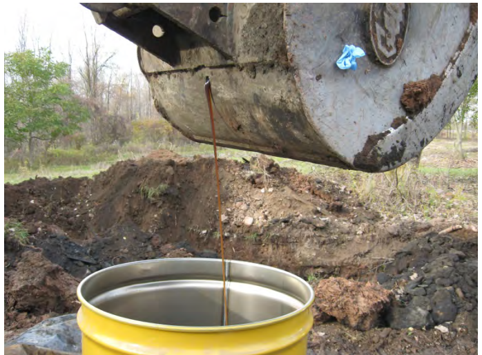
Emptying drum contents into an overpack at TP-21.
