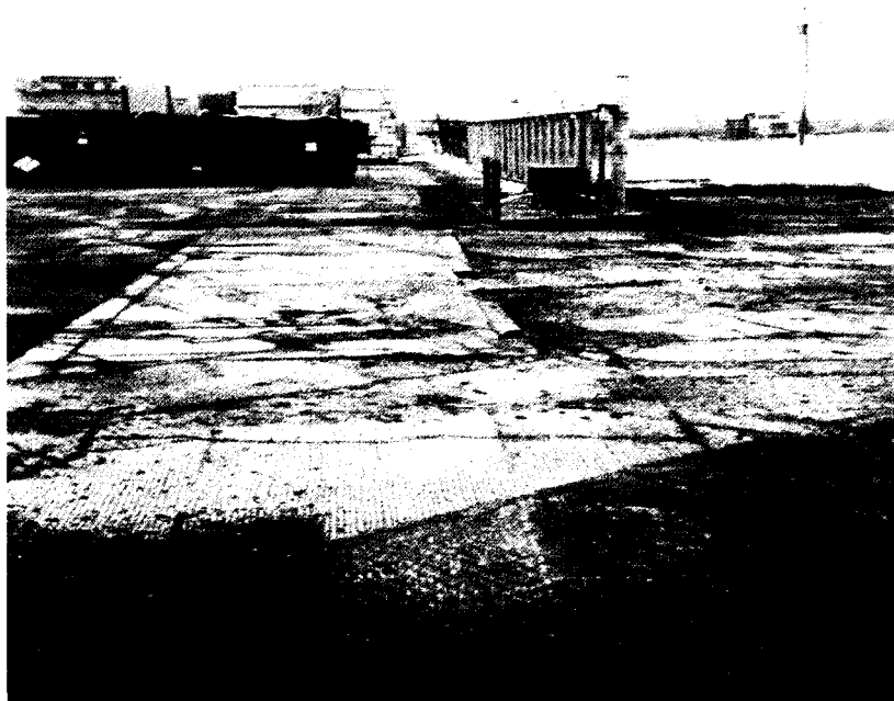
Photo 15: Asphalt near entrance gate and pressure plate removed and segregated.
