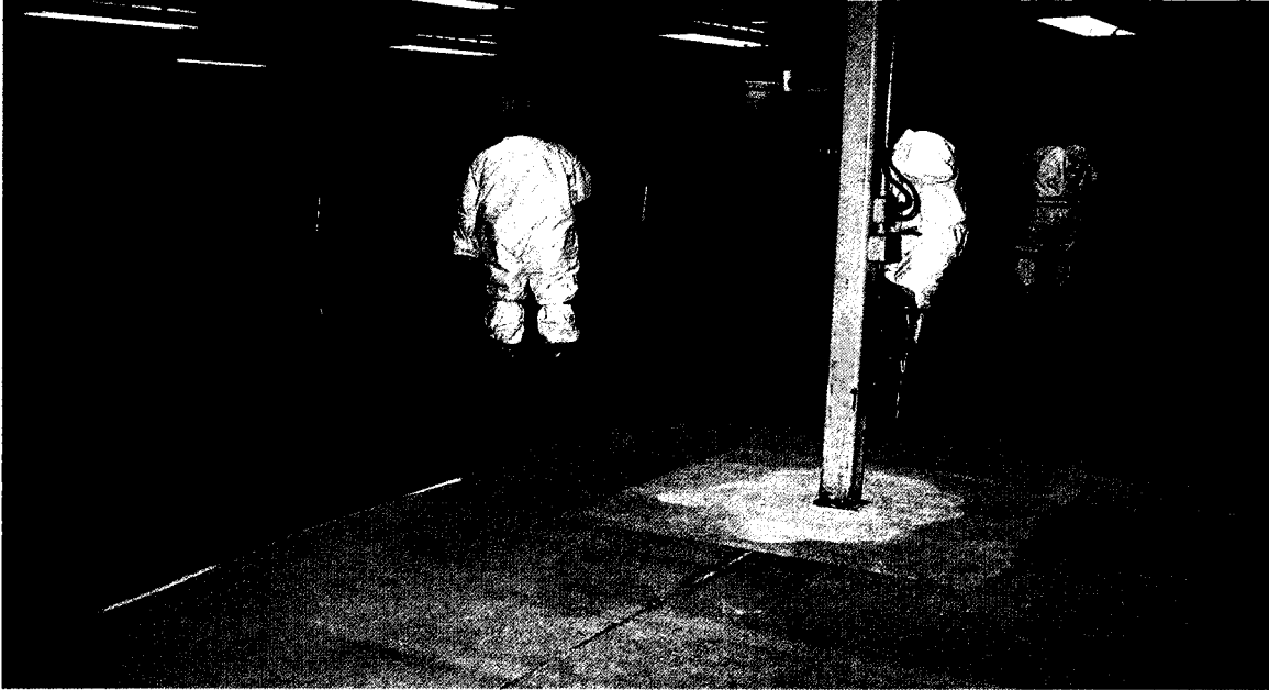
Photo 7: Applying primer to prepared surface.
