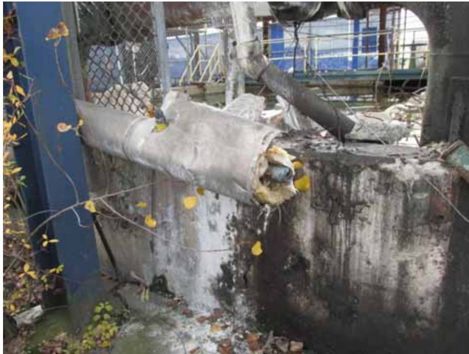
Photo 13: 11/8/13 – Metal jacket with grey caulk seams (non-ACM) over fiberglass insulation with silver backing (non-ACM) in grid R4.
