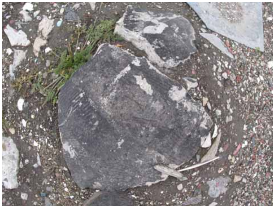
Photo 25: 11/11/13 – Black coating on brick (non-ACM).
