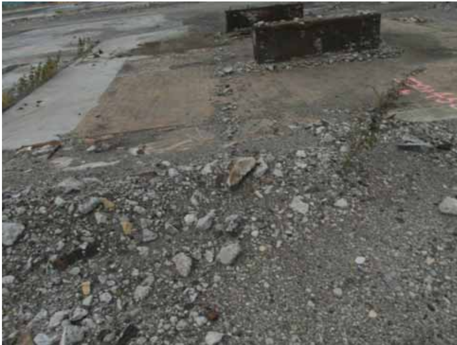
Photo 8: 11/6/13 – Miscellaneous debris with ACM roofing material in Grid G10.
