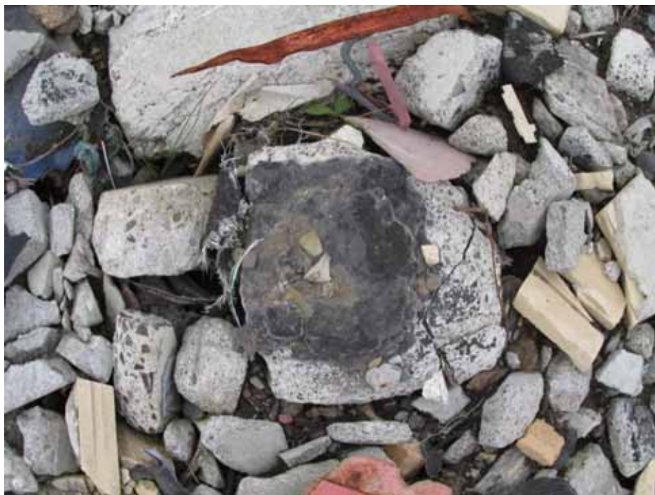
Photo 21: 11/11/13 – Misc. roofing debris (ACM).
