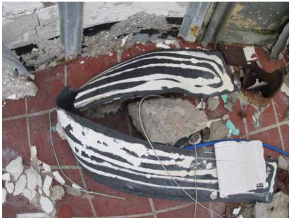
Photo 31: 11/11/13 – Black cove base molding & mastic (non-ACM).
