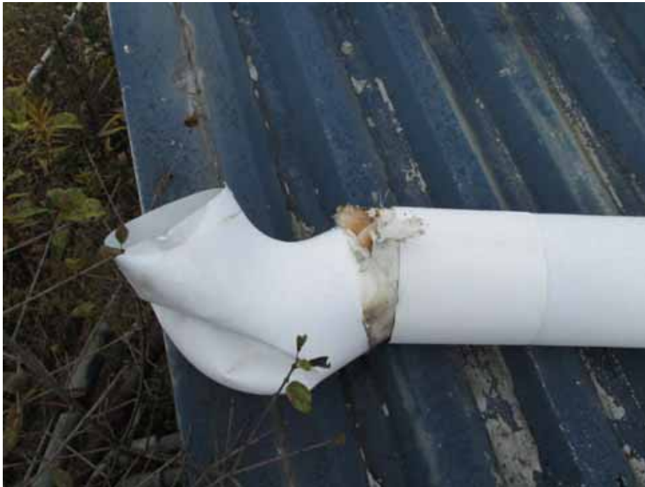
Photo 16: 11/8/13 – White fiberglass backing (non-ACM) in grid S4.
