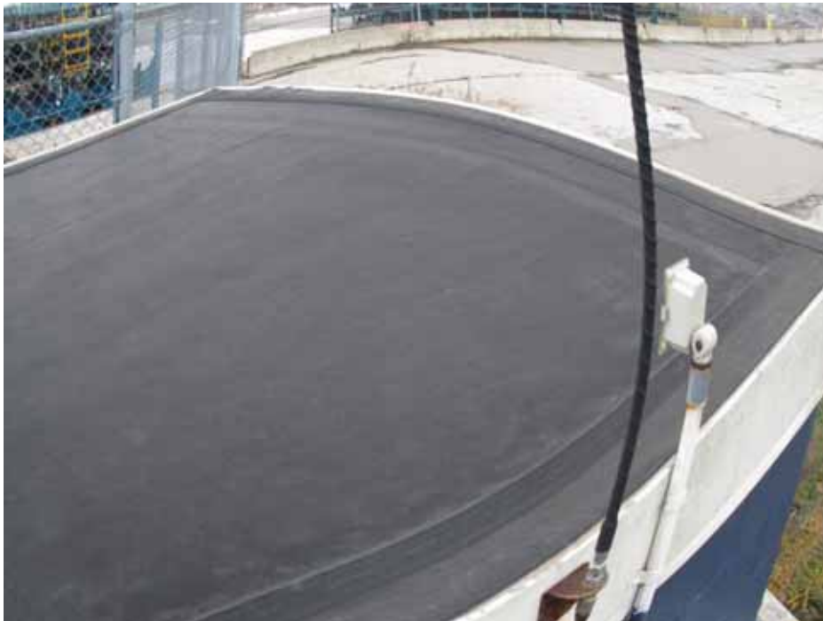
Photo 20: 11/8/13 – Rubber roof membrane (non-ACM) over shed in grid S12.
