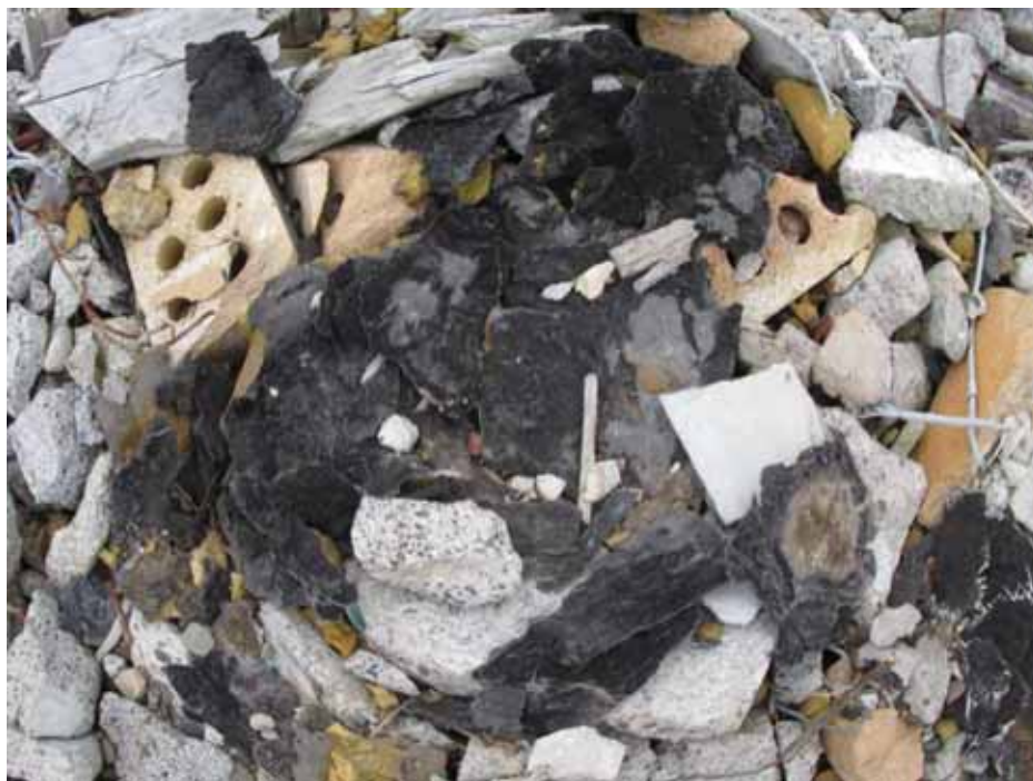
Photo 24: 11/11/13 – Black built up roofing (ACM).
