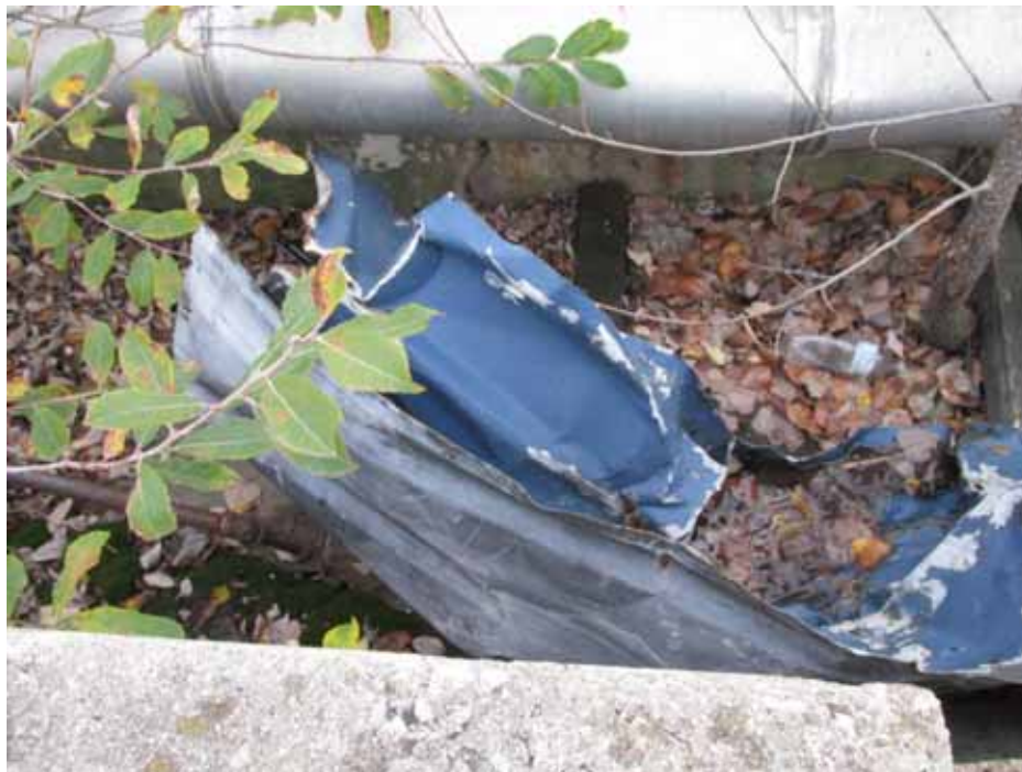
Photo 11: 11/7/13 – Galbestos (ACM) coating on blue painted metal in grid R5.
