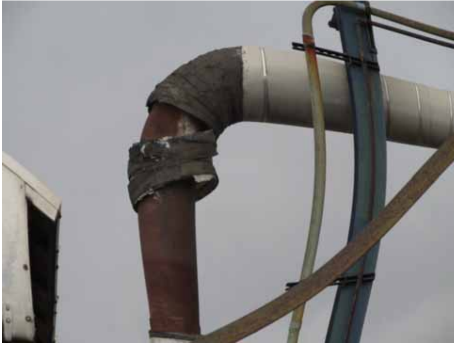
Photo 19: 11/8/13 – Black wrapped pipe insulation (PACM) in grid R4 (inaccessible).
