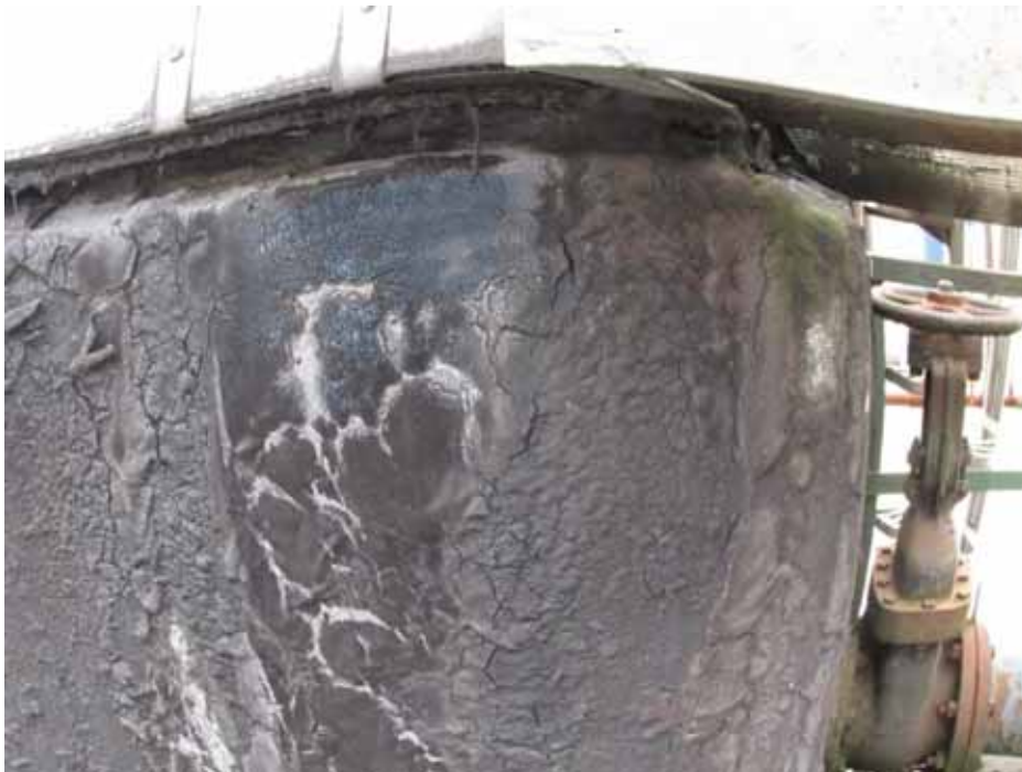
Photo 18: 11/8/13 – Black coating over fiberglass (non-ACM) on tanks in grid S5.
