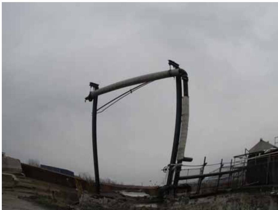
Photo 45: 11/11/13 – Black wrapped pipe insulation (PACM) in grid R4 (inaccessible).
