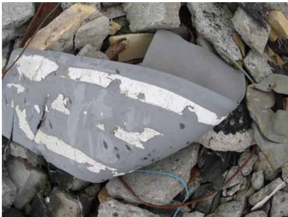
Photo 23: 11/11/13 – Brown cove base molding and mastic (non-ACM) in grid A4.
