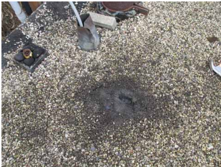
Photo 14: 11/8/13 – Black built up roofing (ACM) in grid S4.
