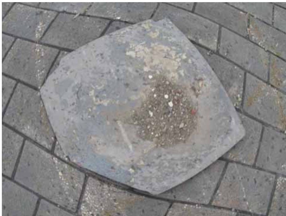
Photo 26: 11/11/13 – 12' X 12' grey floor tile (non-ACM).
