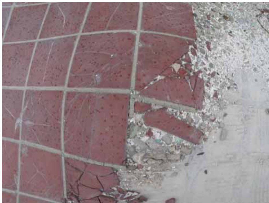
Photo 29: 11/11/13 – Terracotta tile mastic (ACM) and grout (non-ACM).
