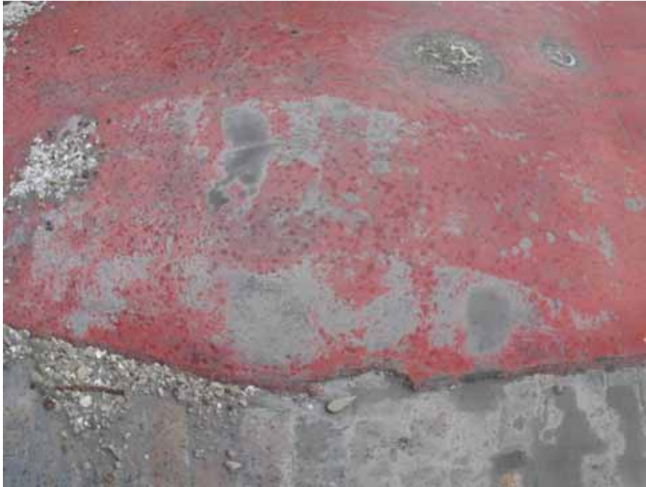
Photo 35: 11/11/13 – Red thick floor coating (non-ACM) in grid A8.
