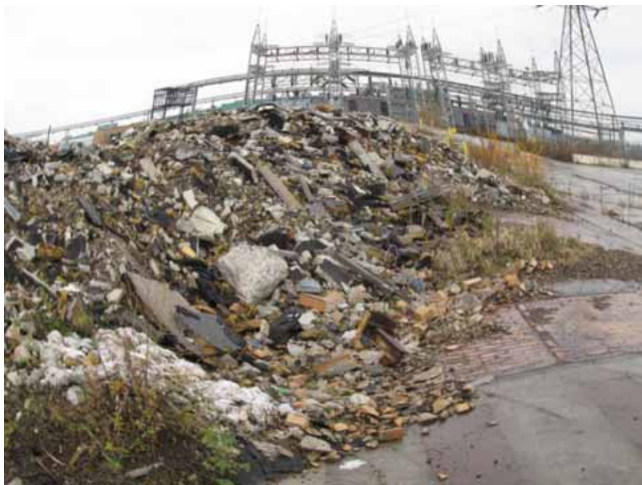
Photo 43: 11/11/13 – Debris pile on southwest end of grids T5-T8 (not surveyed).
