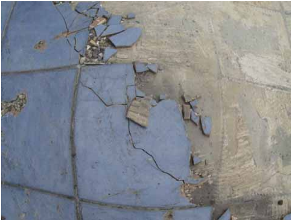
Photo 36: 11/11/13 – 12' X 12' Blue ceramic tile mastic and grout (non-ACM) in grid A9.
