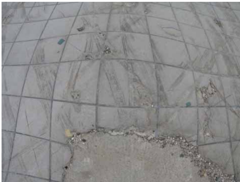
Photo 34: 11/11/13 – Gray floor tile and mastic (non-ACM) in grid A3.
