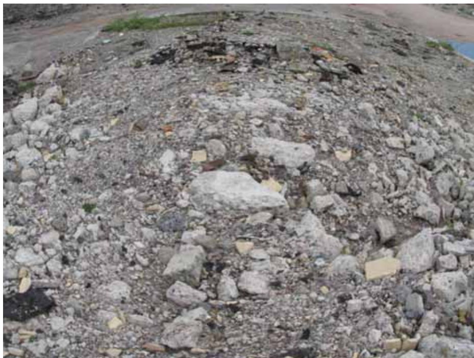
Photo 38: 11/11/13 – Miscellaneous debris with ACM roofing material throughout (typical).
