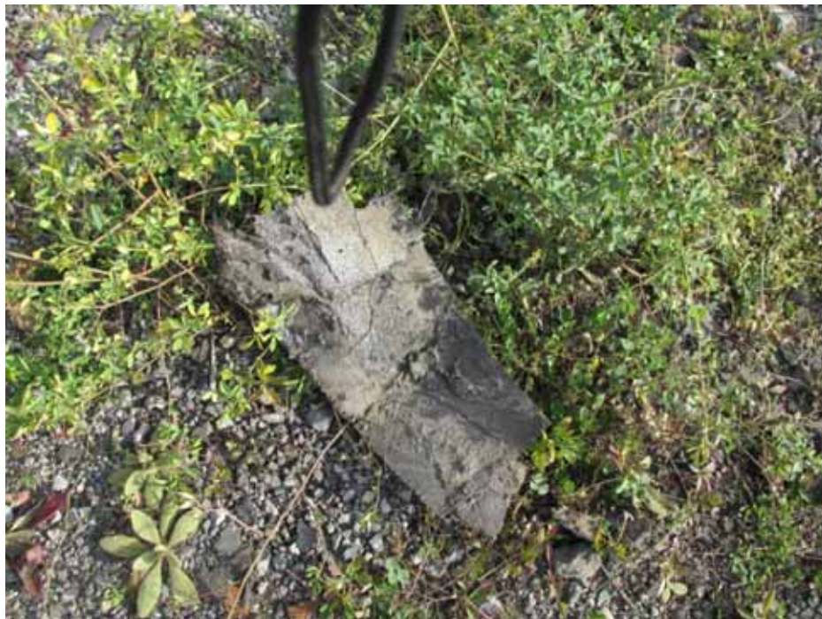
Photo 2: 11/5/13 – Gray roof shingle (ACM-typical).
