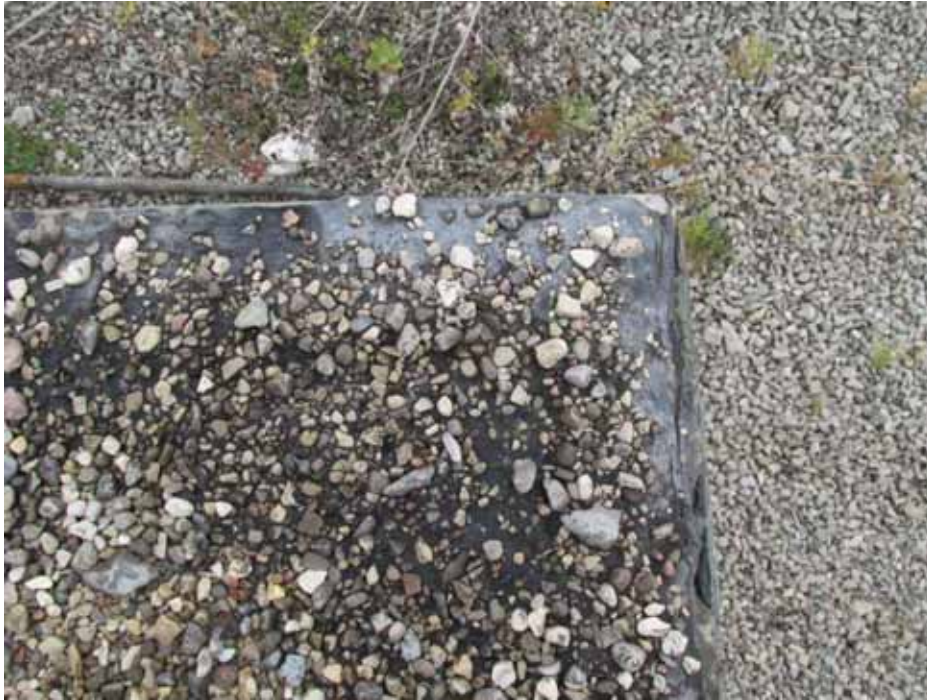
Photo 17: 11/8/13 – Grey perimeter flashing (ACM) in grid S4.
