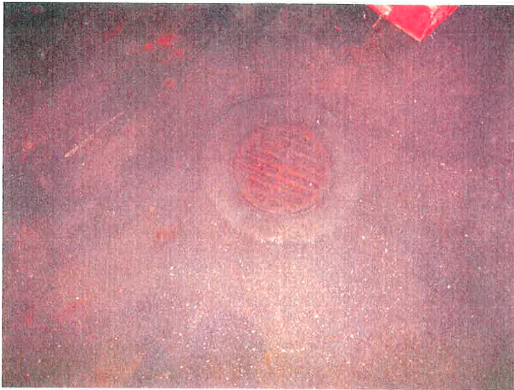
Sealed floor drain.
