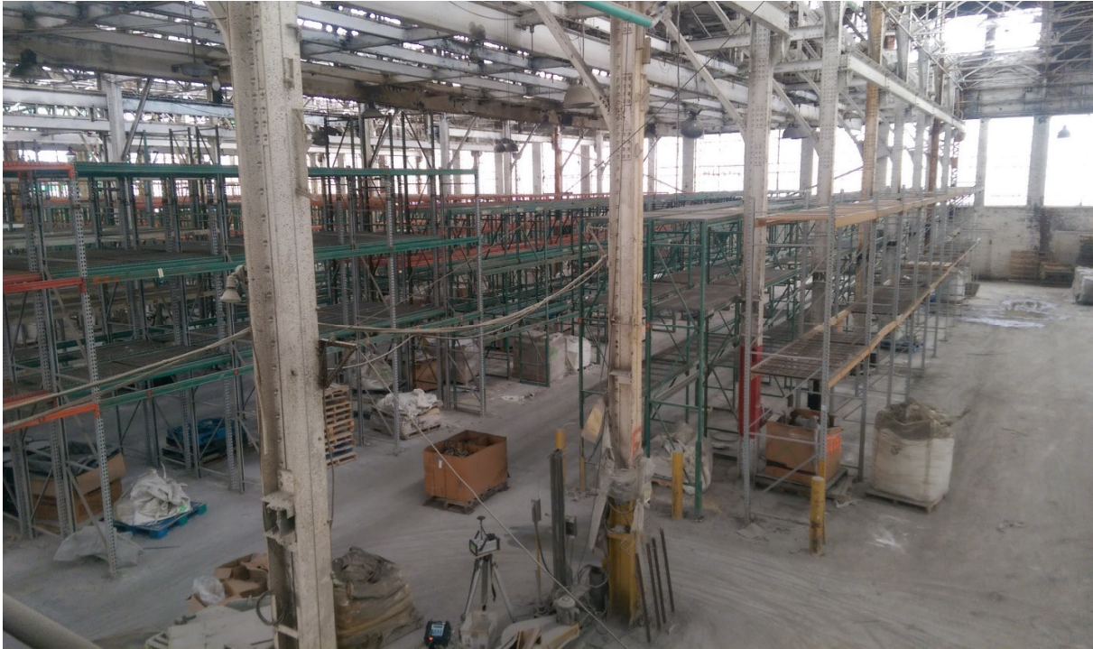
Photograph 56: View of Warehouse A after removal and cleanup activities.
