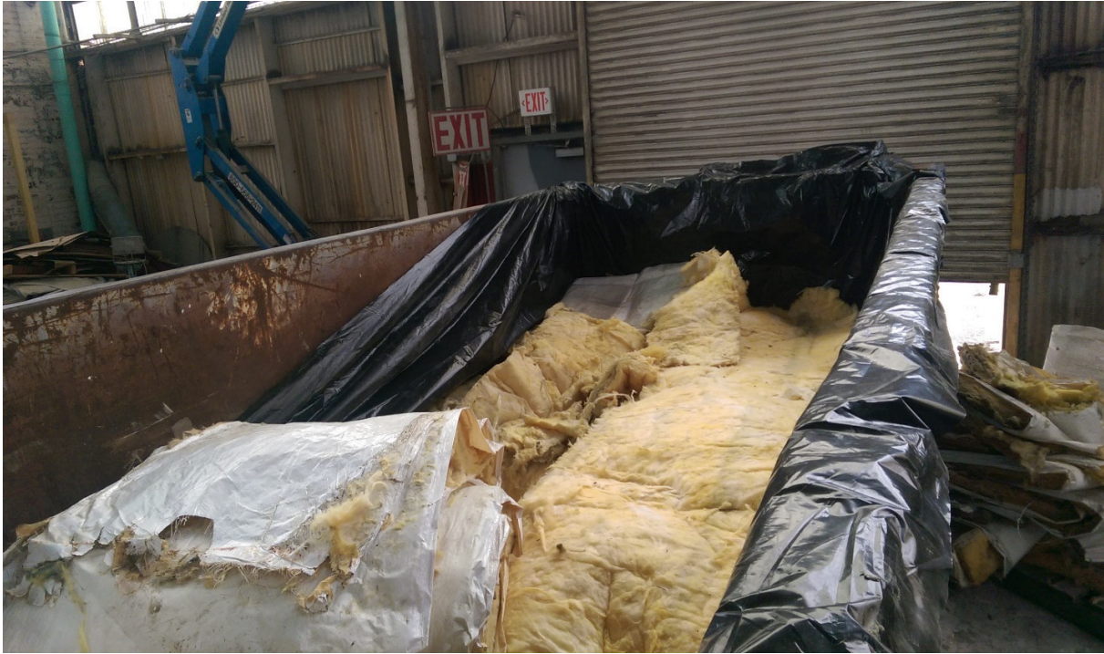
Photograph 69: View of insulation being consolidated in a lined dumpster for disposal.
