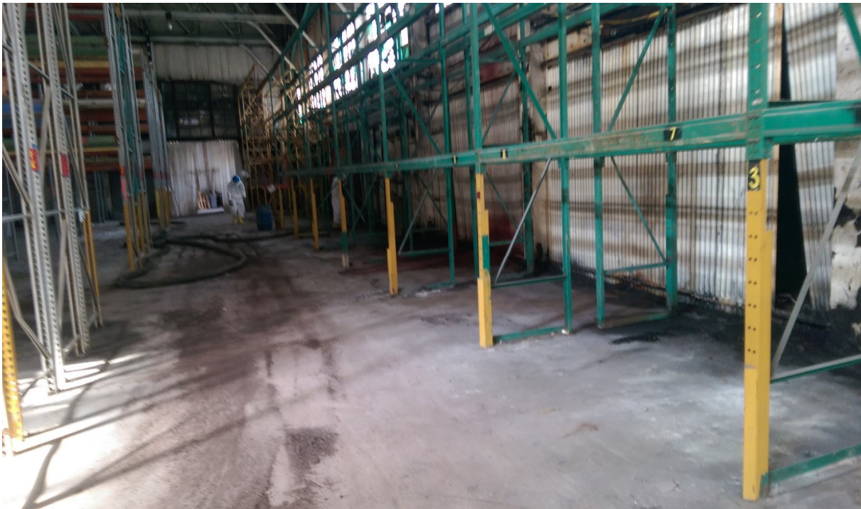
Photograph 60: View of Hallway after removal and cleanup activities.
