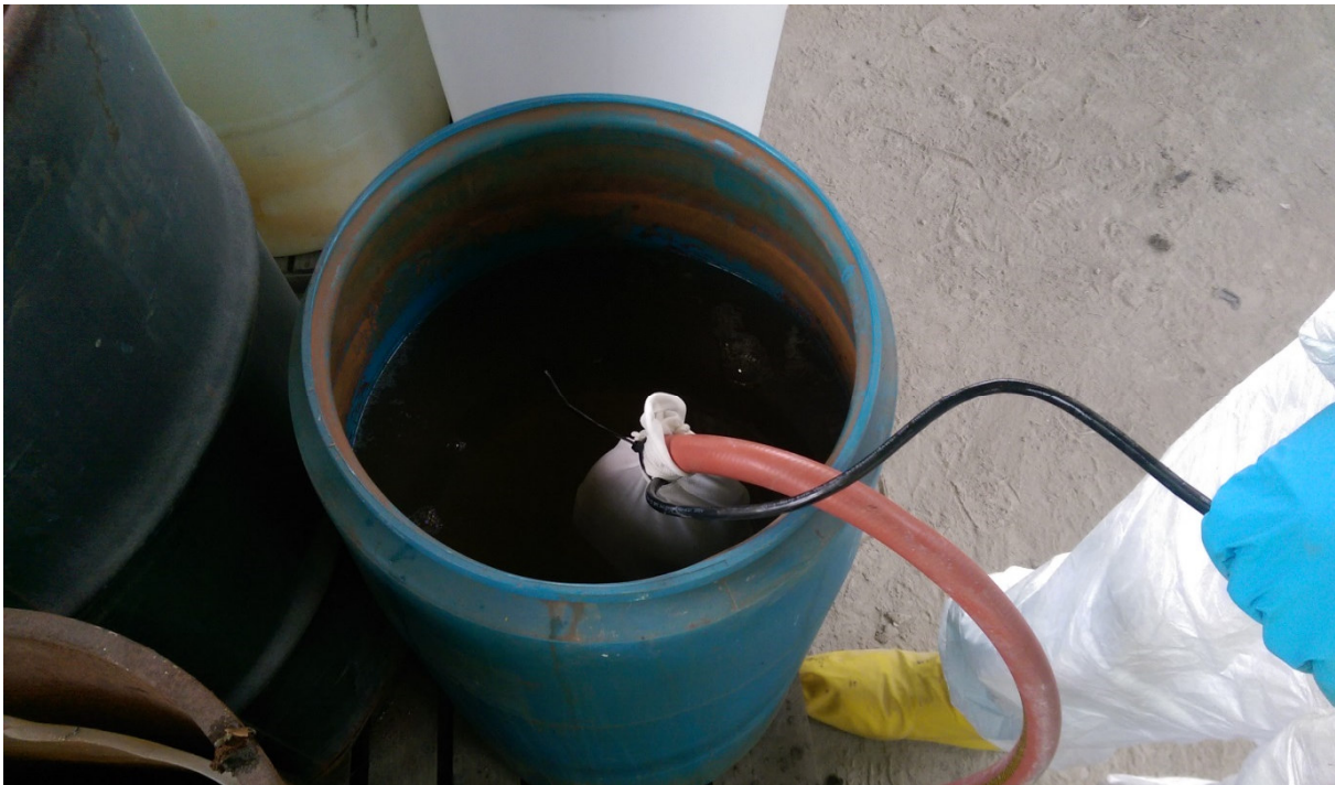
Photograph 42: View of water being pumped out of drum, prior to disposal of drums.
