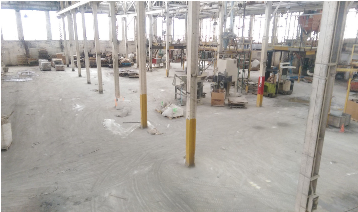
Photograph 58: View of Hallway after removal and cleanup activities.
