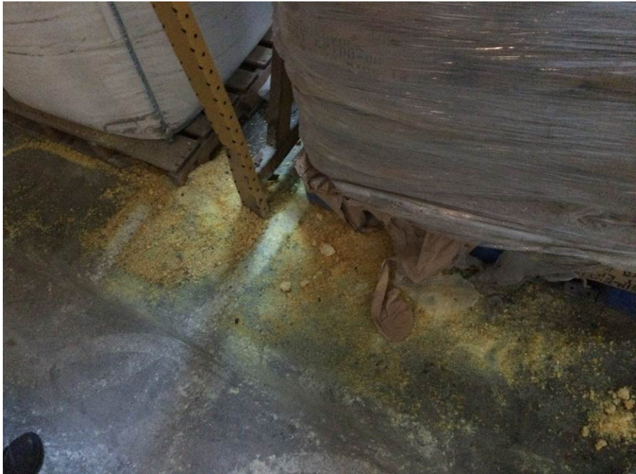
Photograph 12: View of spilled contents on floor found in Hallway.
