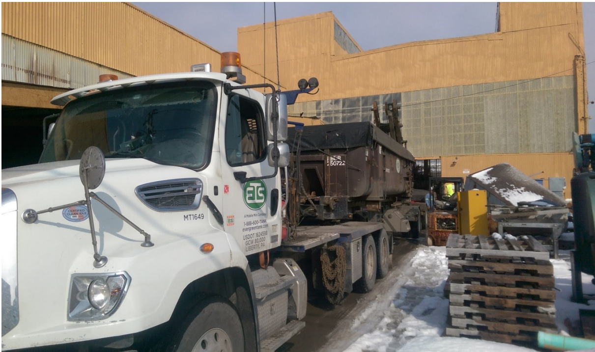
Photograph 38: View of grit material been transported offsite to a disposal facility.
