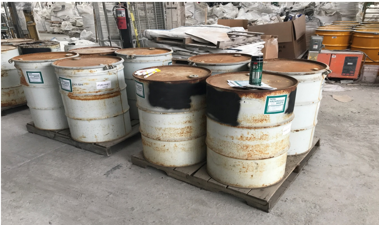
Photograph 28: View of drum staging and labeling prior to loading in truck for disposal.
