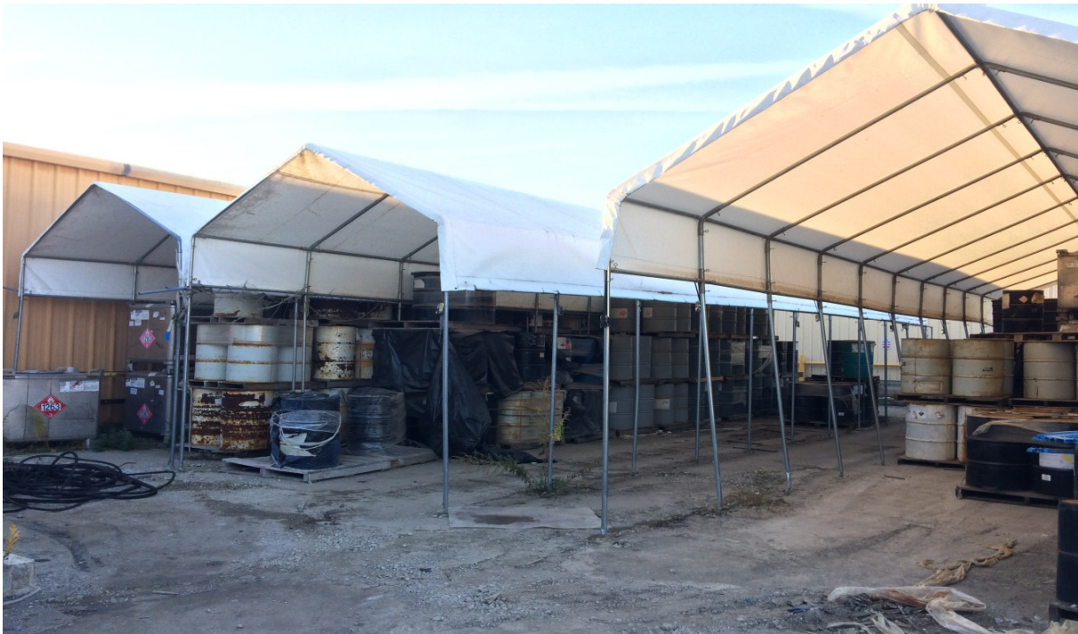
Photograph 12: View of material stored outside, between Warehouse C and Drum Room
