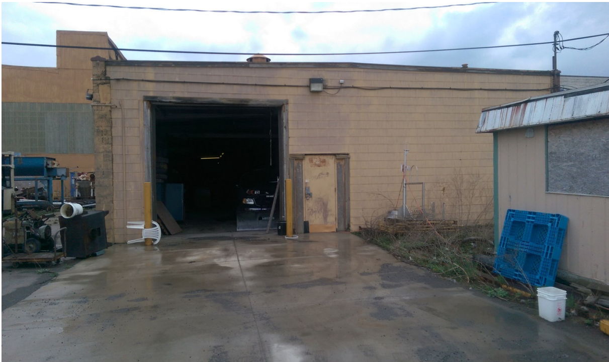
Photograph 2: View of Warehouse B.
