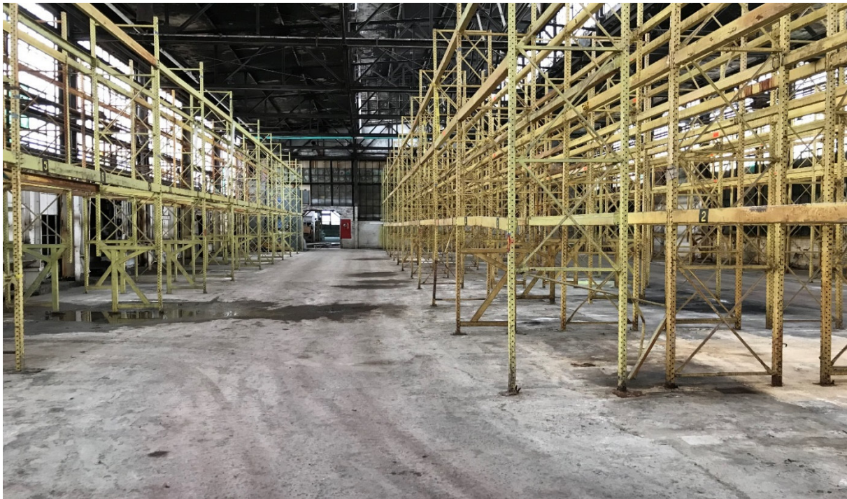
Photograph 64: View of Pigeon Room after removal and cleanup activities.
