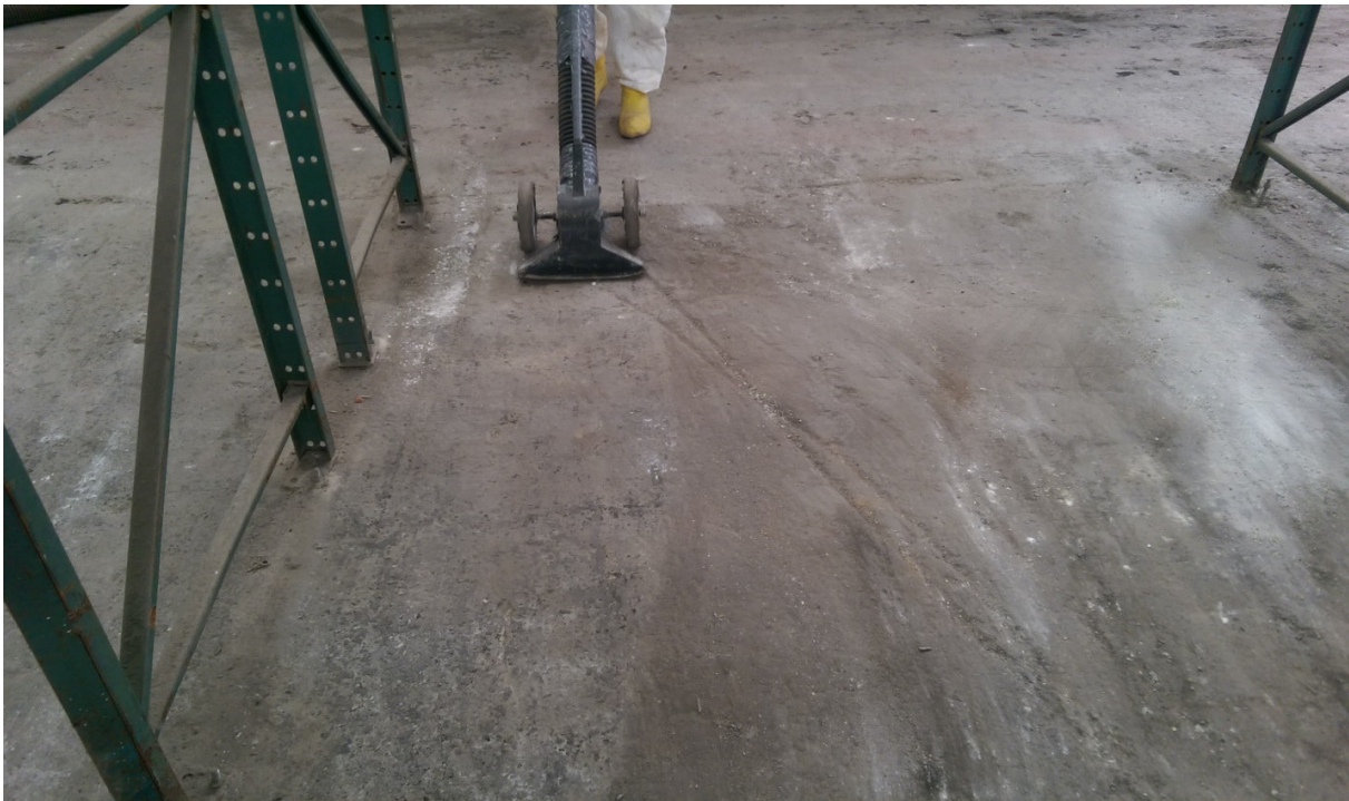
Photograph 74: View of GES crew vacumming floor in Warehouse A.
