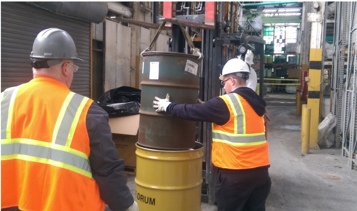
Photograph 16: View of drums been overpacked prior to loading by Veolia on behalf of BASF with the assistance of GES.
