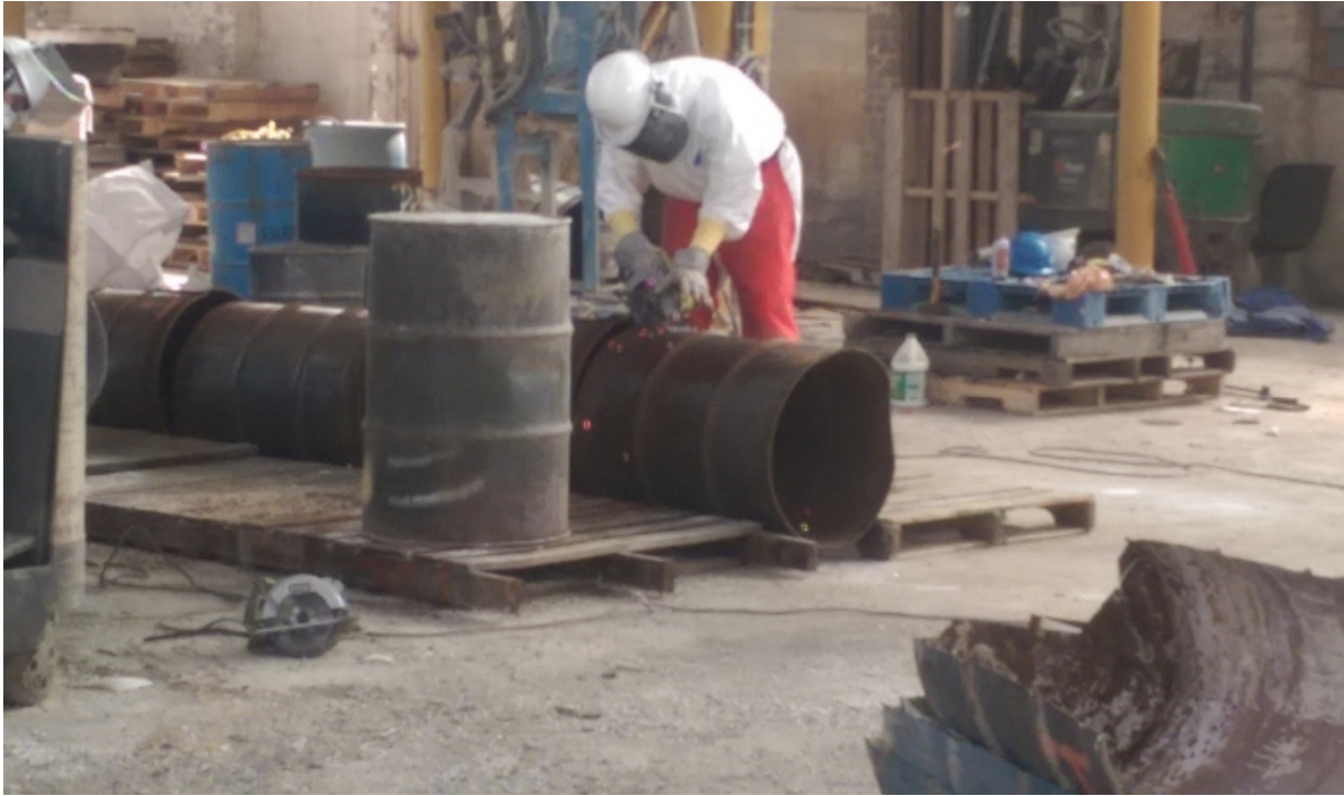
Photograph 33: View of metal drums been cut prior to disposal.
