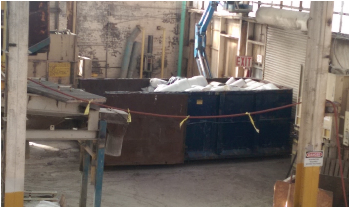
Photograph 34: View of dumpster staged for cut drums and totes for disposal.
