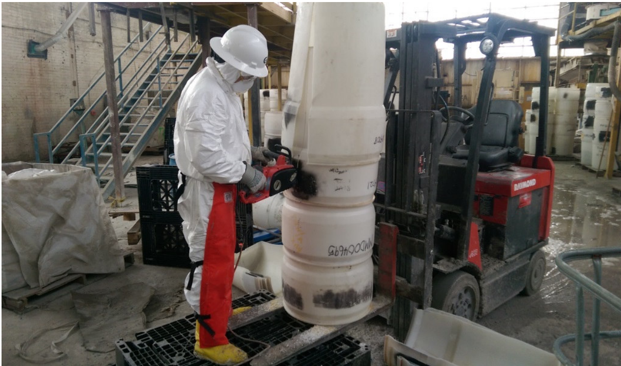
Photograph 30: View of poly drums been cut prior to disposal.
