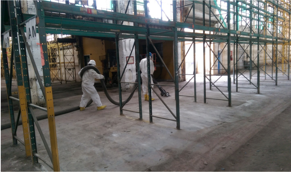
Photograph 73: View of GES crew vacumming floor in Warehouse A.
