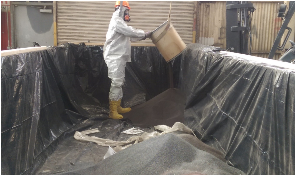
Photograph 36: View of grit material being consolidated in lined dumpster staged in Warehouse A for disposal. Disposal facility specified that the grit material should not be containerized.
