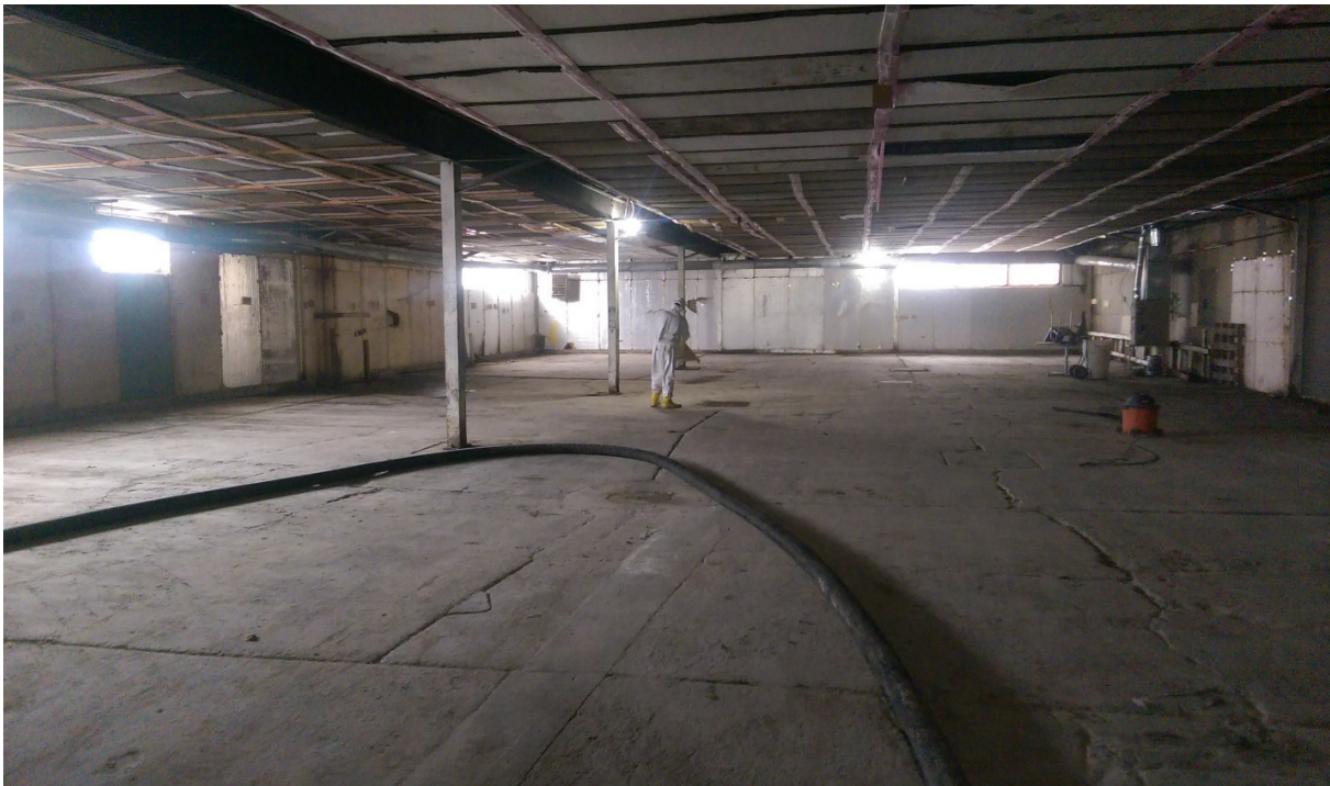
Photograph 68: View of Tote Room after removal and cleanup activities.
