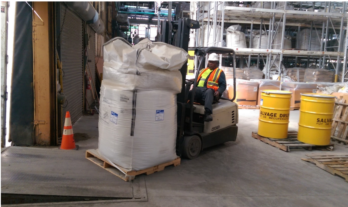
Photograph 18: View of material being loaded on truck for disposal by Veolia on behalf of BASF.
