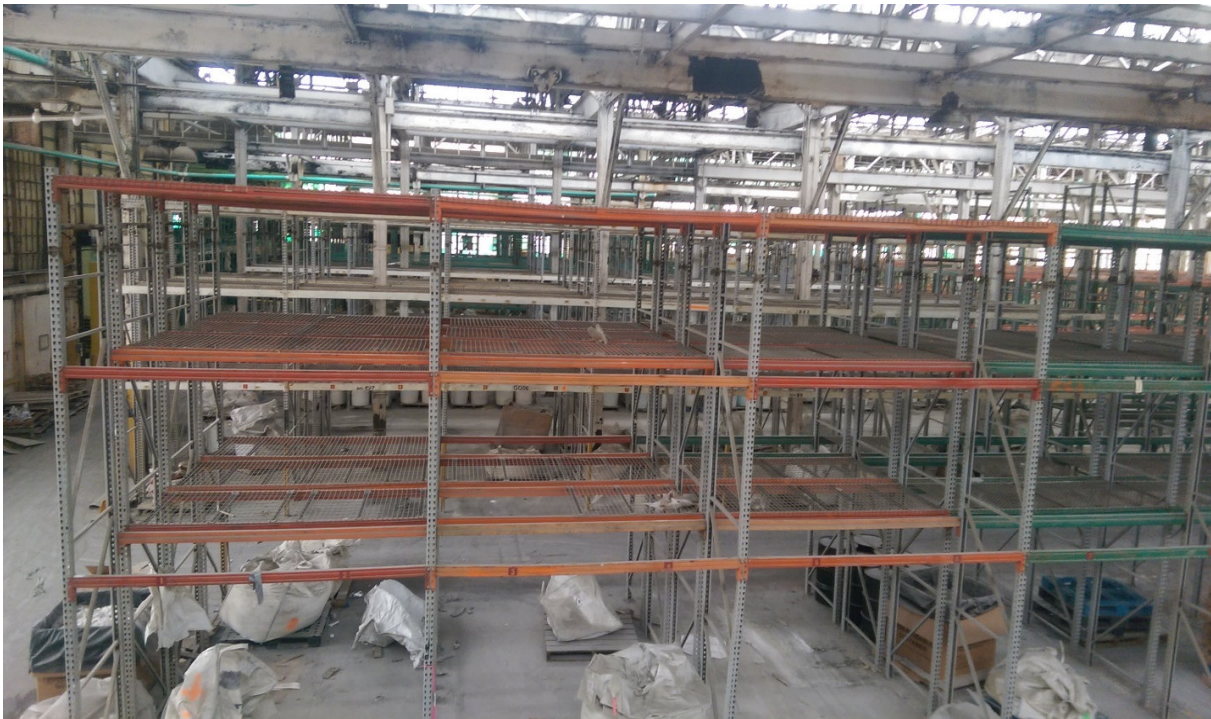
Photograph 62: View of Warehouse A after removal and cleanup activities.
