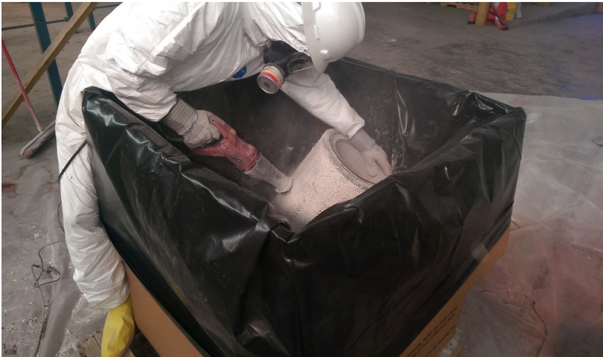
Photograph 40: View of used filters in Warehouse D being cut to pieces for disposal.
