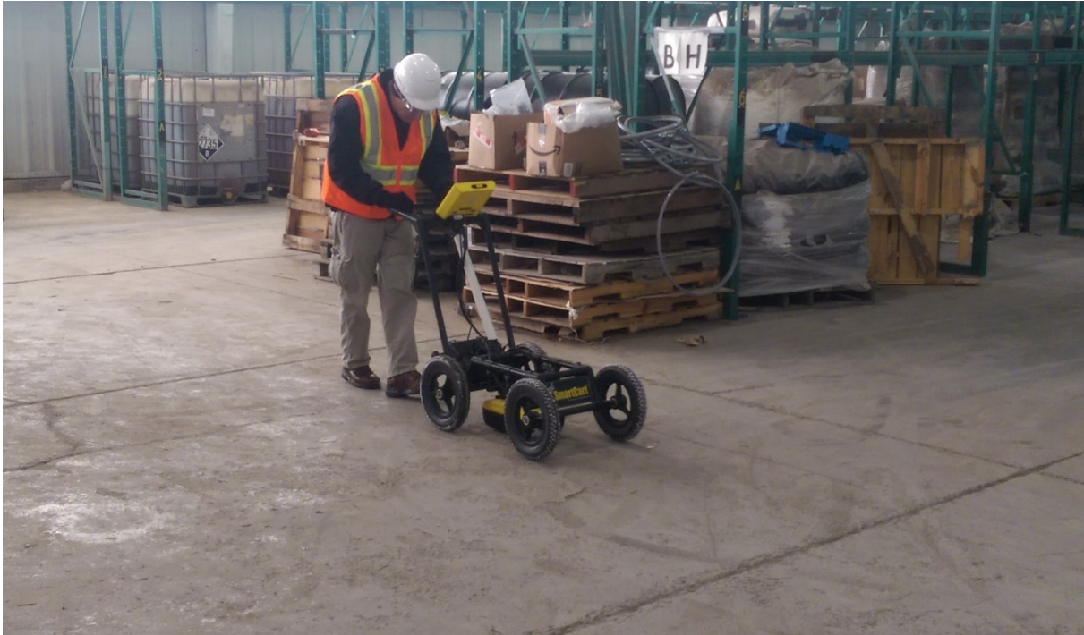
Photograph 53: View of Ground Penetrating Radar (GPR) being setup for use.
