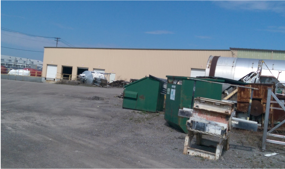
Photograph 3: View of Warehouse C.
