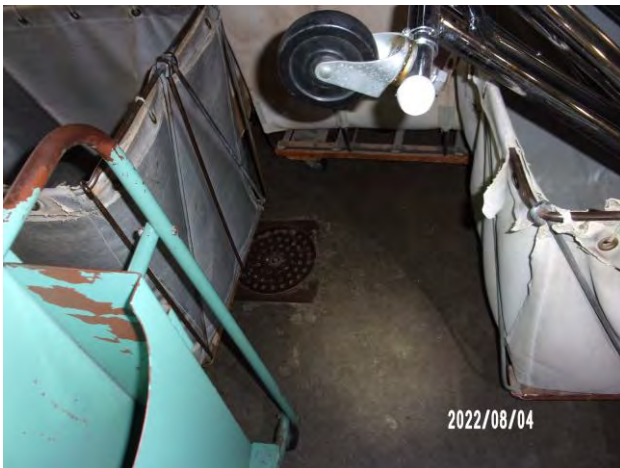
11. Floor drain in the center of the dry cleaning room with staining.
