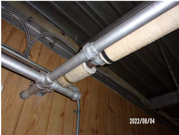
15. View of suspected asbestos wrapped piping.
