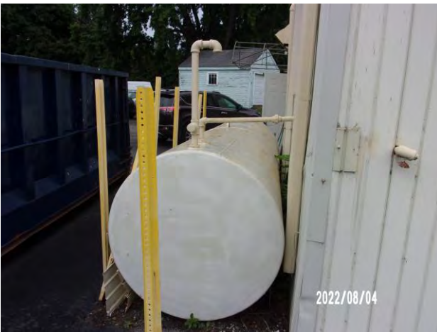
5. View of 1,000-gallon mineral spirits AST located at the rear of the building.
