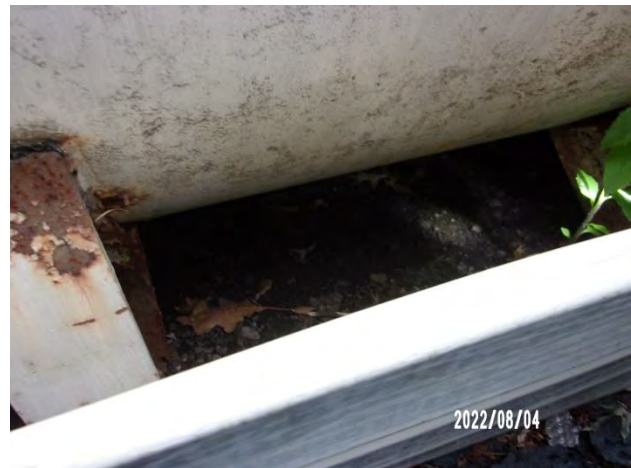
6. View of limited stained soil underneath the AST at the rear of the building
