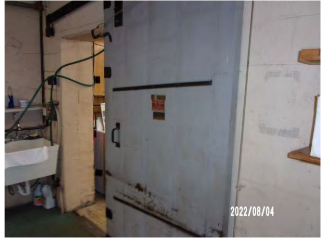
14. View of the fireproof doors in the steam press area.
