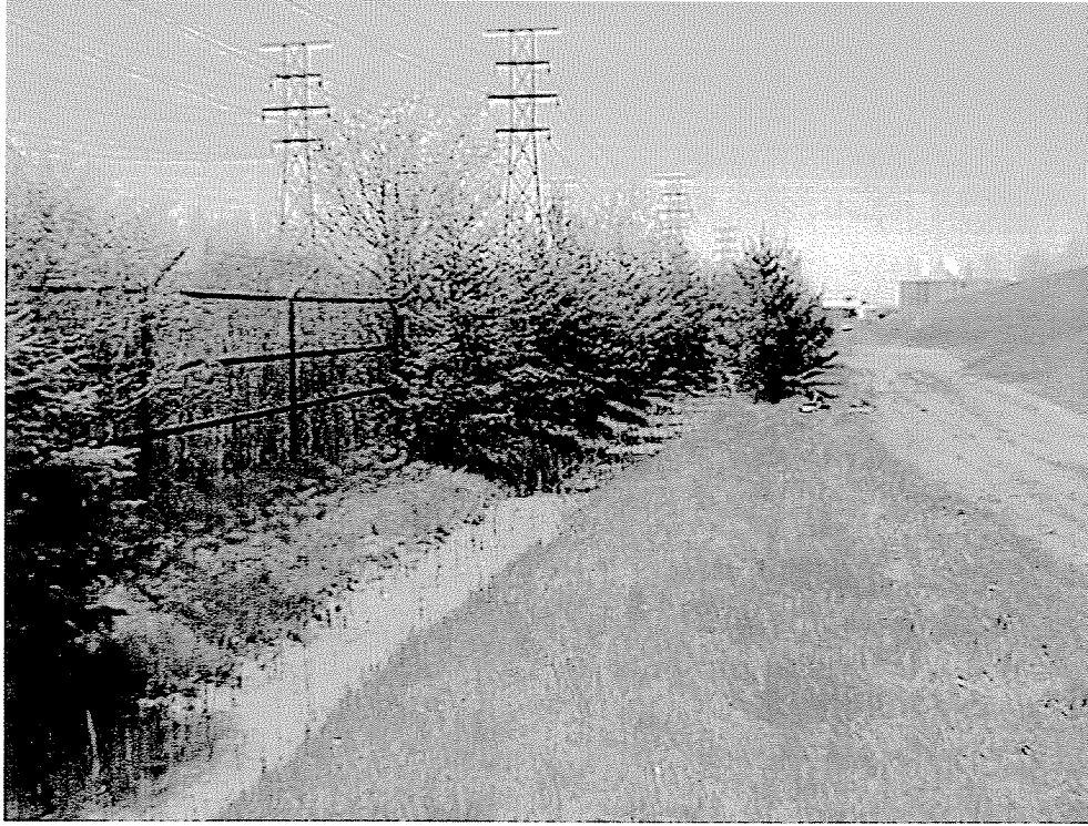
Photo 23. View west along drainage swale at south fence line on AIRCO property.
