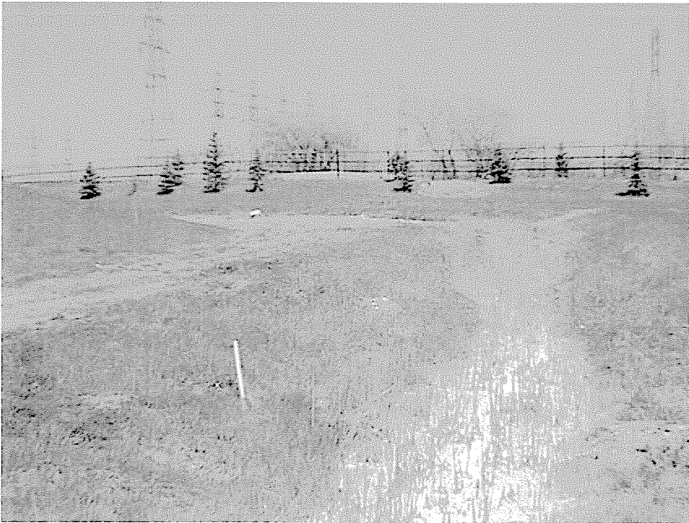
Photo 24. View east along drainage swale at south fence line on AIRCO property.
