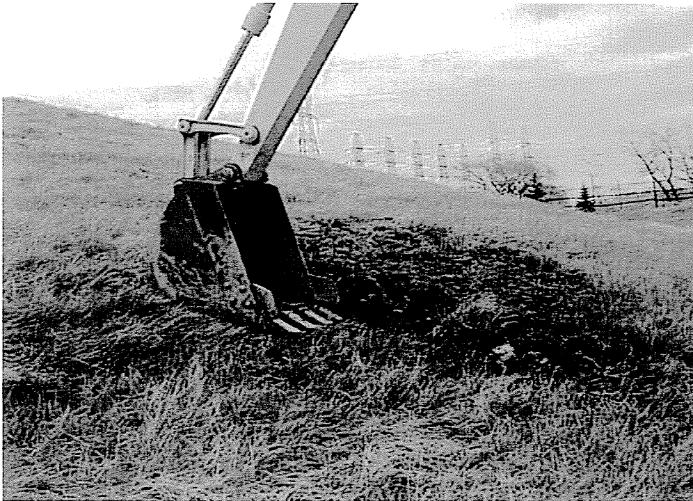
TP-01 in the southern sloped area previously capped.
